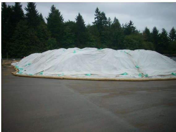
Photo #11: Non-contaminated reusable native backfill.
