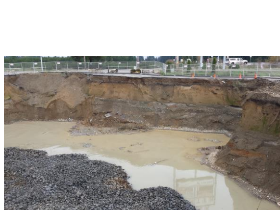
Photo #12: Quarry spall base being spread to northeast.
