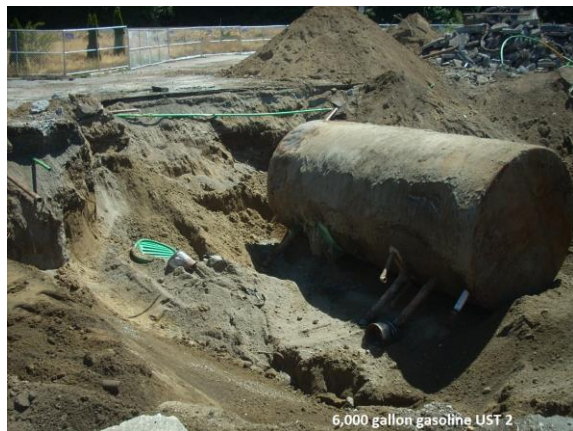
Photo #4: Initial groundbreaking for UST removal.
