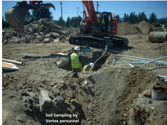
Photo #8: Product line trench soil sampling.
