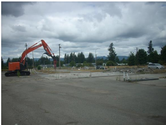
Photo #3: Demolition of concrete slab on grade structures.
