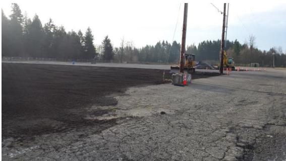
Photo #29: Finished to grade looking Southeast
