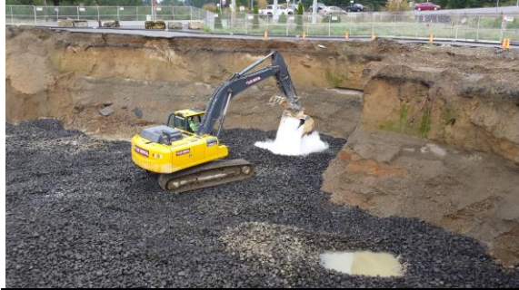
Photo #14: Introduction of Regenesis products into groundwater. Observed bubbling.
