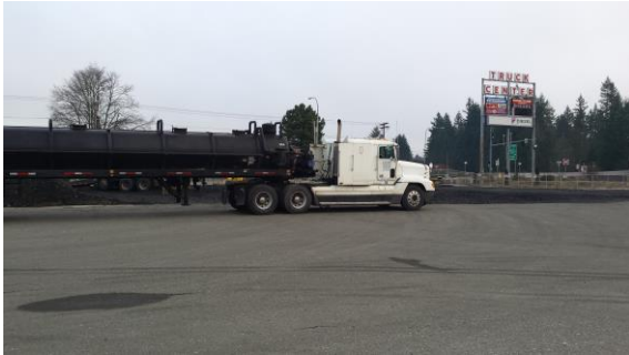
Photo #25: Final cleaning of baker tanks and carbon vessels
