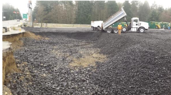
Photo #24: Spalls to top of water table at 8 feet bgs
