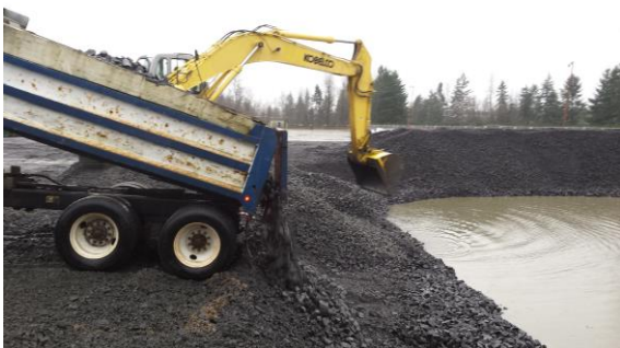
Photo #23: Backfilling into water with spalls. Water at 8 feet bgs
