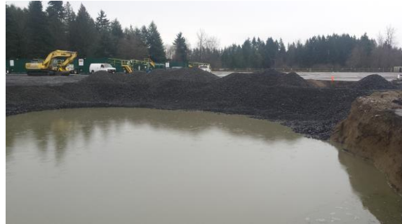
Photo #80: Looking southeast at high water table
