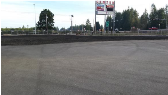
Photo #27: Looking Northeast finish grade
