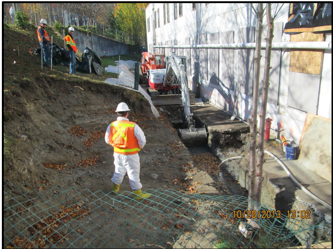
Photograph 1-8: Removal of storm drain line and soil south of Building 27.
