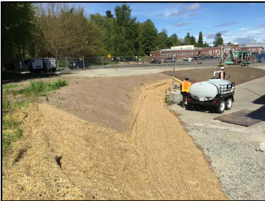
Photograph 1-16: Installation of straw matting over reseeded slopes near Building 27.
