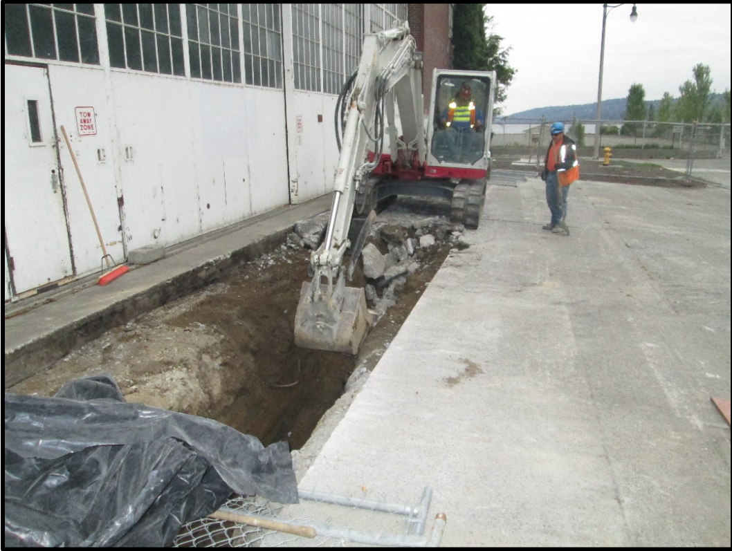
Photograph 1-3: Excavation of Building 2 sink drain line.
