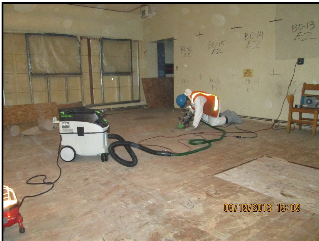
Photograph 1-2: Floor remediation in Building 2 former 1941 Instrument Shop area.
