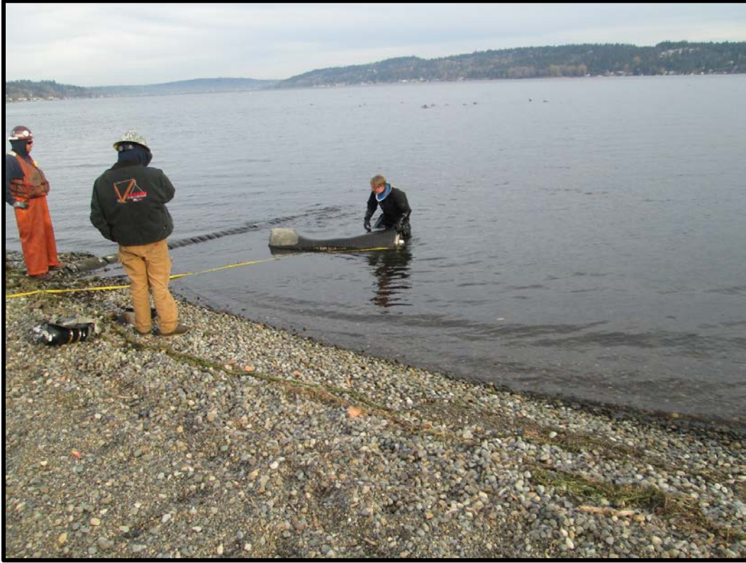
Photograph 1-13: Installation of plug in storm drain outfall to Lake Washington.
