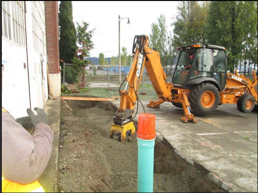
Photograph 1-4: Backfill/compaction of Building 2 sink drain line trench.
