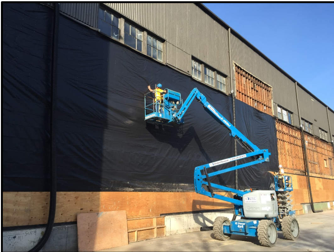
Photograph 1-14: Vapor barrier installation on Building 27 common wall.
