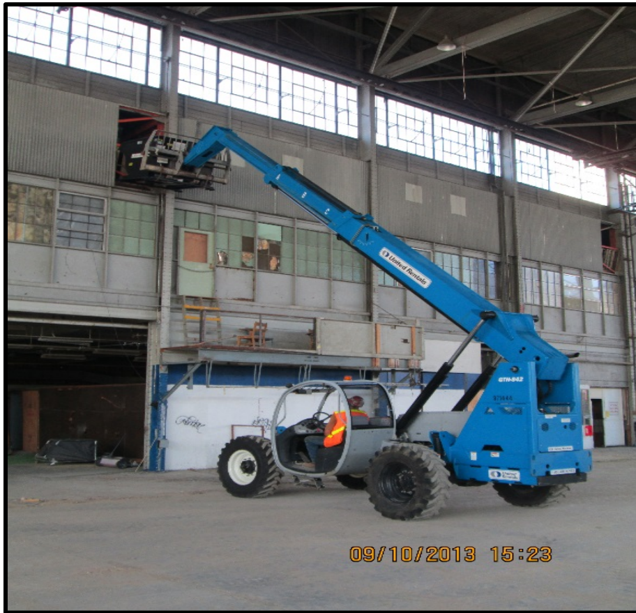
Photograph 1-1: Removing ventilation ducting from Building 2 attic space.
