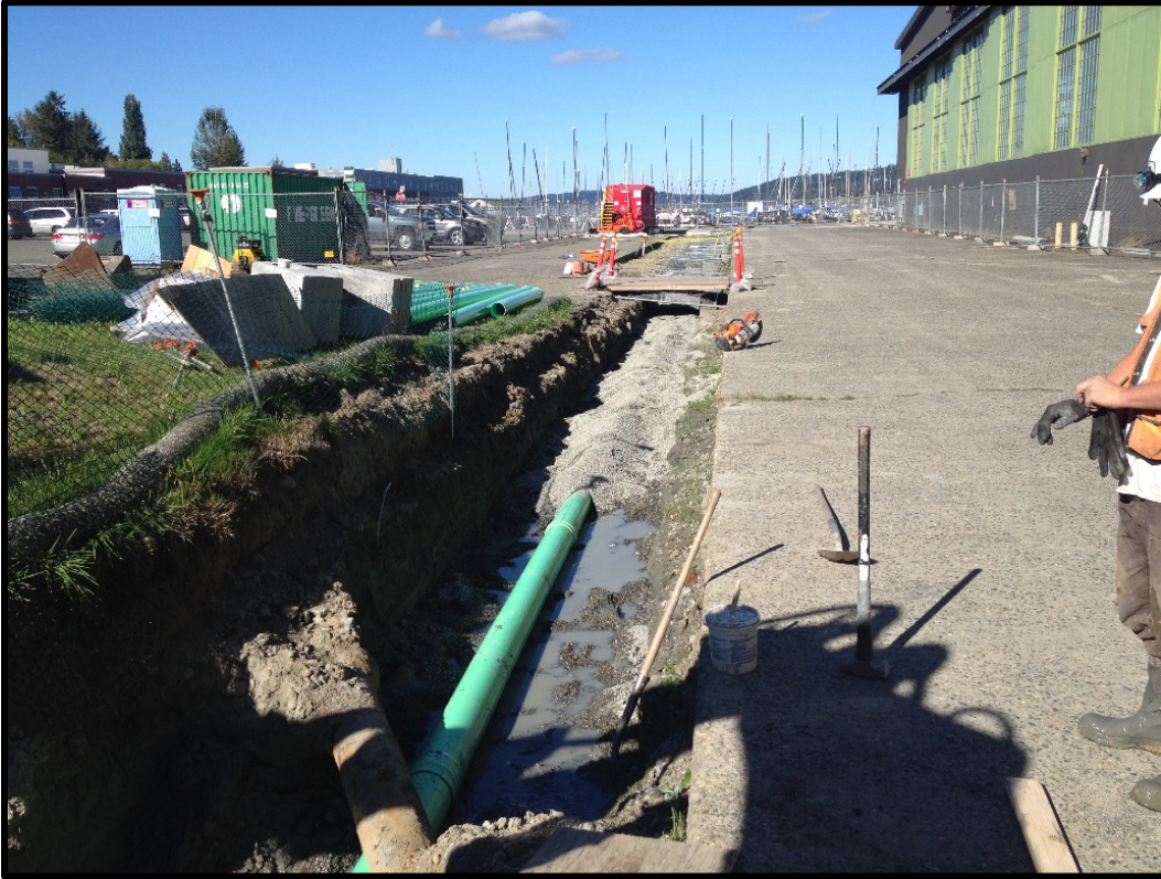
Photograph 1-11: Installation of new storm drain pipe from CB-5 to CB-8.
