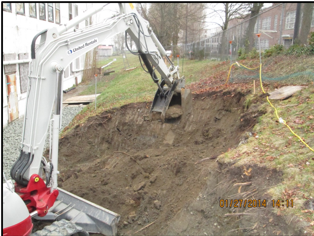
Photograph 1-6: Excavation of HS-07 south of Building 27.
