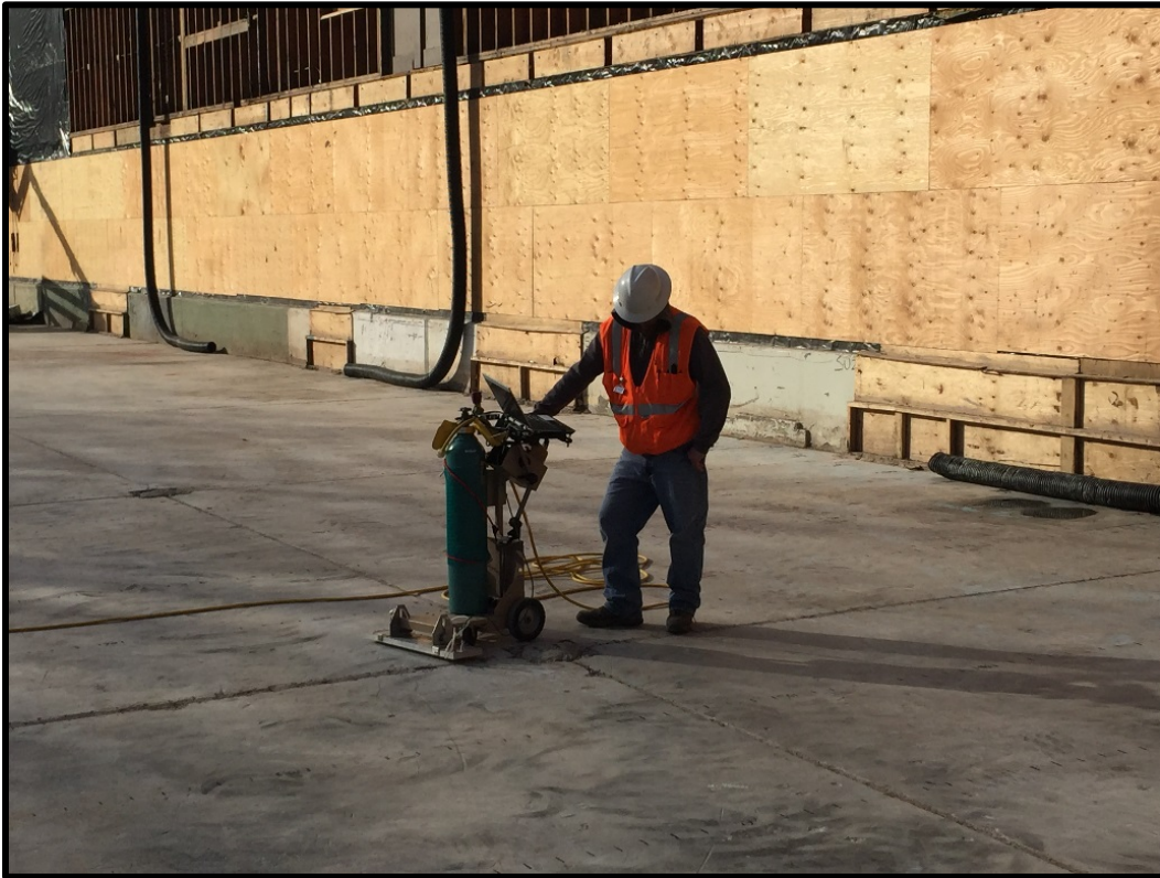
Photograph 1-15: Performing alpha/beta scan survey of the former South Shed concrete slab.
