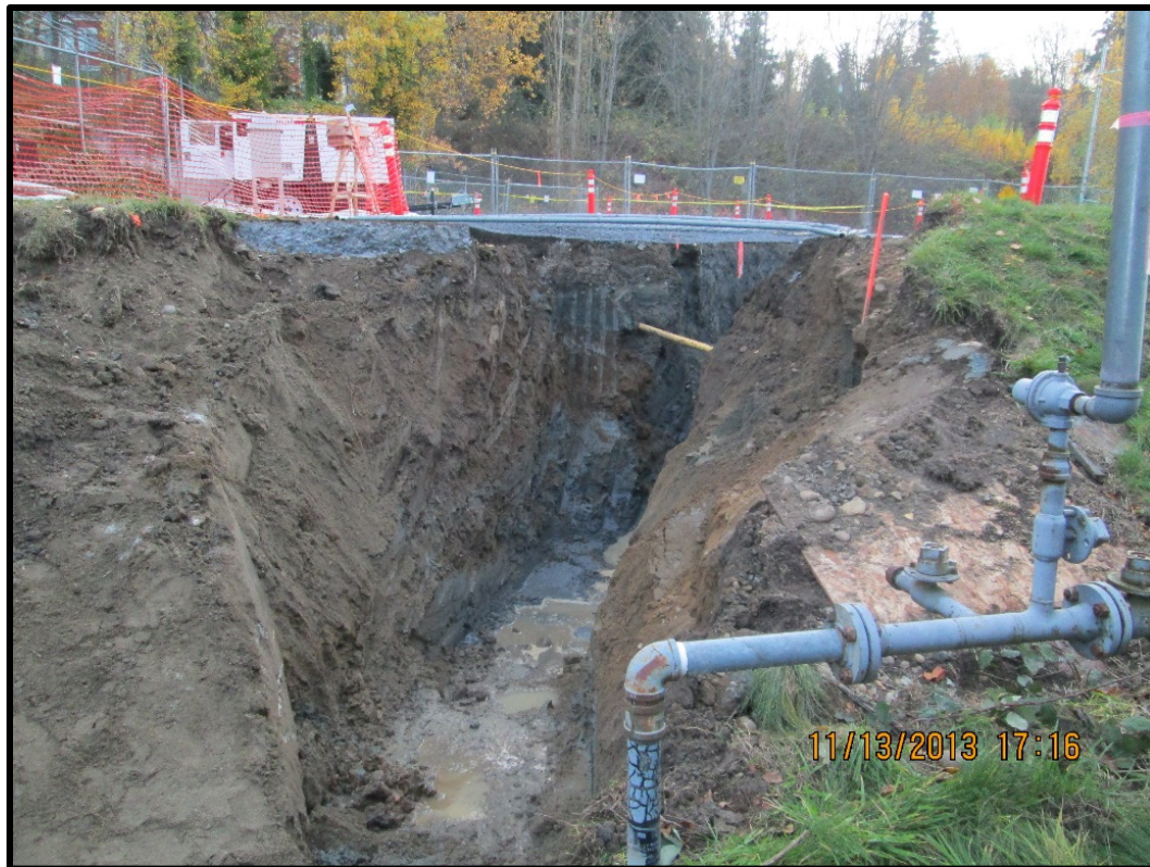
Photograph 1-10: Storm drain line to MH-141 excavation west of Building 27.
