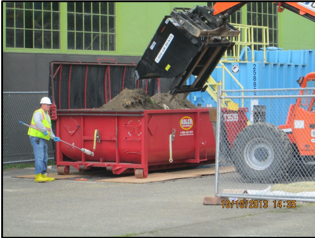
Photograph 1-9: Placement of low-level radioactive soil into a disposal bin.
