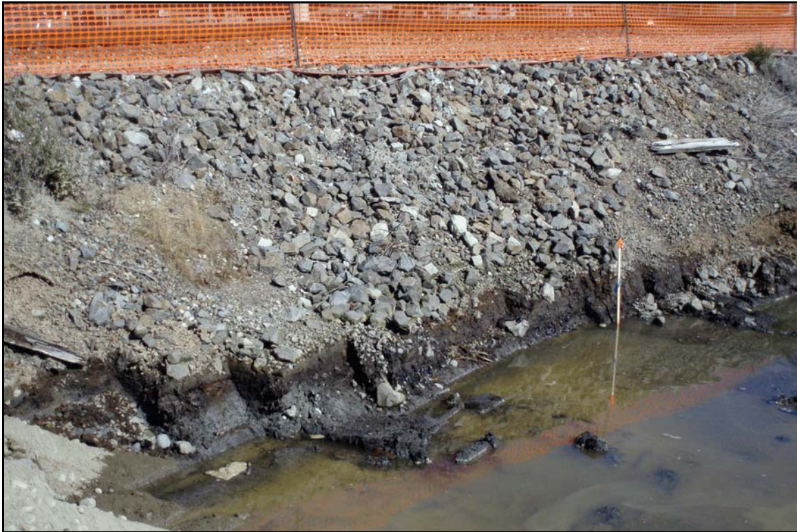
Figure 11. Close-up of excavated Willow Creek, depth at twelve feet below surface.
