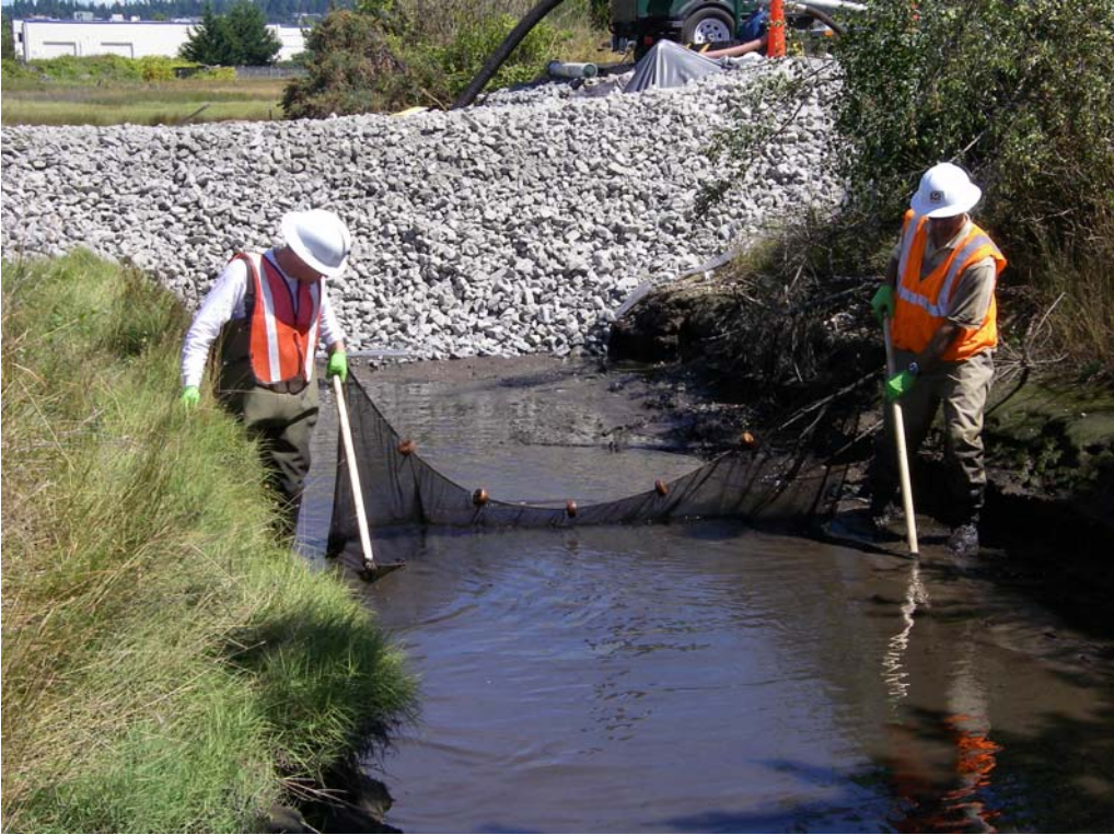
Coffer Dam and Seining
