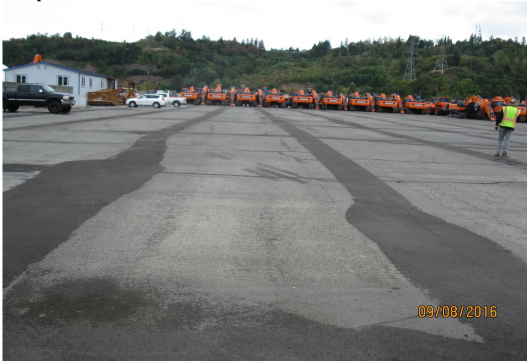
Photo 1: Cap Area - from the south
