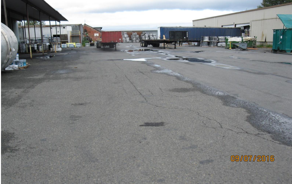
Photo 3: Storage Area and Asphalt Cap - from the north
