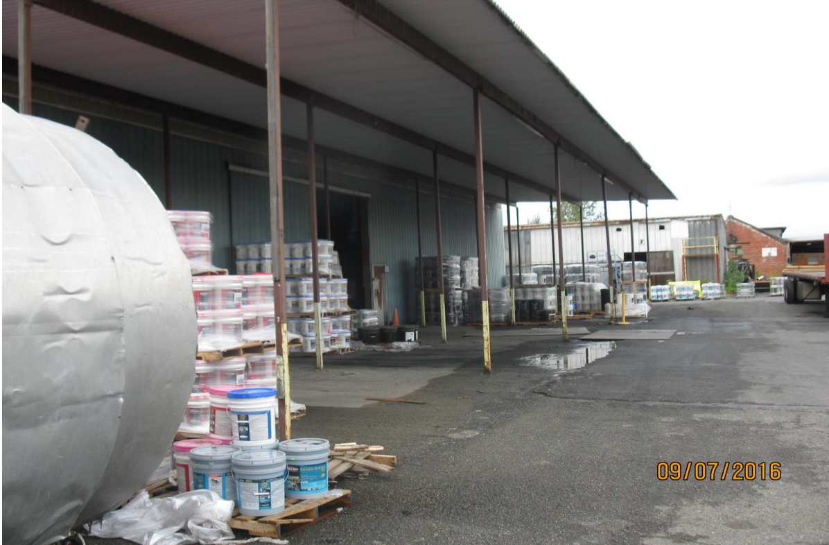
Photo 4: Former Storage Building and Asphalt/Concrete Cap – from the northeast
