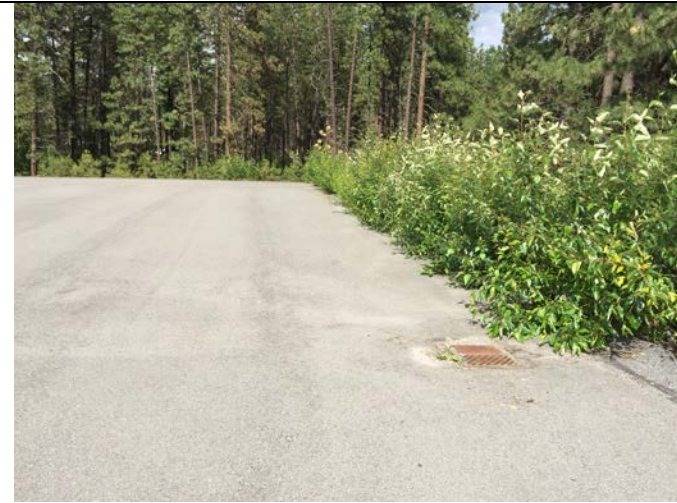
Photo 2: View looking east along southern edge of cap. Note vegetation growth along margin of asphalt cap.
