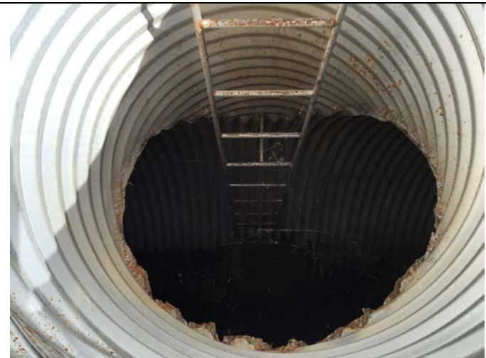
Photo 12: View inside vault at cap.
