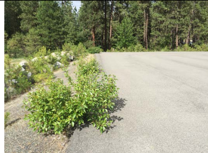
Photo 4: View looking east along northern edge of cap. Note vegetation growth along margin of asphalt cap.
