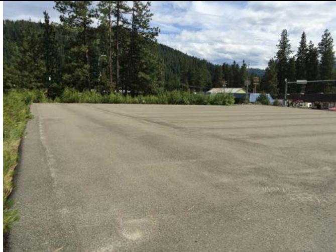
Photo 3: View looking south along eastern edge of cap. Note vegetation growth along margin of asphalt cap.
