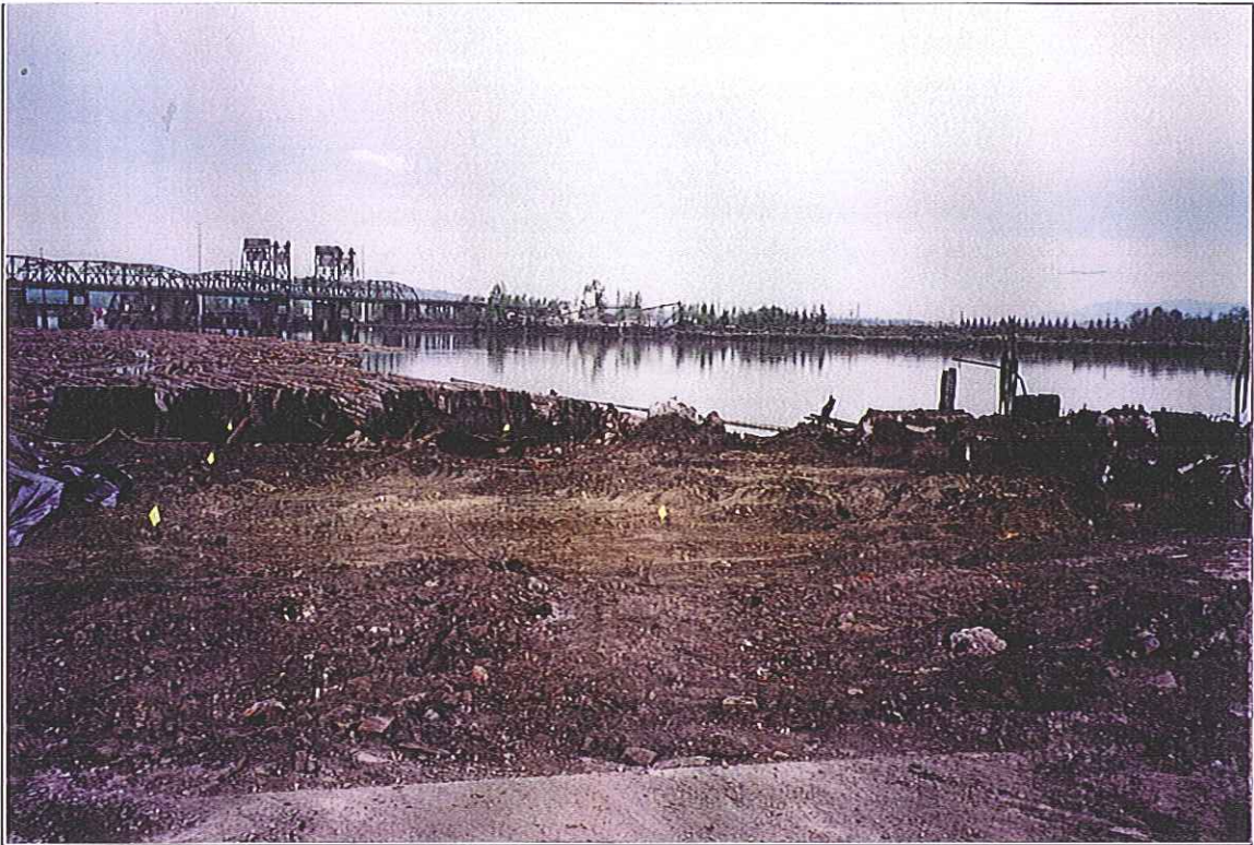
Area 7-2B Excavation Area (Looking North)
