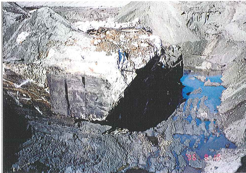
Area 7-1 Excavation Area Concrete Structure Removed (Looking East)
