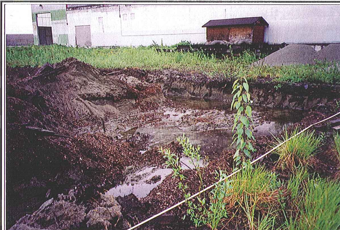
Area 10-4B Perimeter Trench (Looking Southeast)
