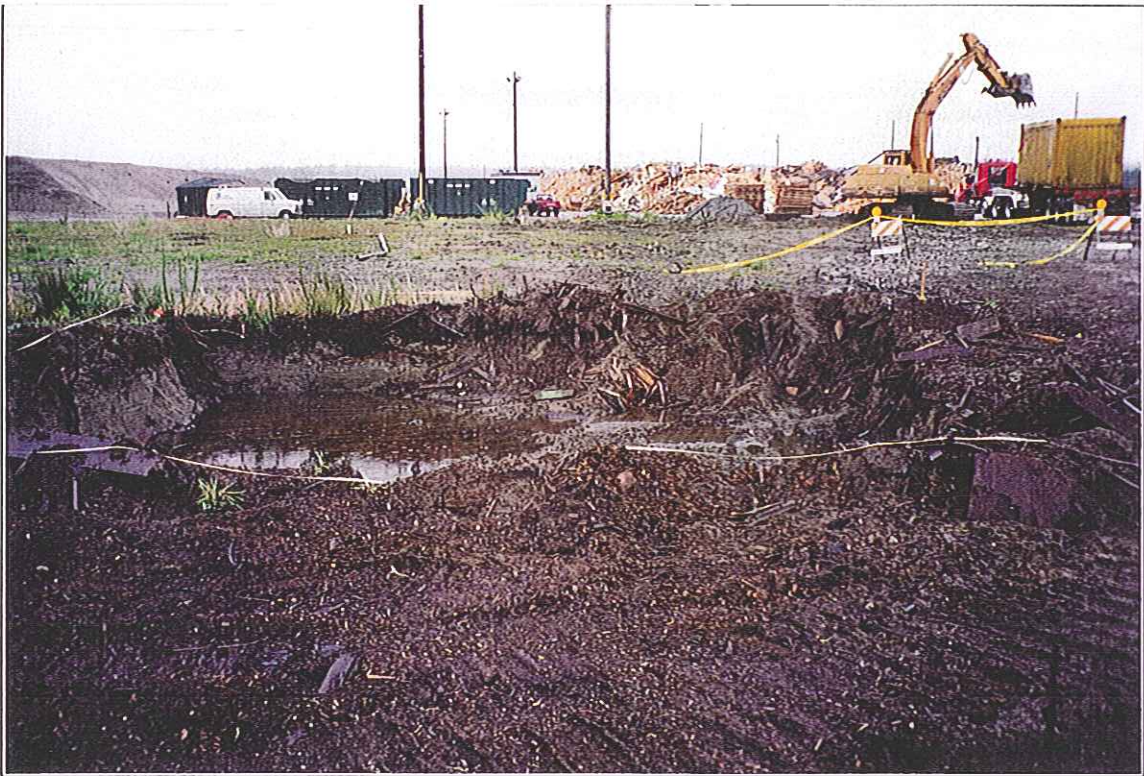
Area 10-4C Excavation Area (Looking East)
