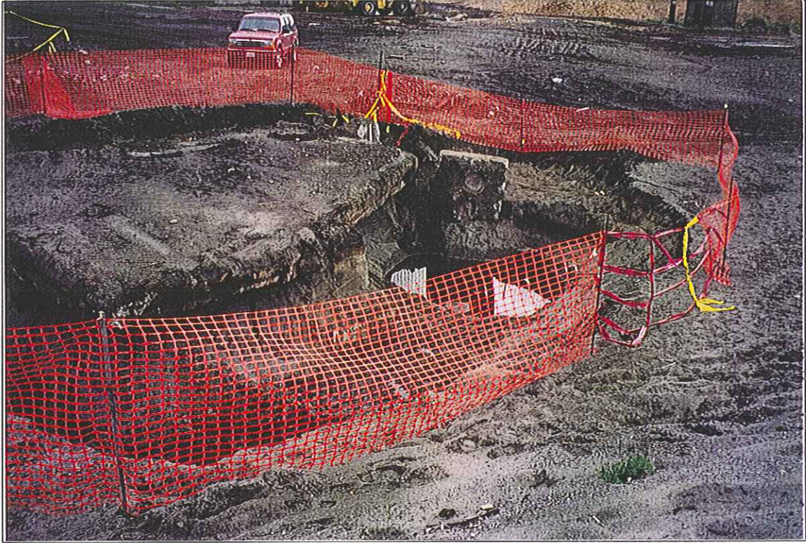
Area 8-1 Excavation Area (Looking Southwest)
