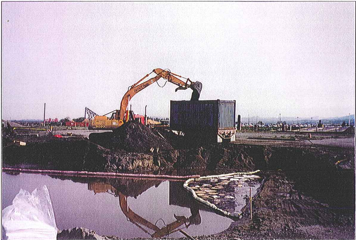
Area 8-3A During Excavation (Looking Northeast)
