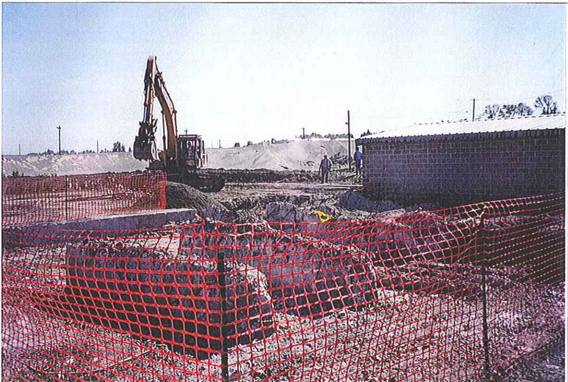
Area 7-2A Debris Removed to Concrete Slab (Looking South)
