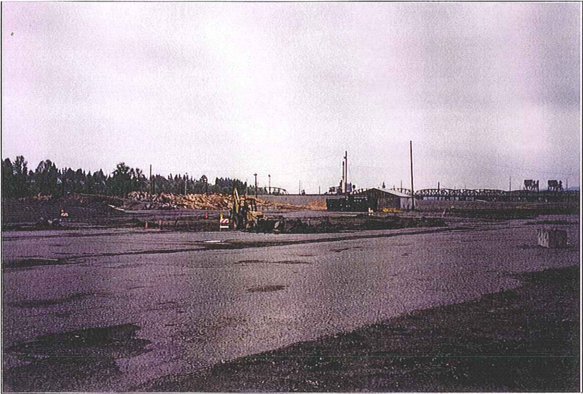
Area 8-3A Removing Asphalt Pavement (Looking Northwest)
