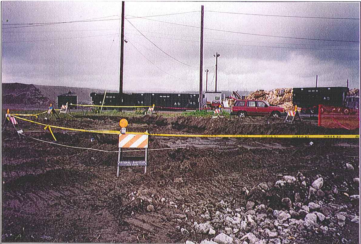
Area 10-3A Excavation Area (Looking East)
