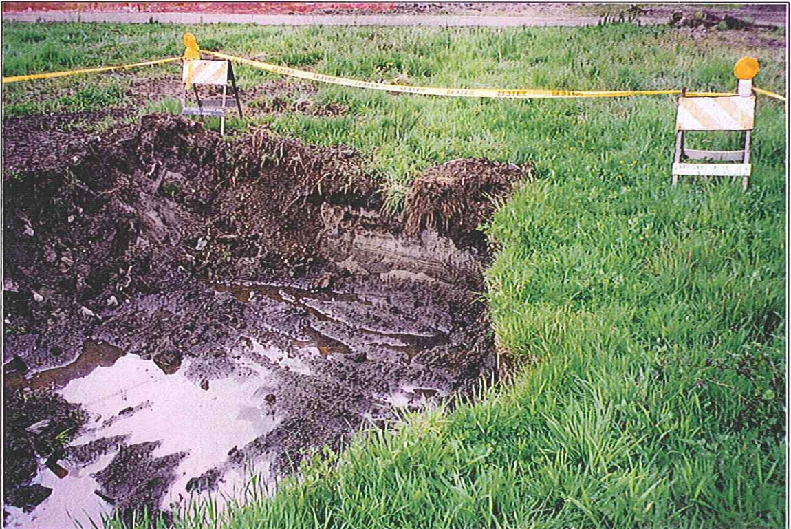
Area 10-3B Excavation Area (Looking East)
