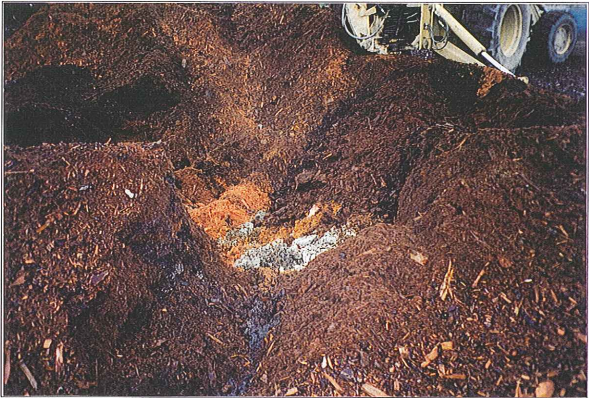
TP-16 Area Excavation to Lime Waste
