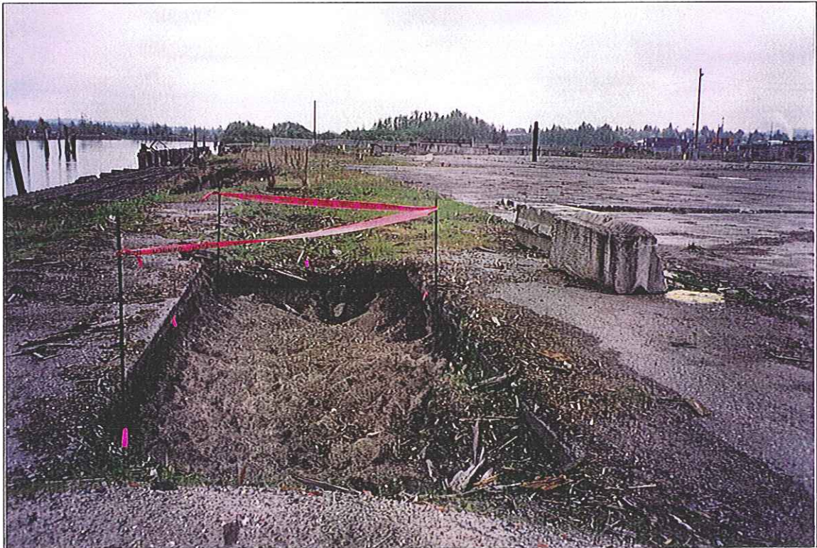
Area 8-4 Excavation Area (Looking East)
