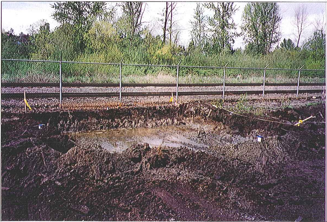
Area 10-4A Initial Excavation Area (Looking West)
