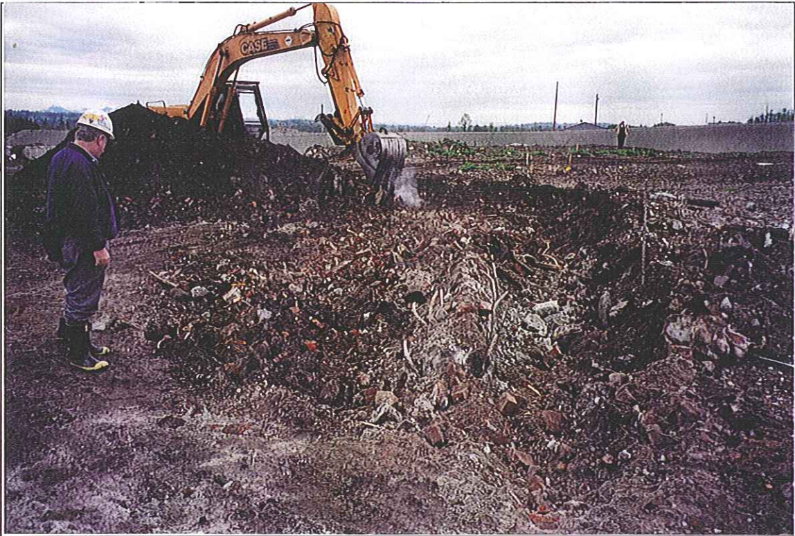
Area 7-2A Initial Stages of Debris Removal (Looking Southeast)
