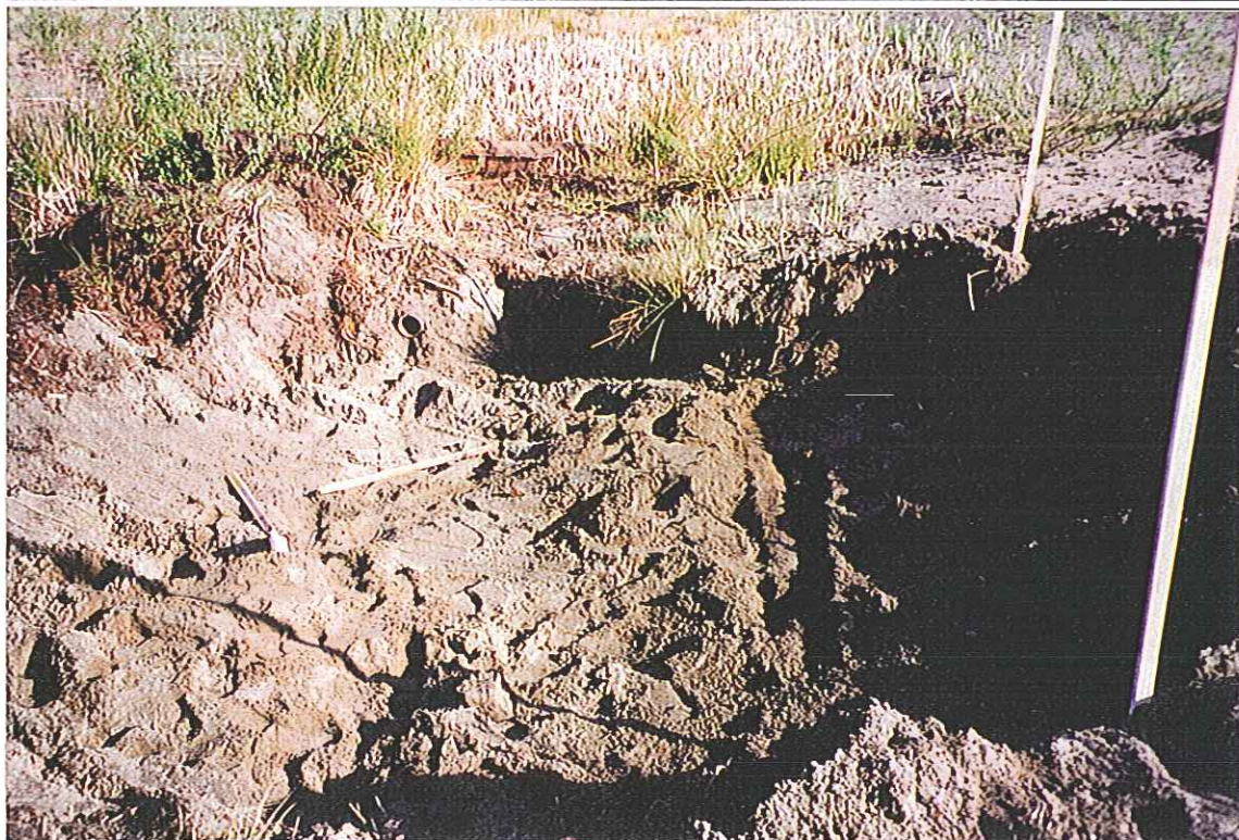
Area 10-1 During Excavation (Looking Northwest)
