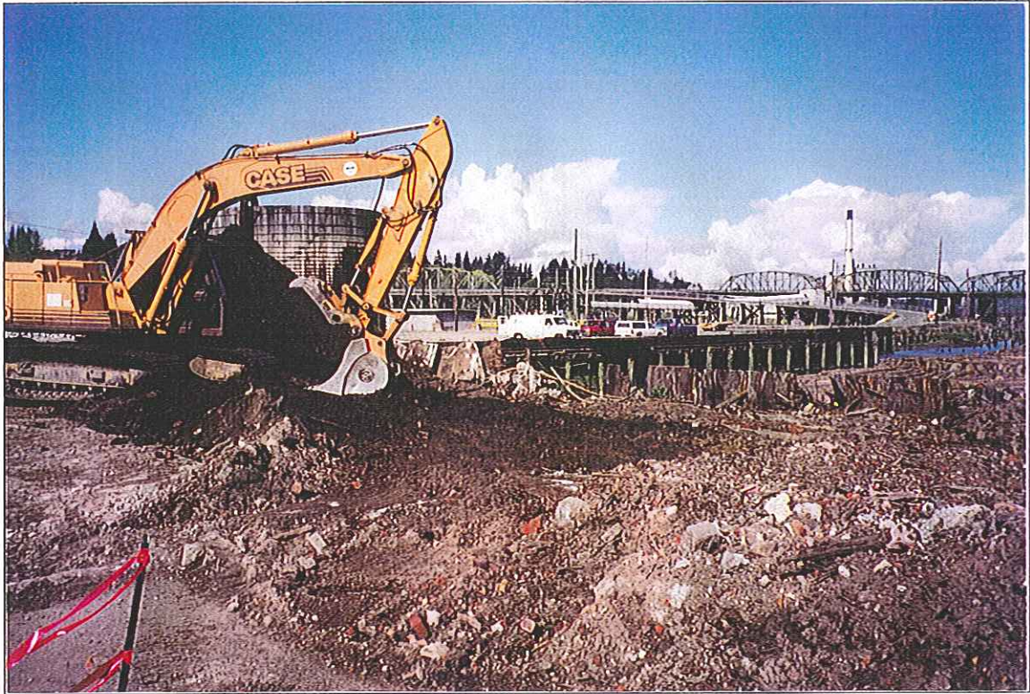
Area 7-2B During Excavation (Looking North)
