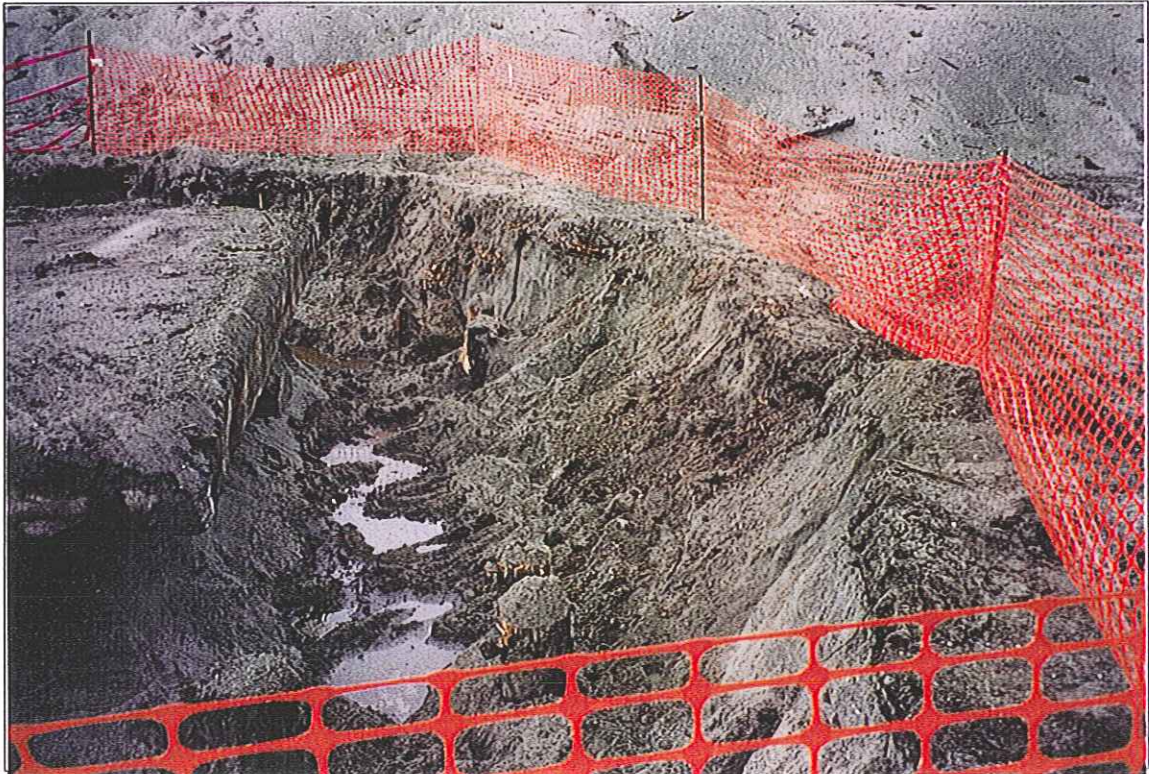
Area 8-1 Excavation Area (Looking Northwest)
