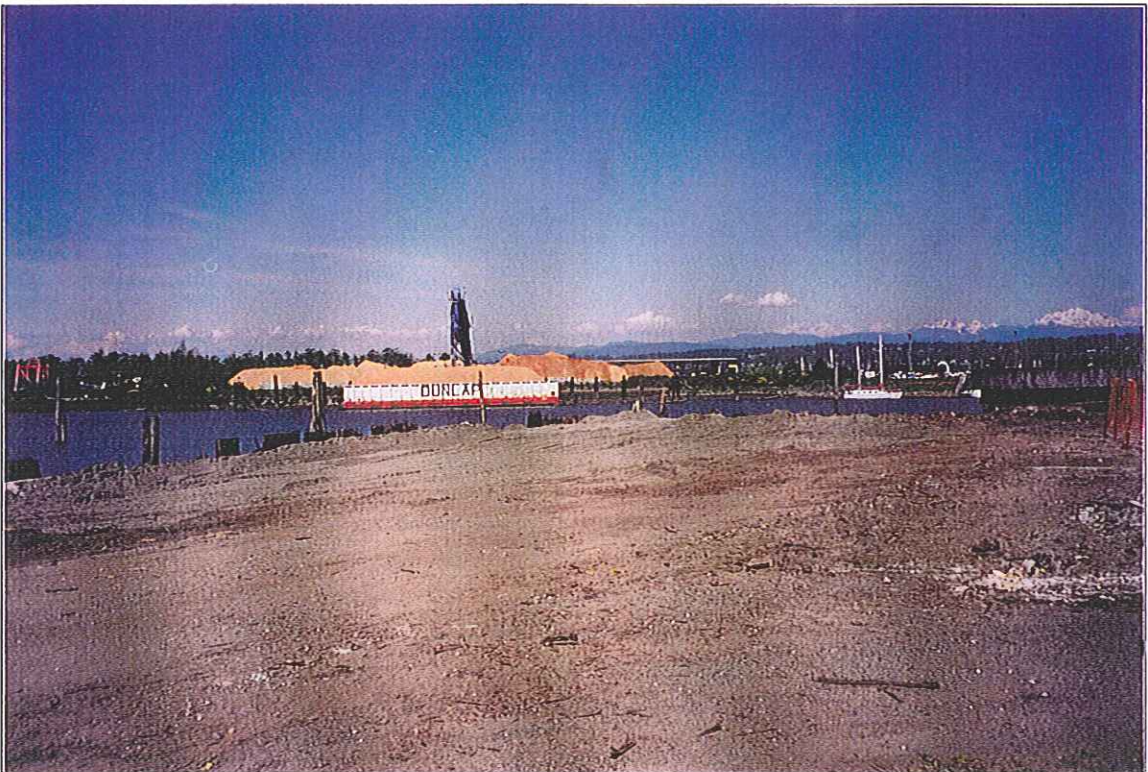
Area 7-2B Backfilled (Looking Northeast)
