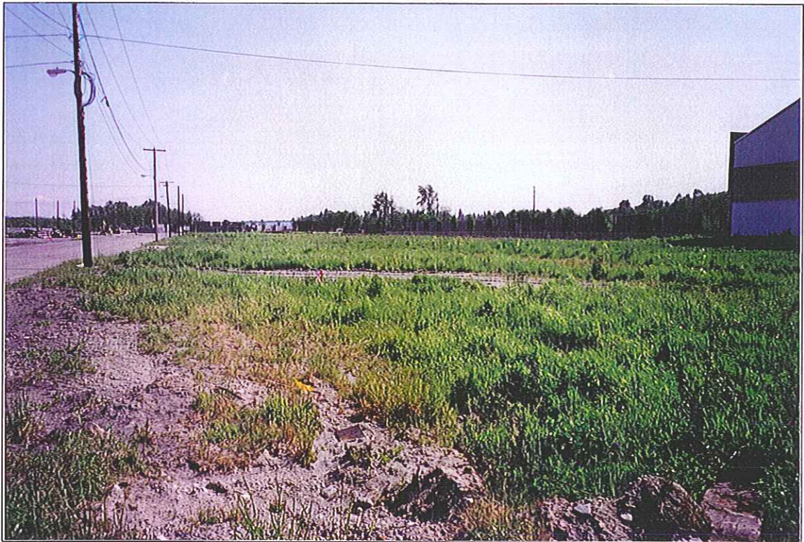
Portion of Area 10-3 Backfilled (Looking South)
