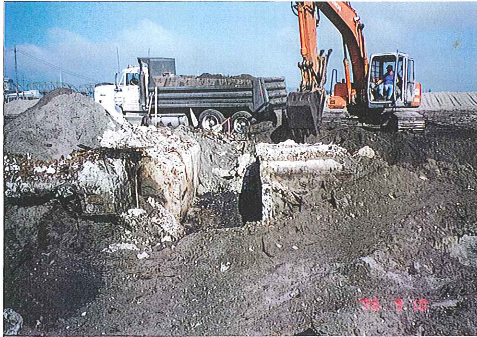
Area 7-1 During Excavation Showing Concrete Structure (Looking North)
