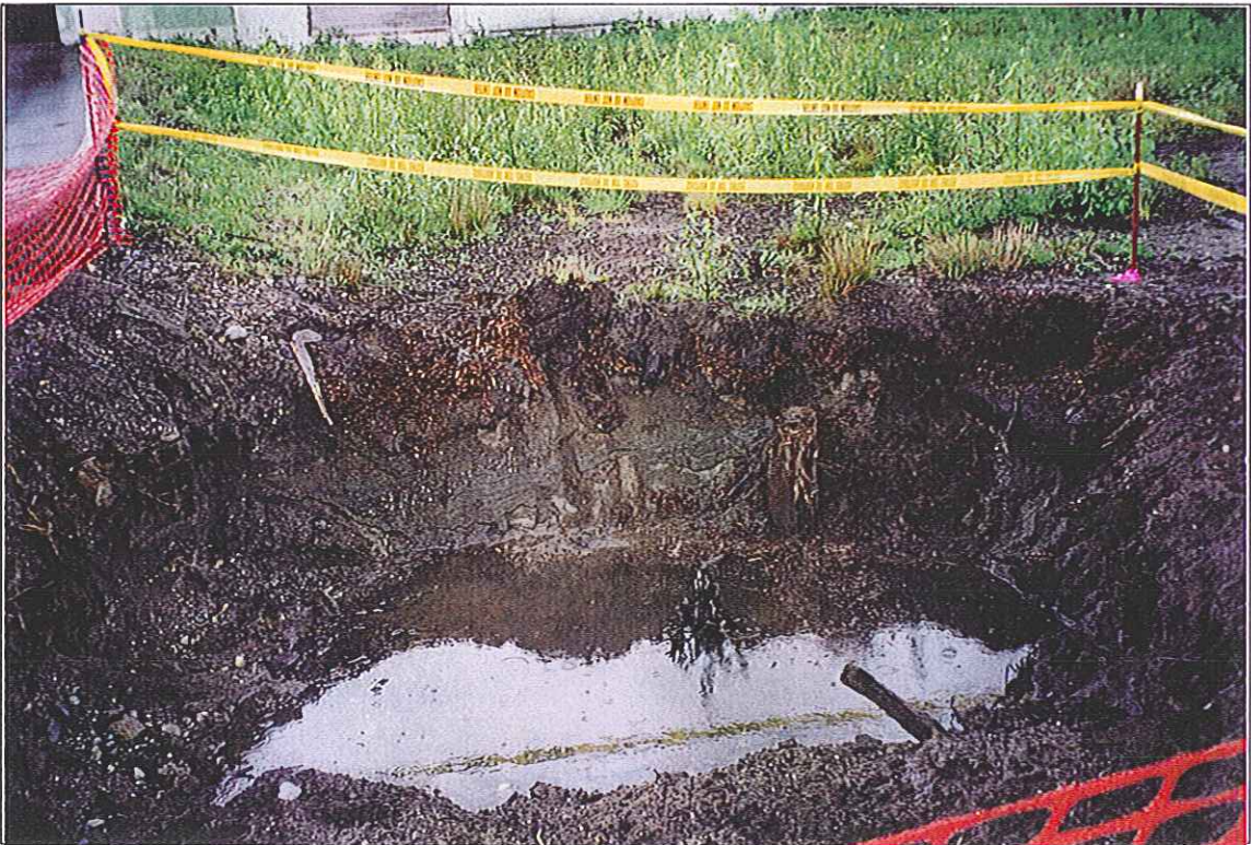
Area 10-4D Excavation Area (Looking South)
