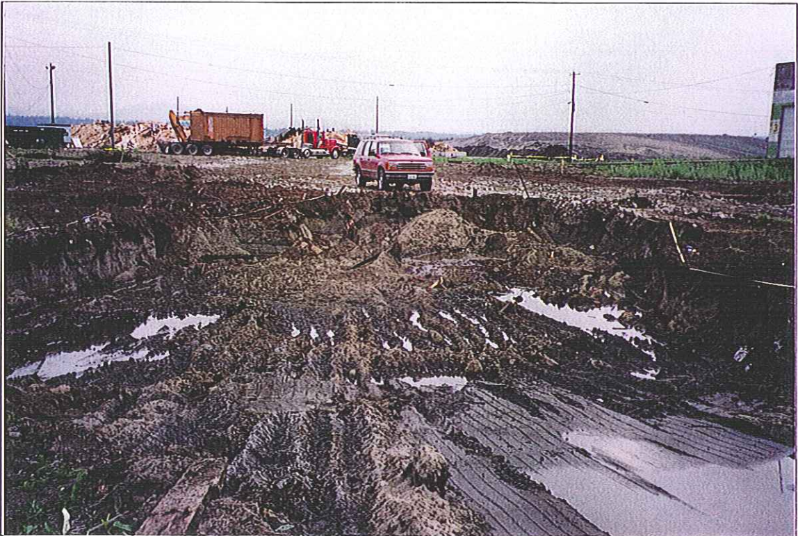
Area 10-4A Extended Excavation Area (Looking East)
