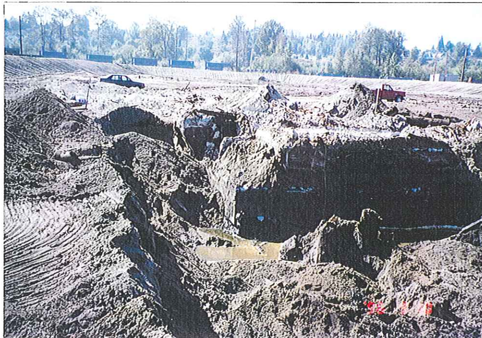
Area 7-1 Excavation Area Showing Concrete Structure (Looking Northwest)
