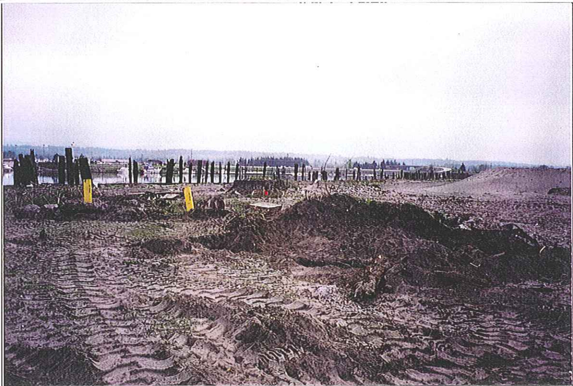
Area 7-2C Excavation Area (Looking Southeast)
