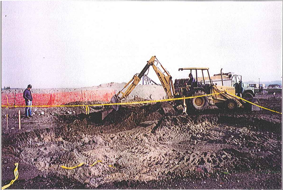
Area 8-2 Excavation Area (Looking Northwest - Fenced Area 8-1 in background)
