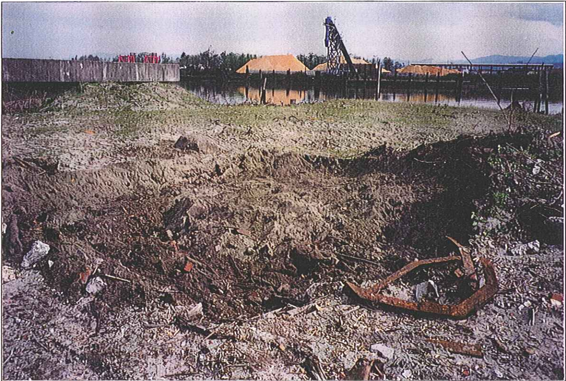
Area 7-2C Excavation Area (Looking Northeast)
