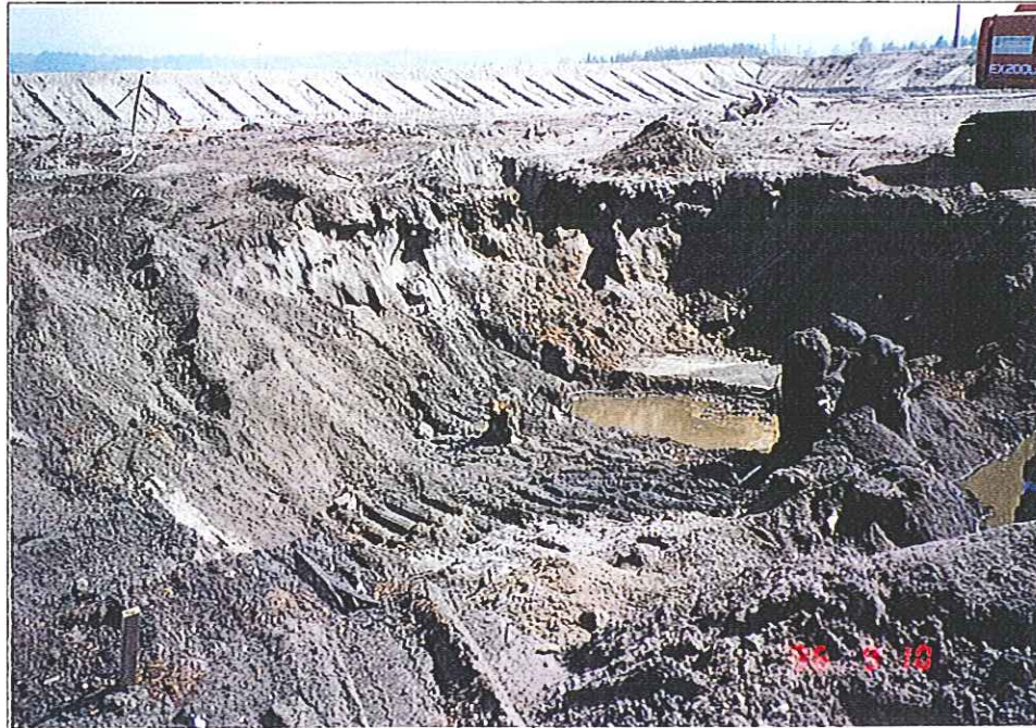
Area 7-1 During Excavation Showing Concrete Structure (Looking East)
