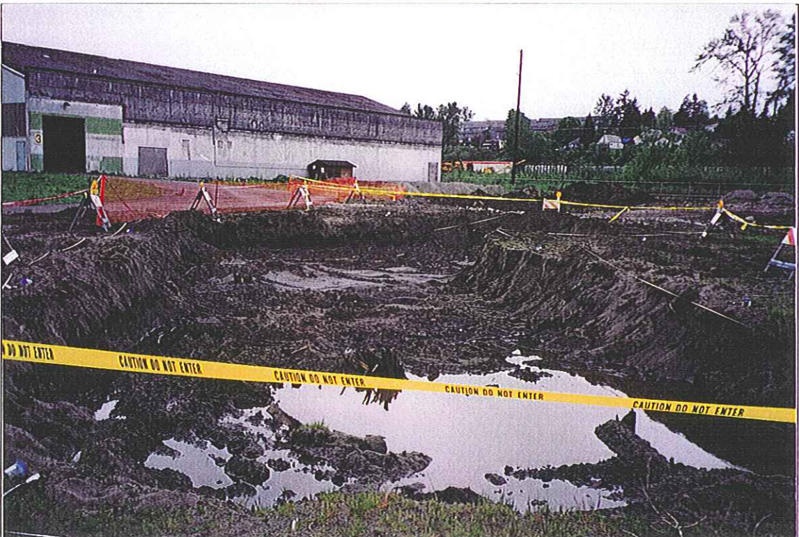
Area 10-3A Excavation Area (Looking Southwest)
