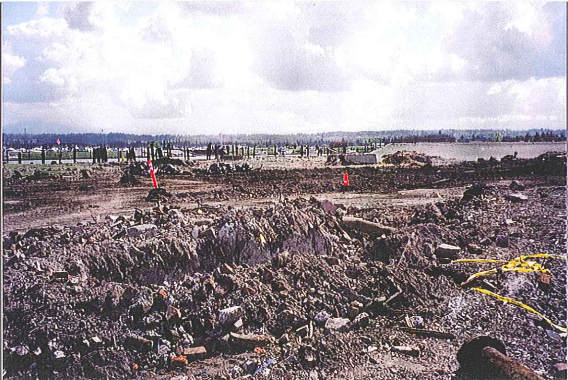
Area 7-2A Removal of Debris to Concrete Slab (Looking East)
