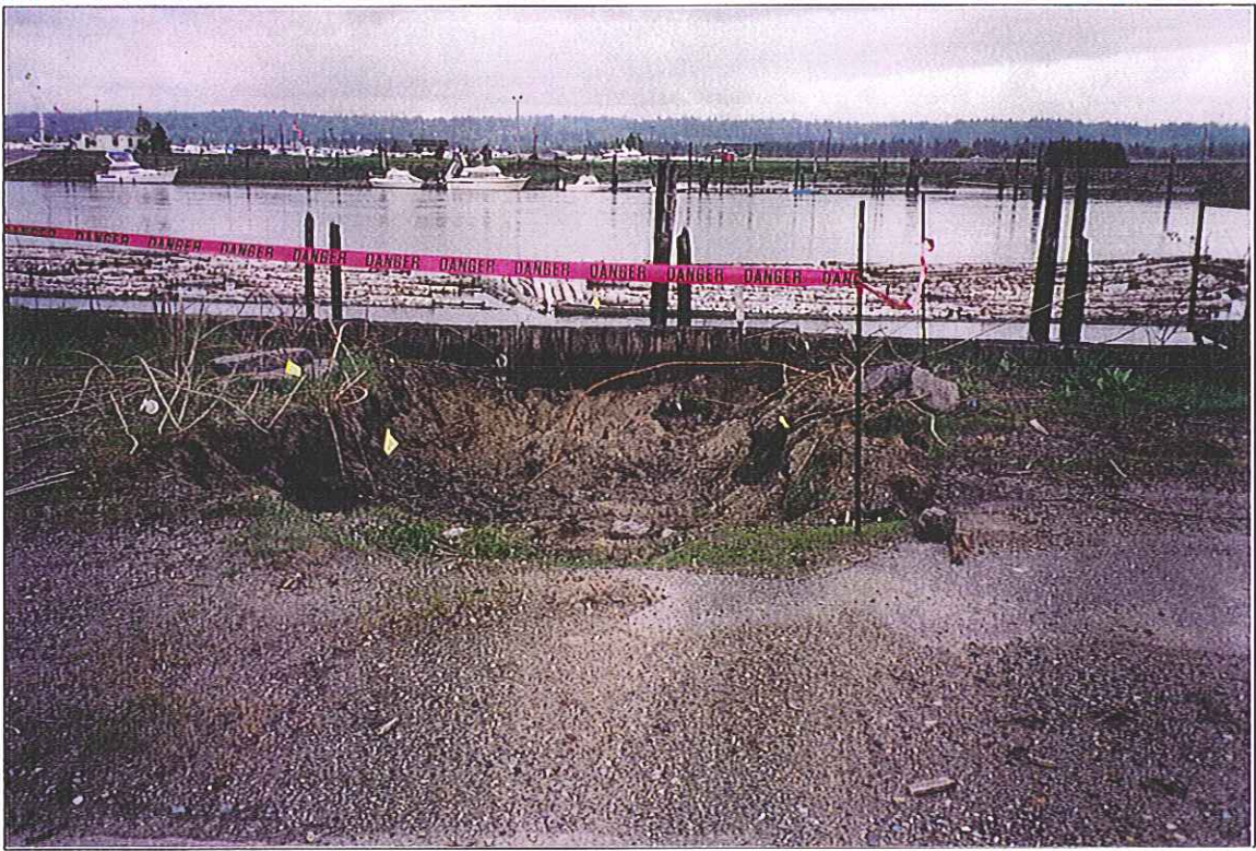
Area 8-3B Excavation Area (Looking East)
