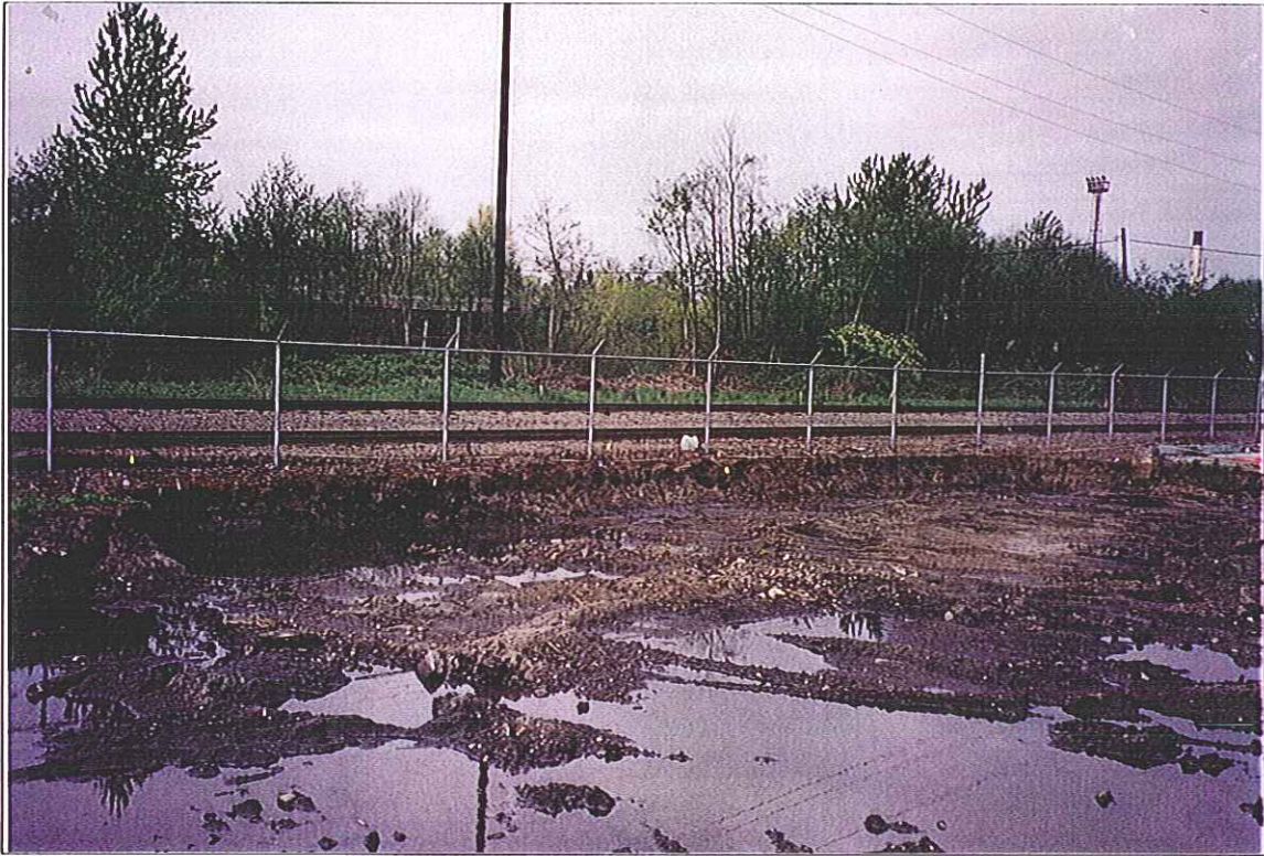
Area 10-1 During Excavation (Looking West)
