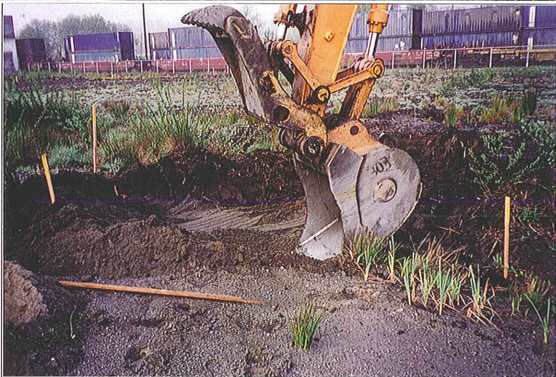
Area 10-2 During Excavation (Looking Southwest)
