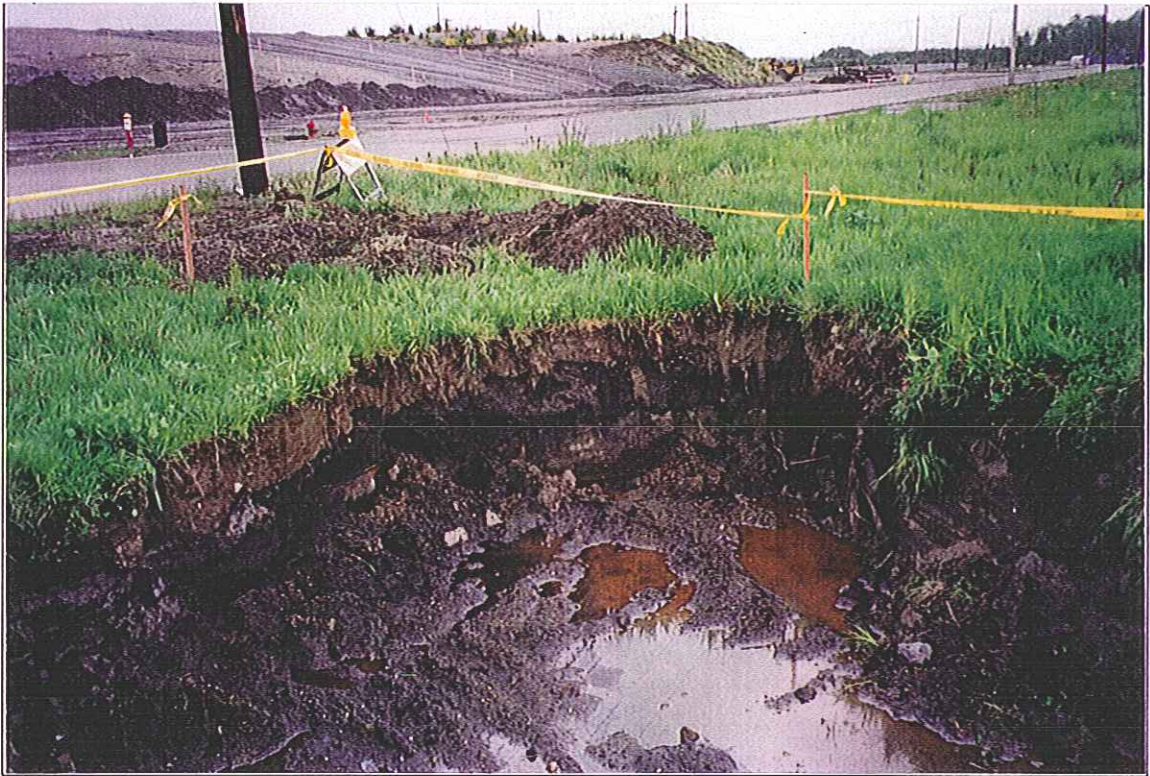
Area 10-3B Excavation Area (Looking Southeast)
