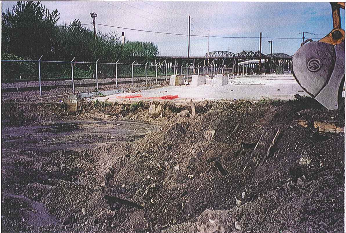
Area 10-1 During Excavation (Looking Northwest)
