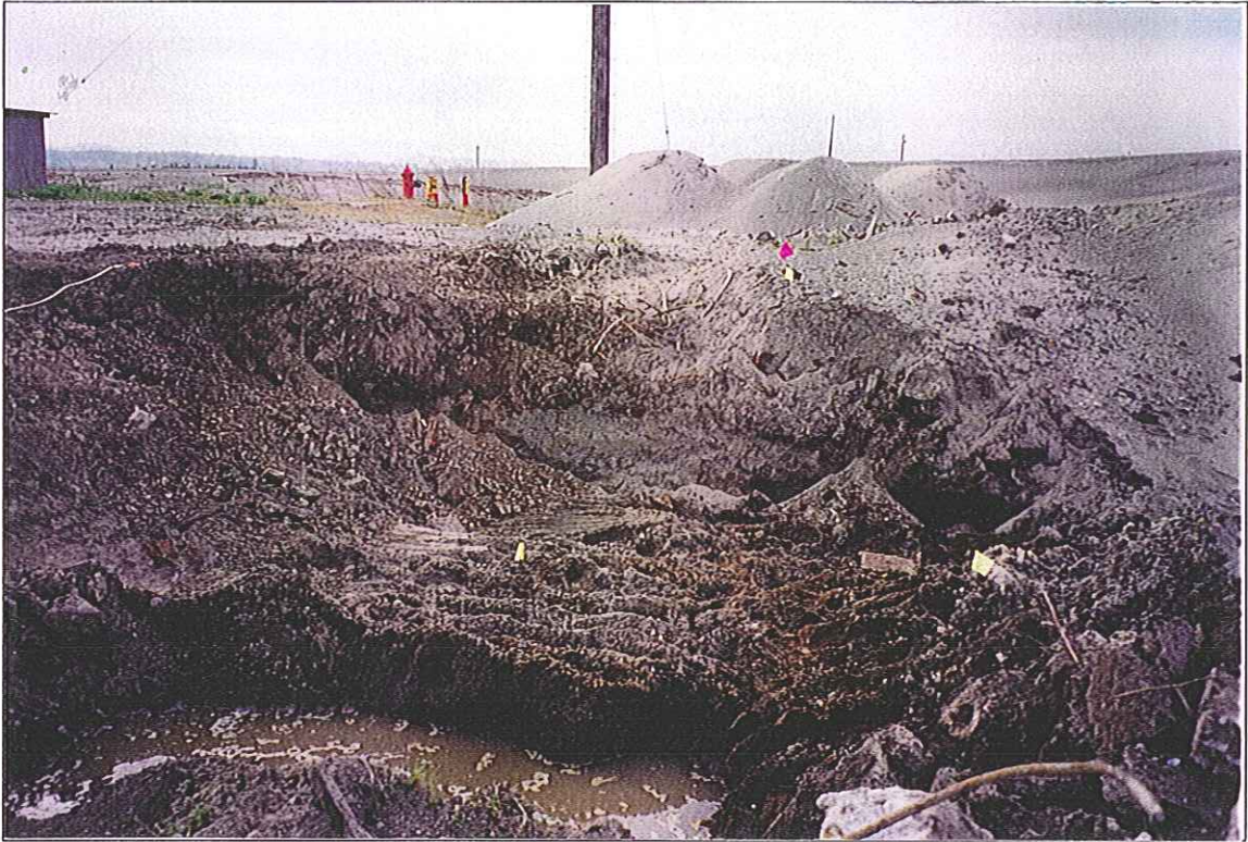
Area 9-1 Excavation Area (Looking Southeast)
