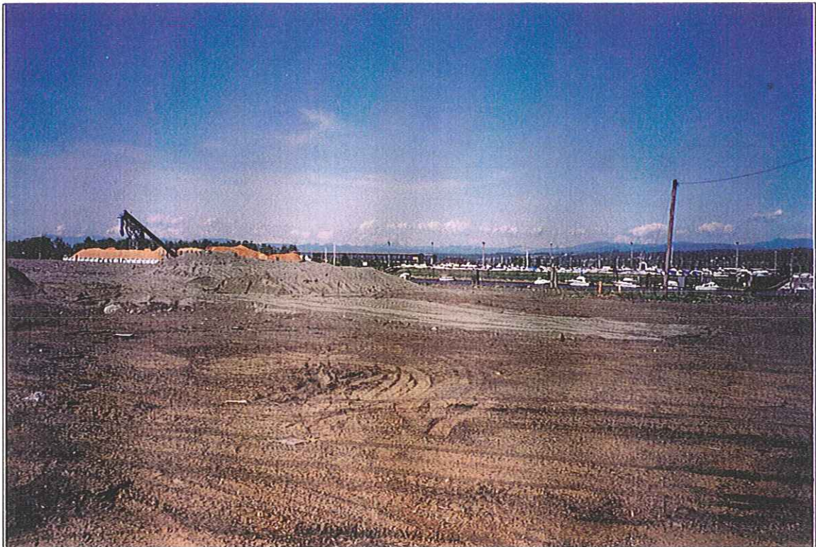
Areas 8-1 and 8-2 Backfilled
