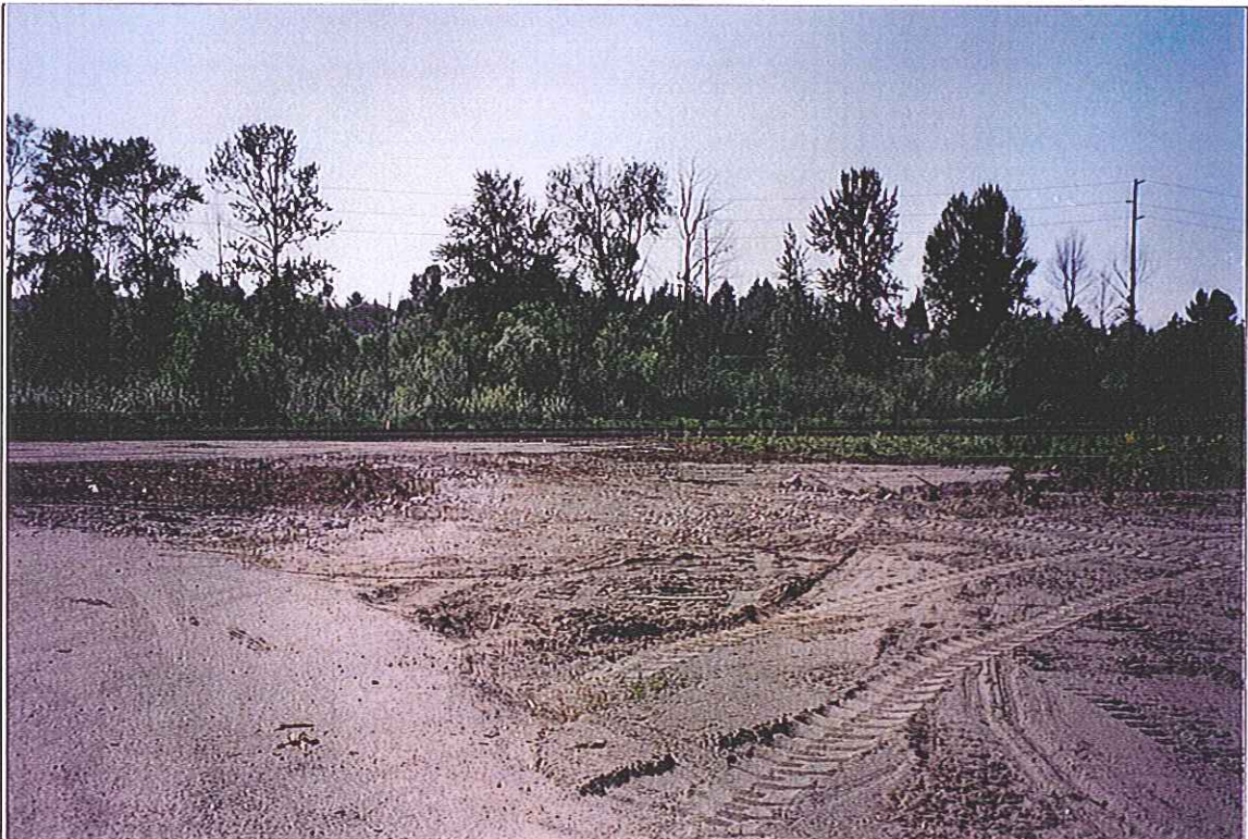
Portion of Area 10-4 Backfilled (Looking West)
