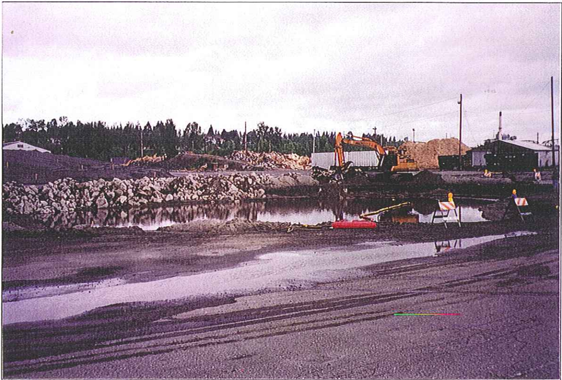
Area 8-3A Initial Backfilling (Looking Northwest)
