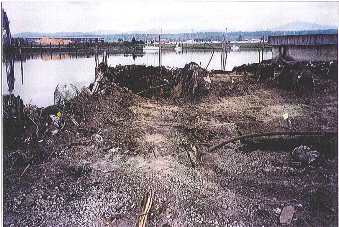
Area 7-2B Excavation Area (Looking East)
