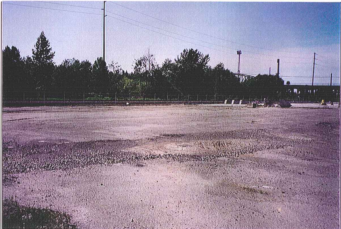
Area 10-1 Backfilled (Looking West)
