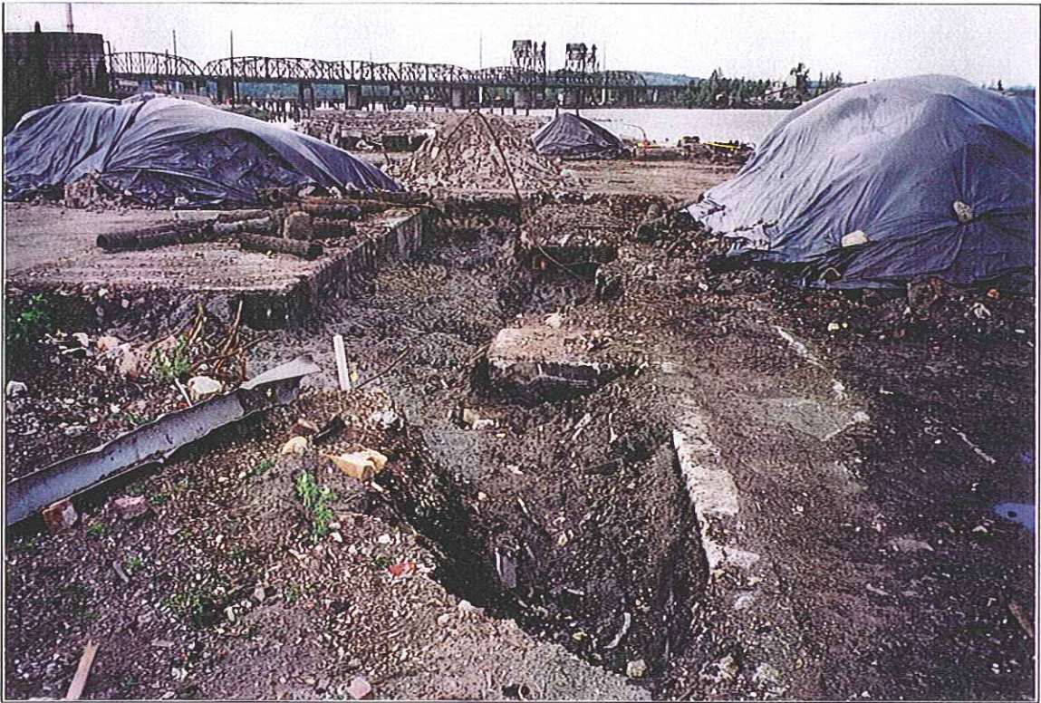
Area 7-2A Debris Removal in Central Area (Looking North)
