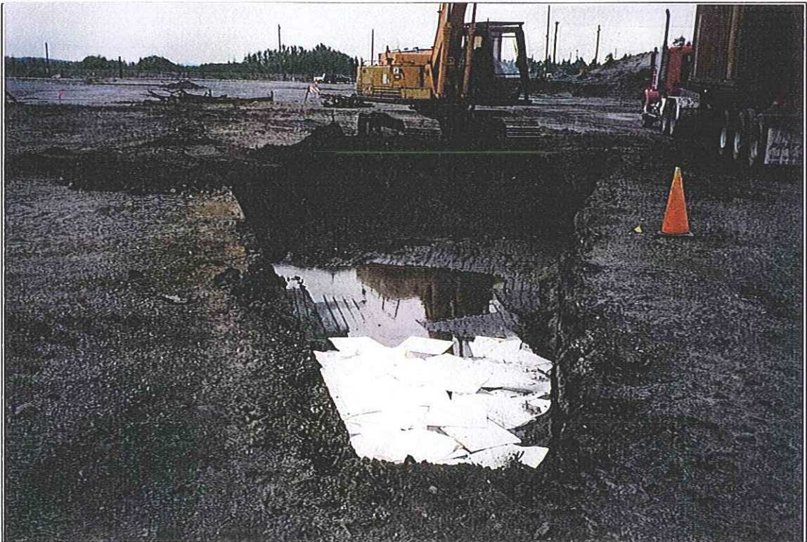
Area 8-3A Initial Excavation (Looking Southeast)
