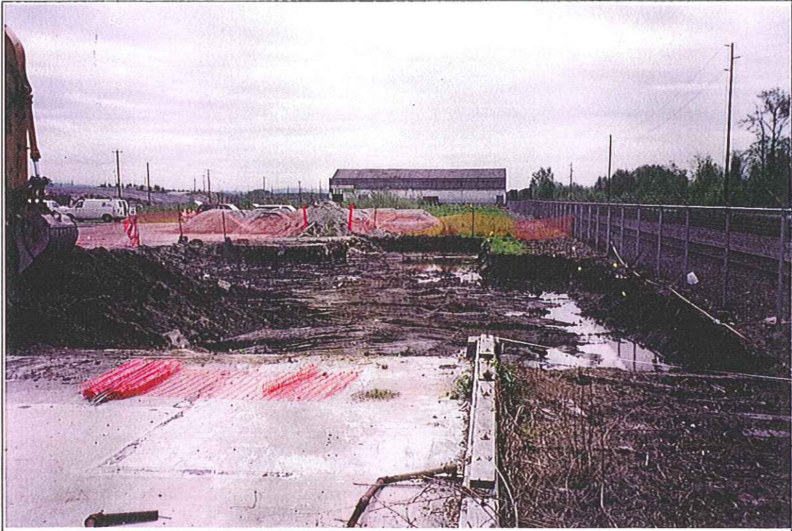
Area 10-1 During Excavation (Looking Southeast)
