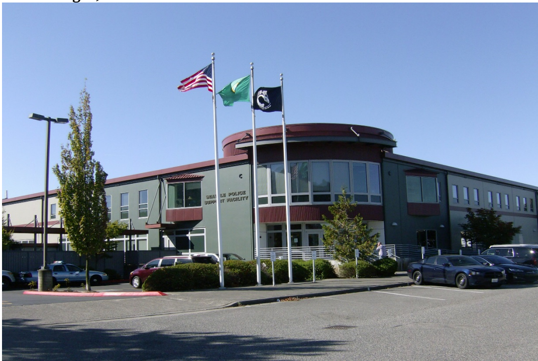
Photo 1: Building C, north end - from the east
