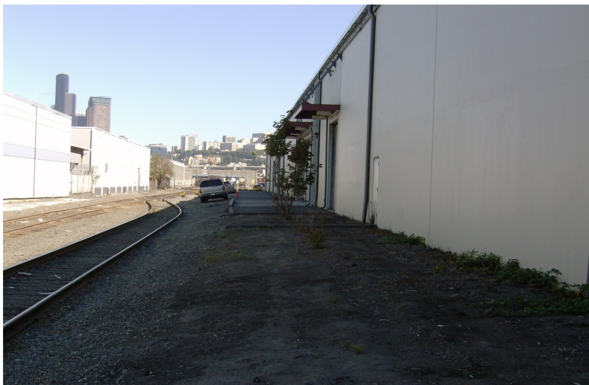
Photo 4: Building C, back along railroad tracks south end looing North.
