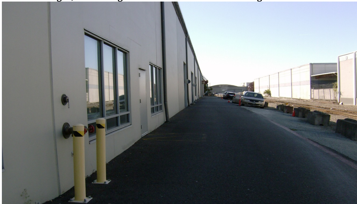
Photo 3: Building C, back along railroad tracks north end looing south.
