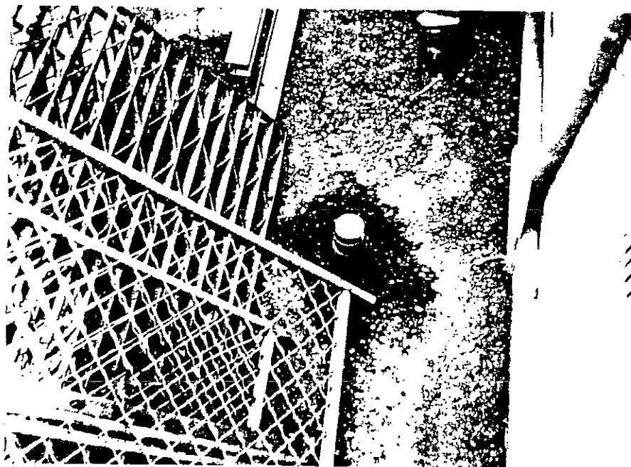
PHOTO 4: FILL PIPE TO HEATING OIL, UST, WEST END OF OLD FEED STORE
