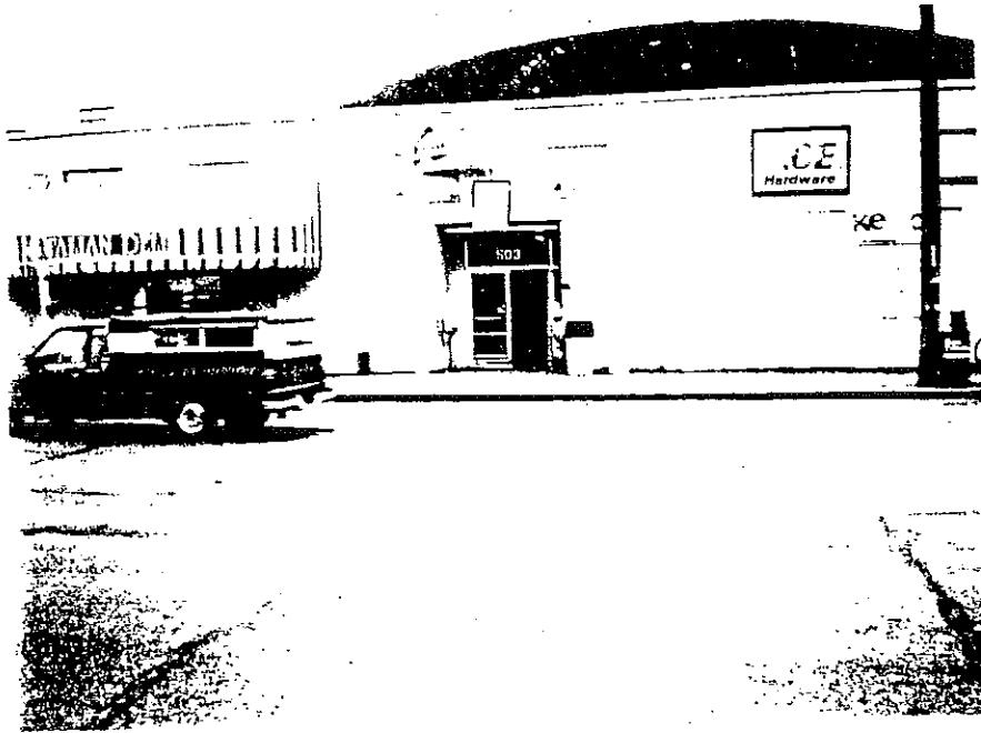
PHOTO 1: FACING WEST. ENTRANCE TO WEST BUILDING
