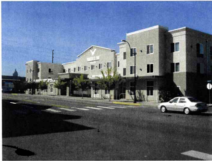
EASTERN PORTION OF PROJECT SITE. PHOTOGRAPH TAKEN FACING SOUTHWEST.
