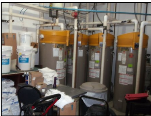
11 : Natural gas-fired water heaters and swimming pool chemicals
