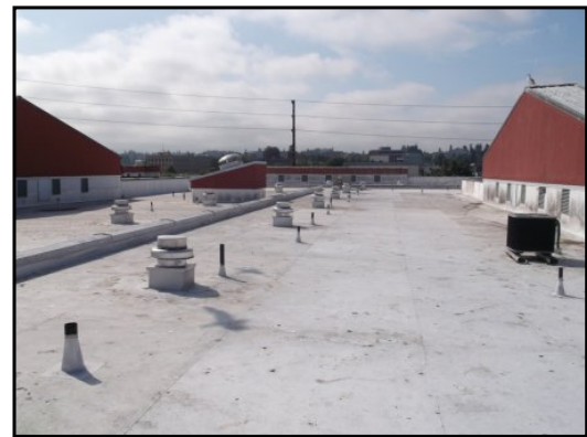
10 : Roof and HVAC equipment
