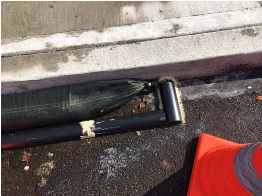
Photograph 2. Upgradient end of filter sock, bolted to concrete curb.
