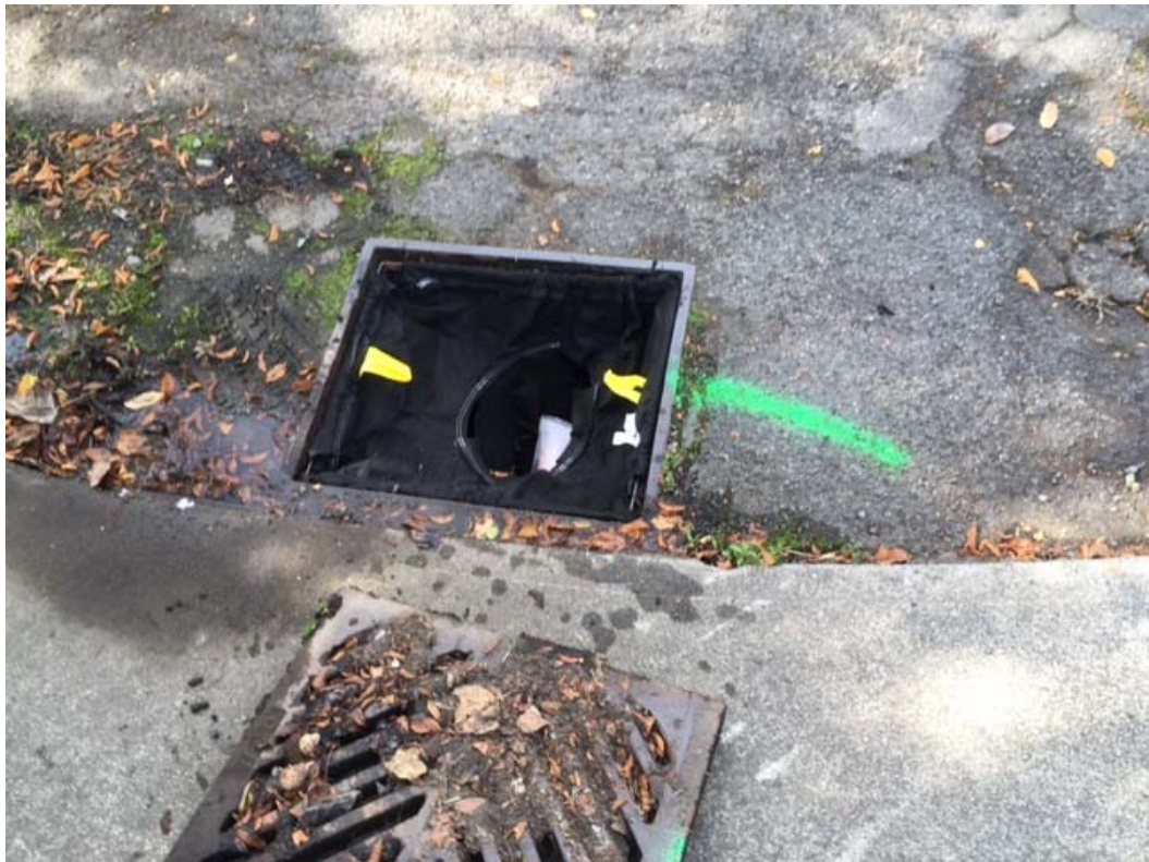
Photograph 4. Filter insert installed in downgradient catch basin.
