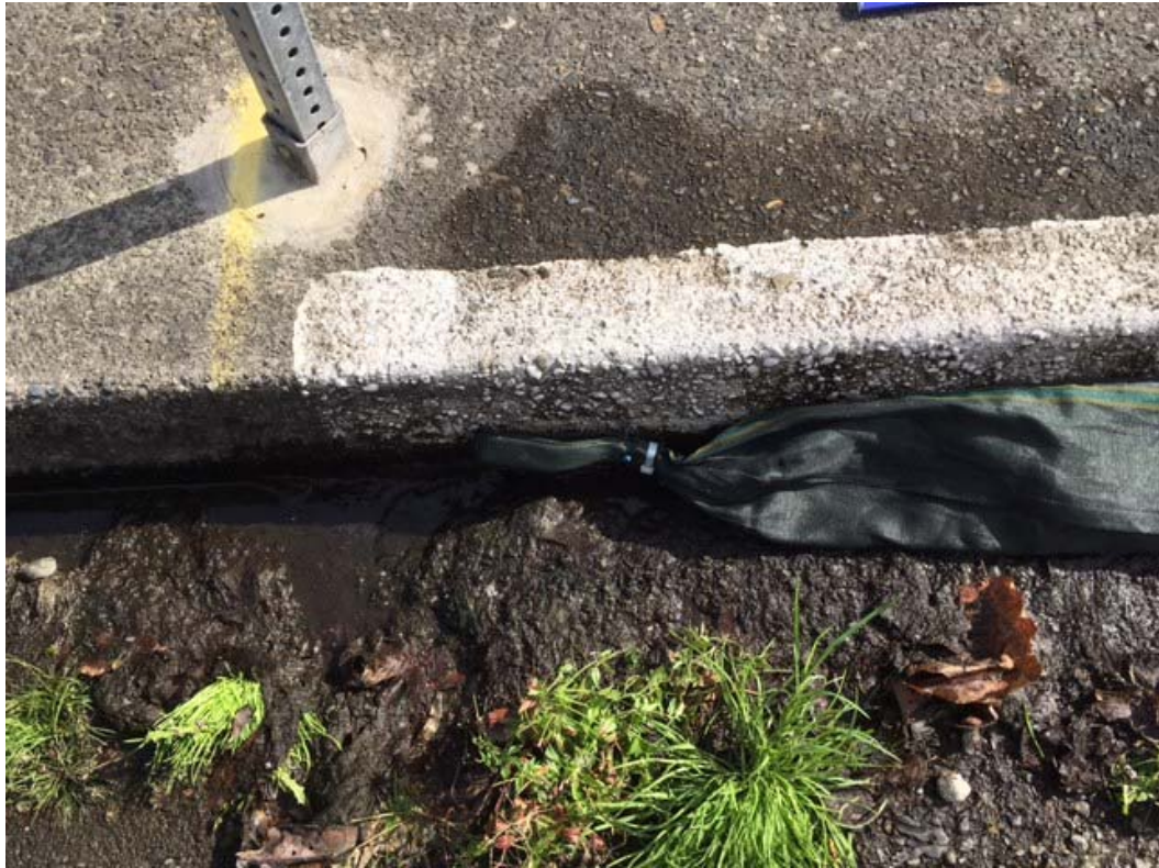
Photograph 3. Downgradient end of filter sock, bolted to concrete curb.
