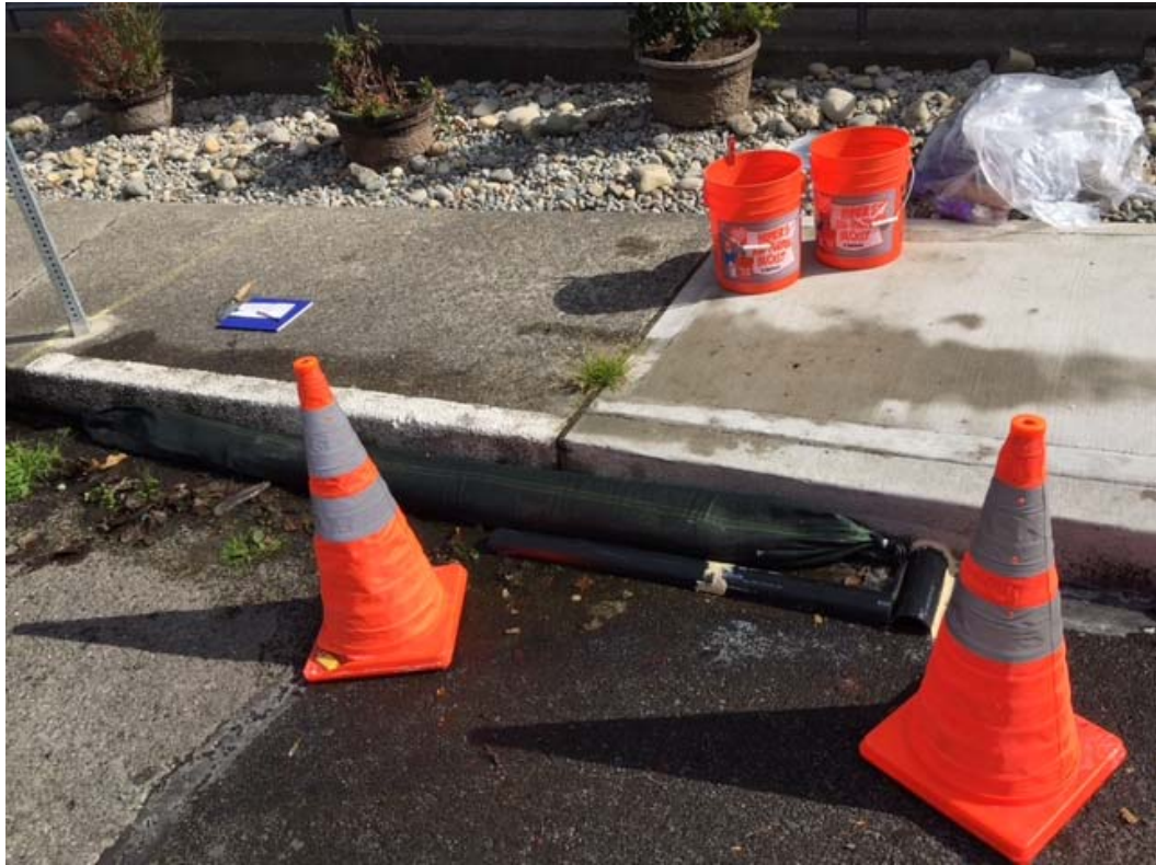
Photograph 1. Filter sock at curb line and ABS pipe berm.
