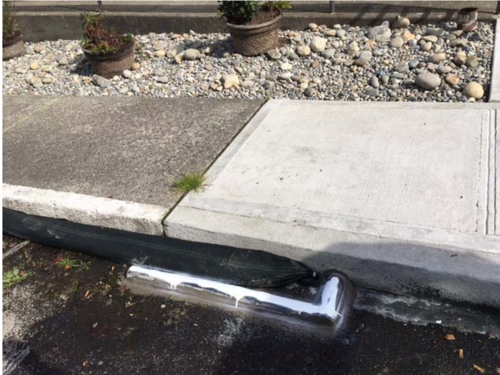
Photograph 5. Filter sock and berm reinforced with hydraulic cement.
