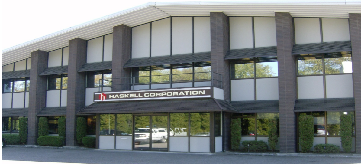
Photo 1: Haskell Corporation Building near the entrance to the commercial park.
