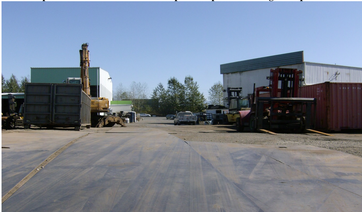
Photo 2: Cap area at center east side – steel plates to prevent damage to cap.
