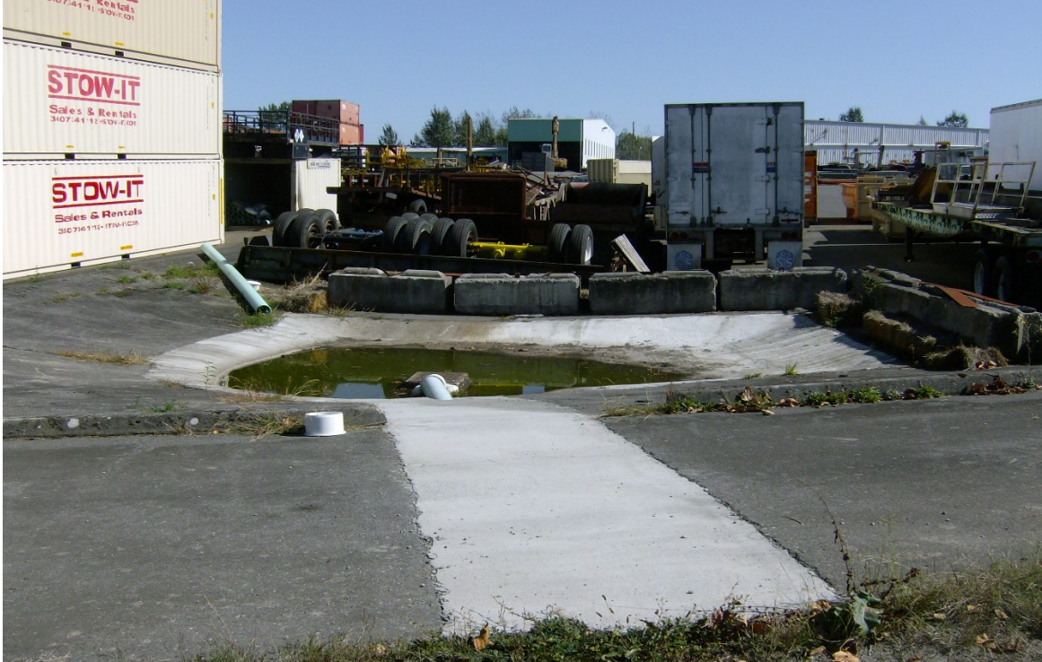
Photo 3: Paved capped area – surface collection basin - from the east
