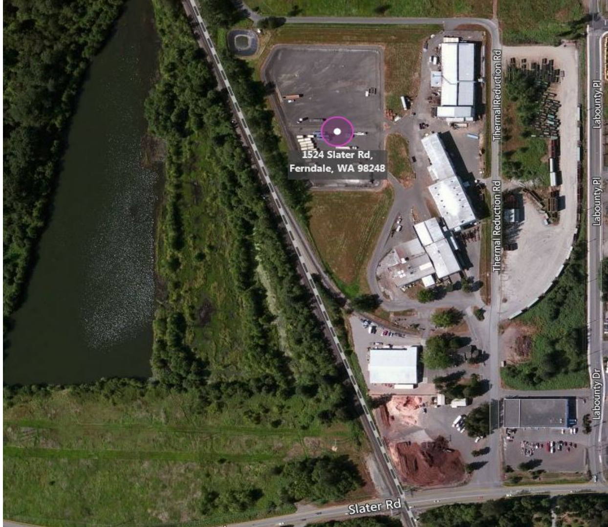
Photo 5. Recomp of Washington (Scrap-it) pad and buildings - Aerial View.
