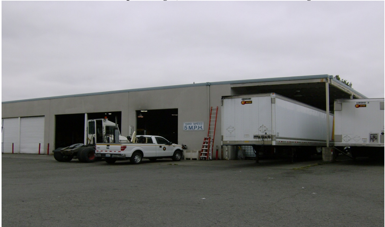
Photo 1: UST under concrete pad at right, south side of maintenance bldg.
