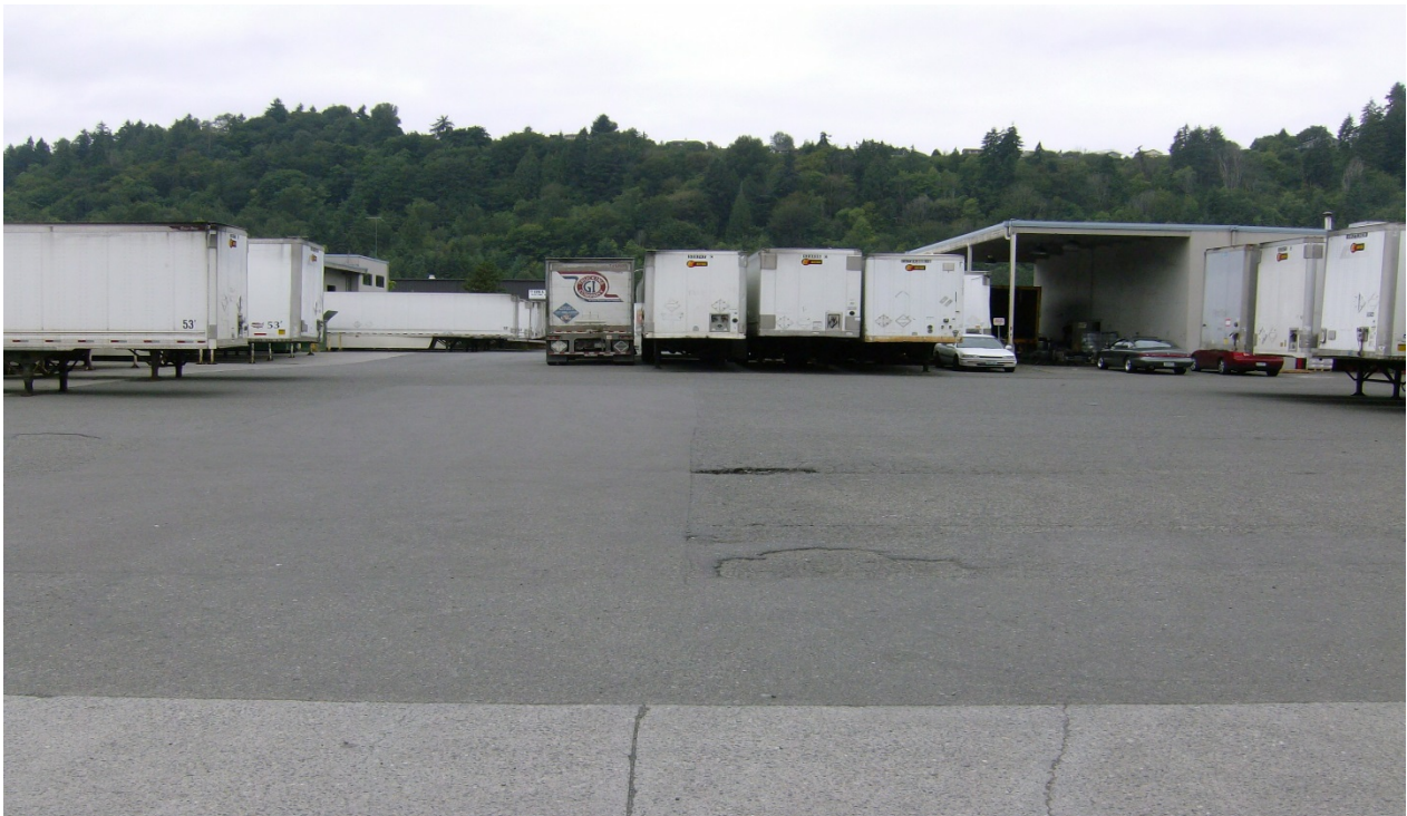
Photo 2: Asphalt area southeast of the maintenance building at the right.
