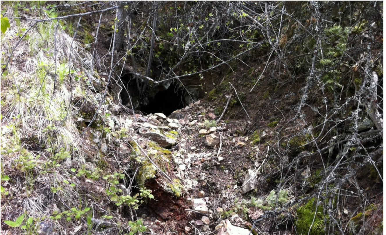
Typical adit partially blocked by soil and rock.
