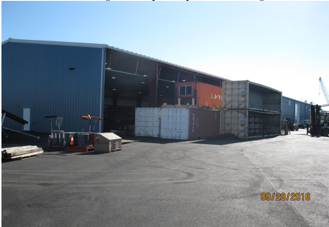
Photo 4: Former Pond Site Engineered Asphalt Cap and New Building – from the Southeast
