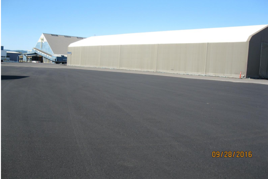
Photo 3: Former Pond Site Engineered Asphalt Cap – from the West
