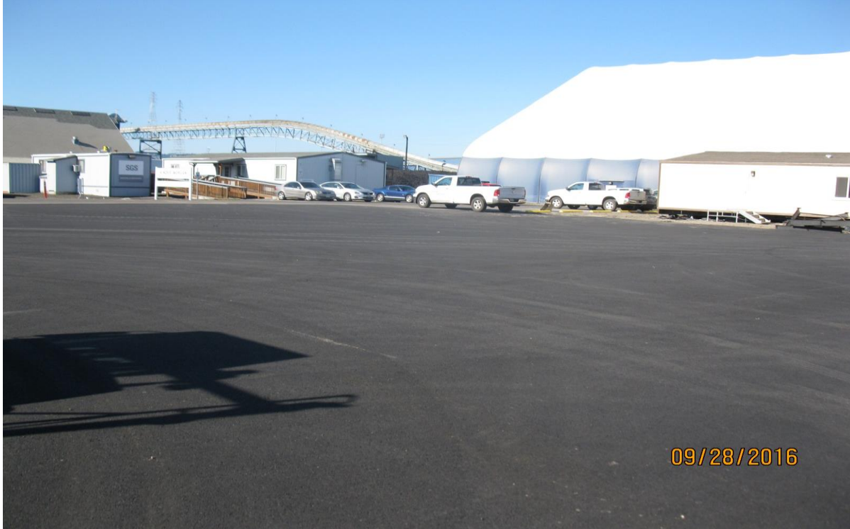
Photo 5: Former Pond Site Engineered Asphalt Cap – form the Northwest
