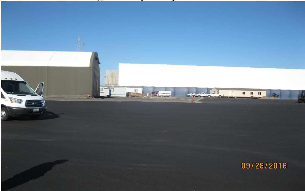
Photo 2: Former Pond Site Engineered Asphalt Cap – from the North
