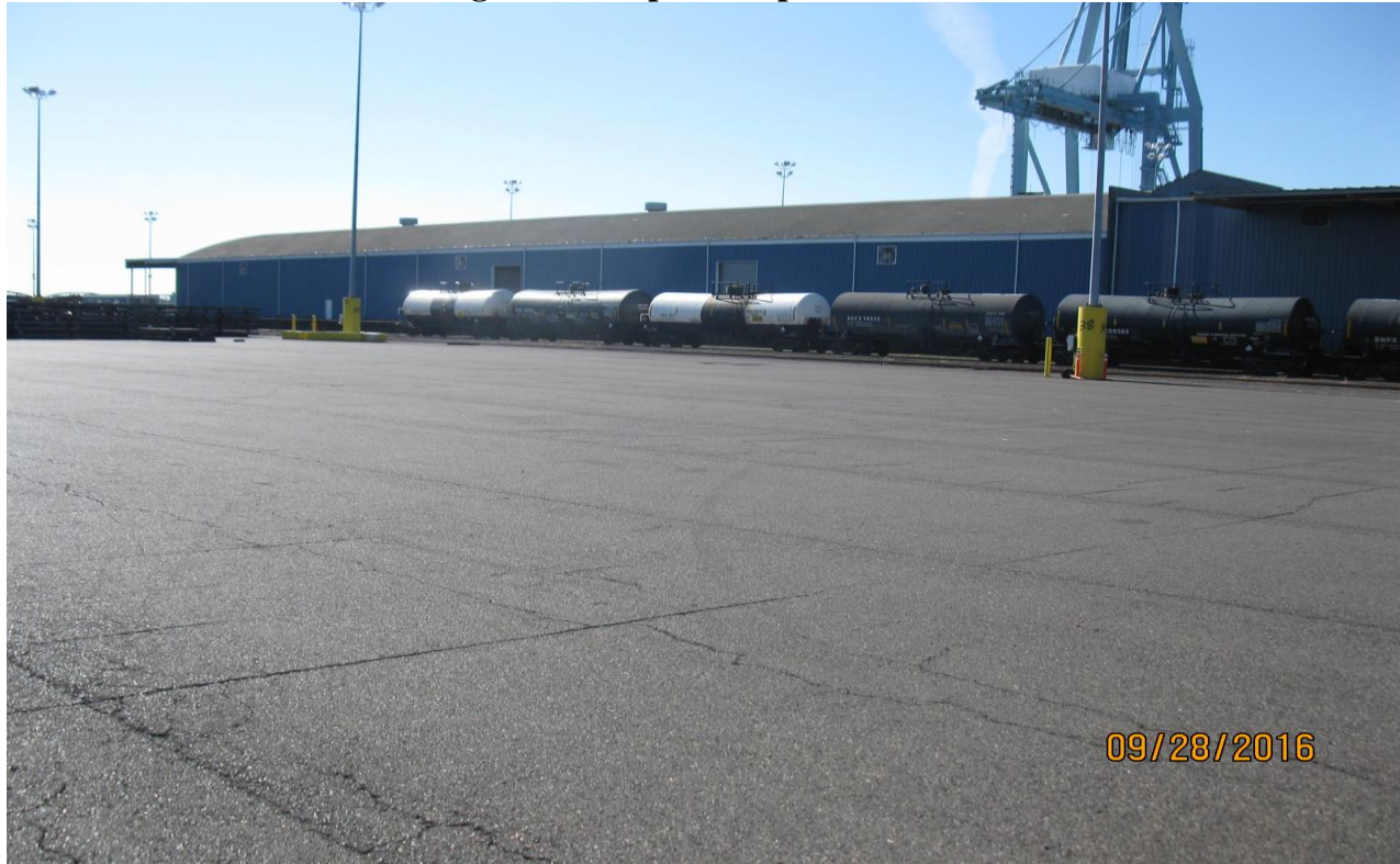
Photo 8: Former Plant Site Engineered Asphalt Cap – from the North
