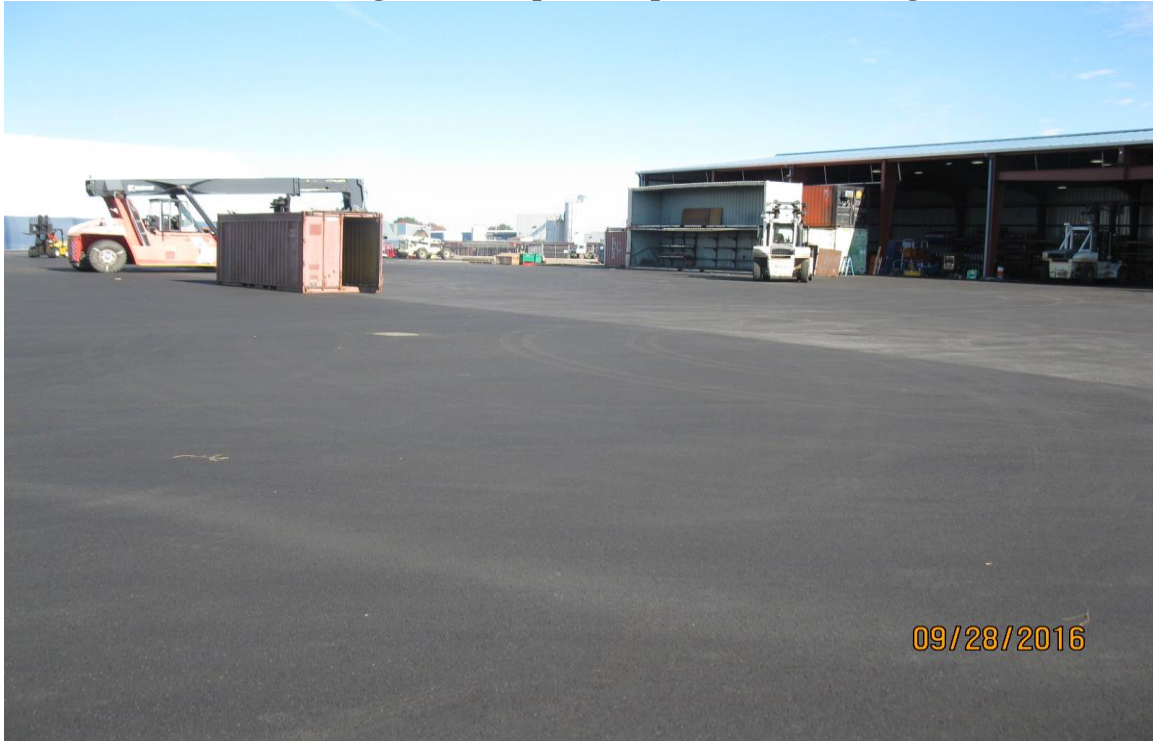
Photo 1: Former Pond Site Engineered Asphalt Cap and New Building—from the Southeast
