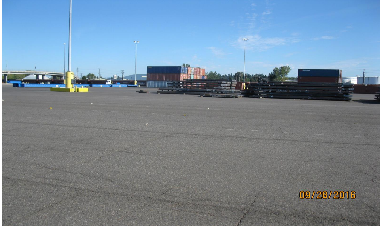
Photo 7: Former Plant Site Engineered Asphalt Cap – from the Southwest
