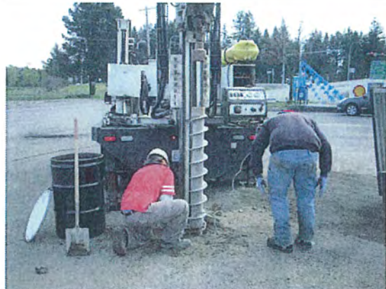
Photo #4: Drilling New Monitoring Well WDOE-6AR (Looking Northeast)
