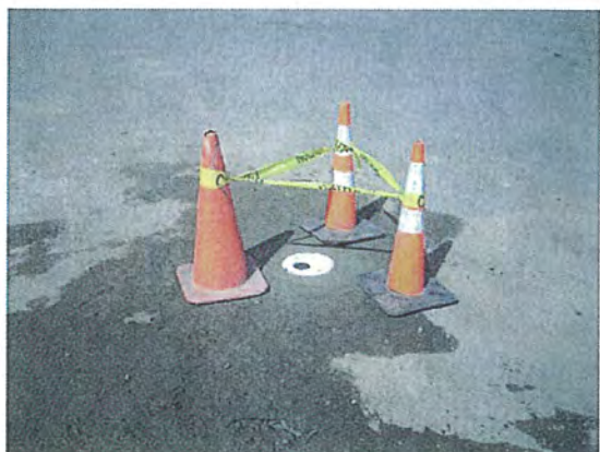
Photo #6: Completed Monitoring Well WDOE-6AR
