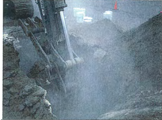
Photo #2: Mixing ORC-A into the Backfill of the Excavation
