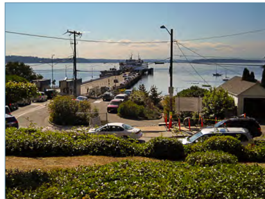
Barton Pump Station, Seattle, Washington
