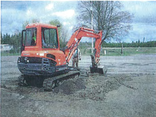
Photo #3: Preparing the Excavation Area for Paving.(Looking Northwest)
