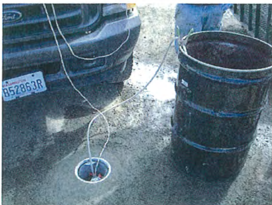
Photo #5: Tubing and Barrel showing setup for Well Development
