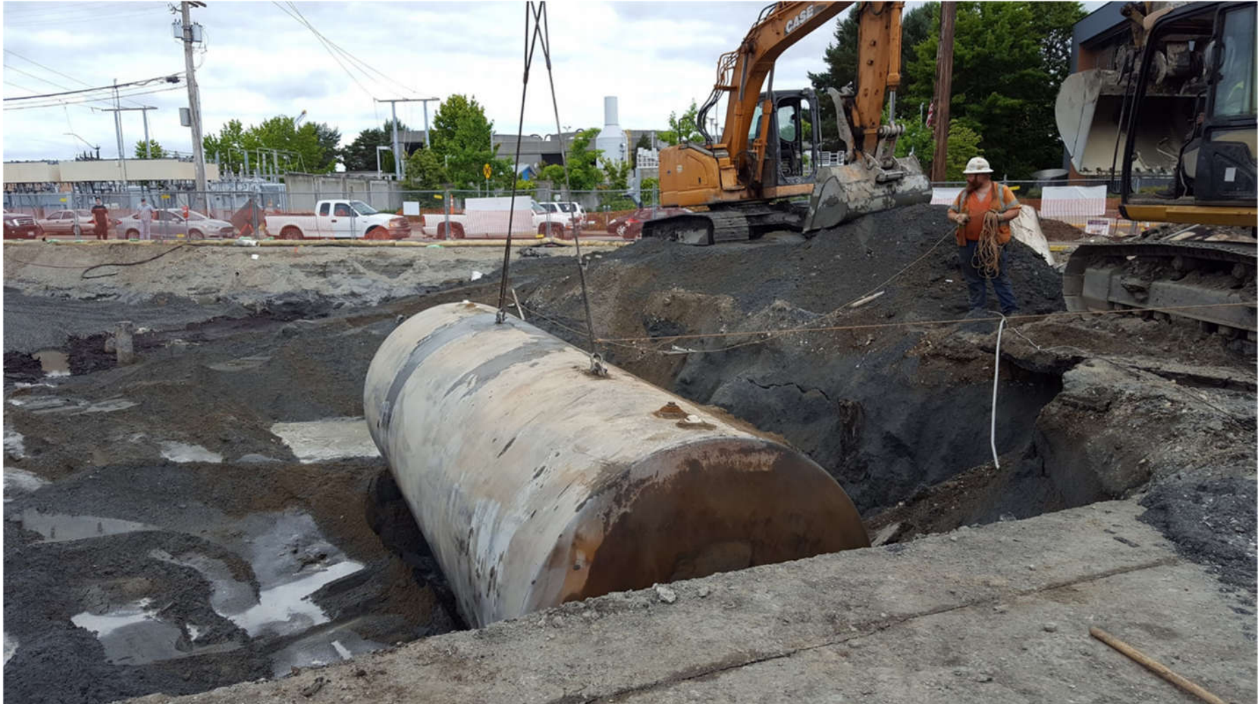
Photo # 18: Removal of TANK-4. No visible holes, pits, or damage observed.
