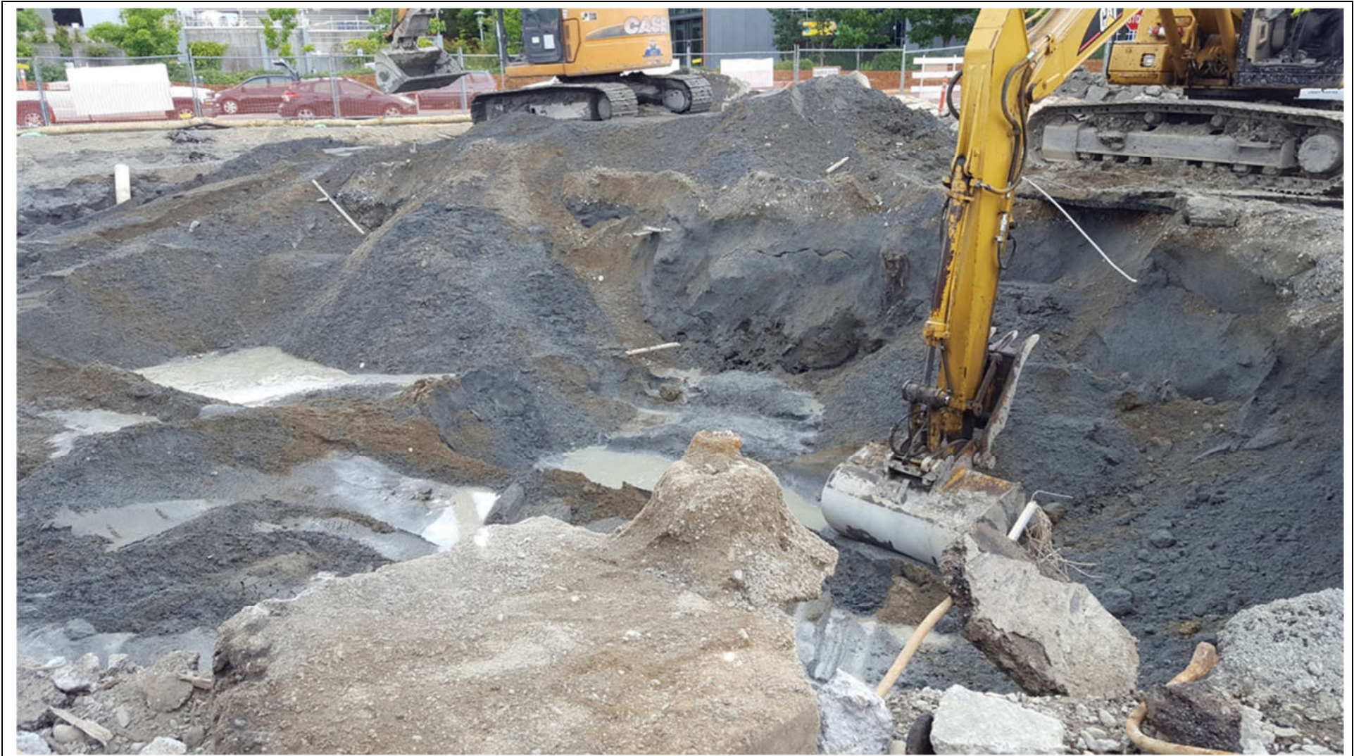
Photo # 22: Excavated tank pit.
