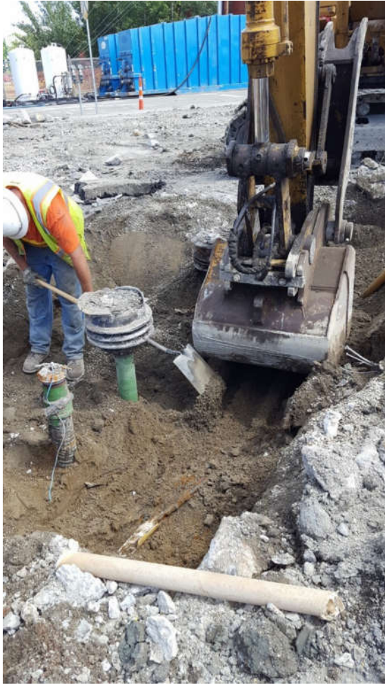
Photo # 14: Hand digging around fill ports/turbines as to not break the piping from the UST.
