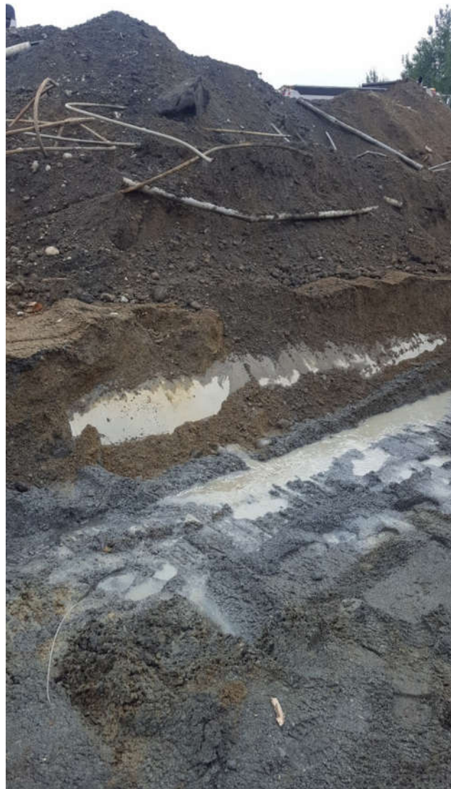
Stockpile of soil along the eastern side of the Property showing the vent lines from the former USTs.
