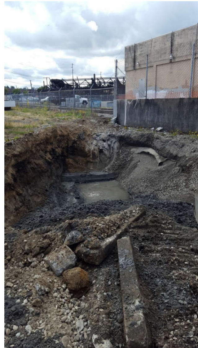
Photo # 2: End of Day 1, area where historical diesel AST excavated.
