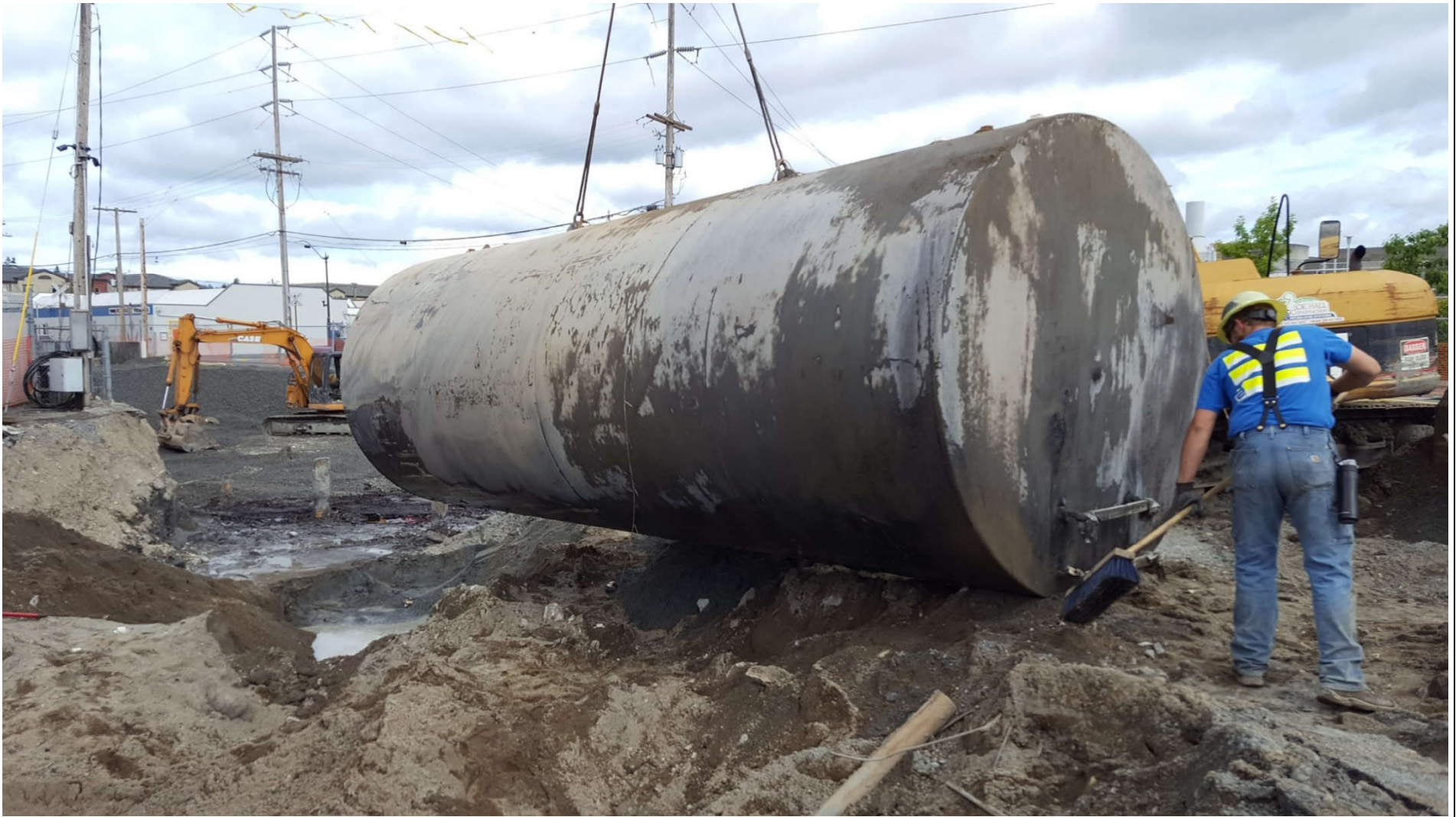
Photo # 17: Removal of TANK-1. No visible holes, pits, or damage observed.
