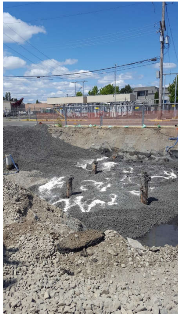
Photo #12: ORC-A spread around the clean backfill on the westside.
