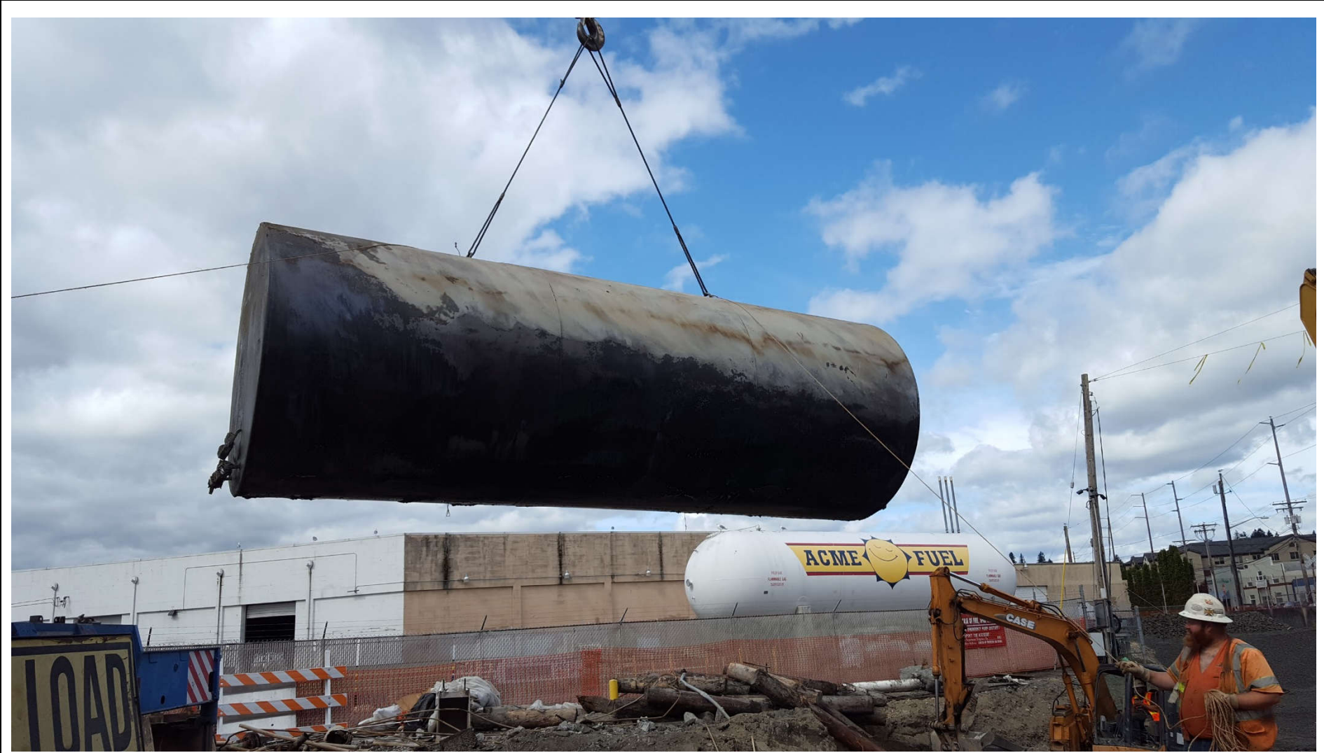
Photo # 20: Removal of TANK-2. No visible holes, pits, or damage observed.
