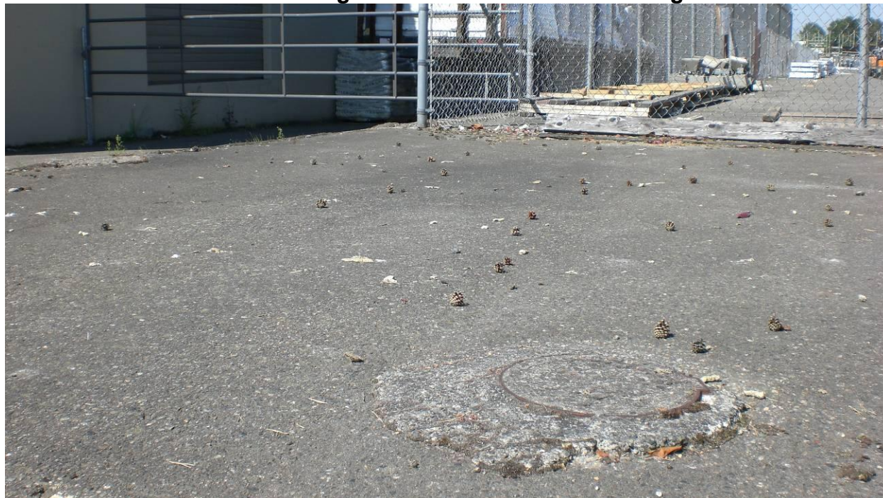
Photo 3: Abandoned Monitoring Well on North Side of Building – from the east
