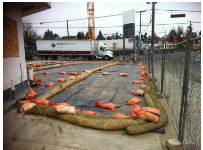
Photograph 12. Site backfilled and covered, December 10, 2013.
