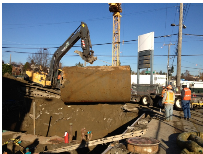
Photograph 6. Loading UST #3 on December 4, 2013.
