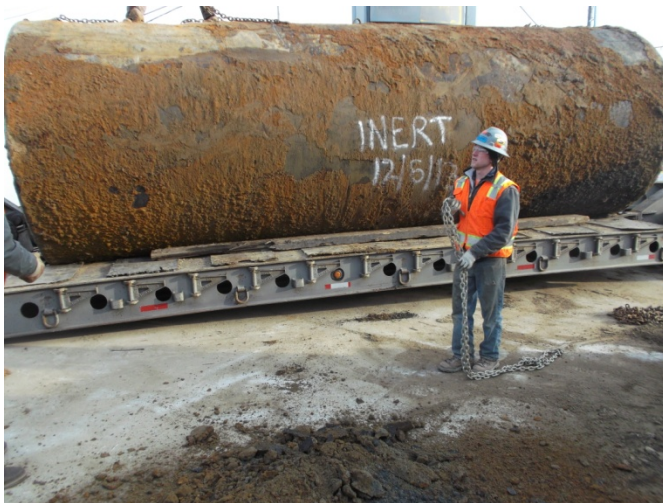
Photograph 11. Preparing UST #4 for transport, December 5, 2013.
