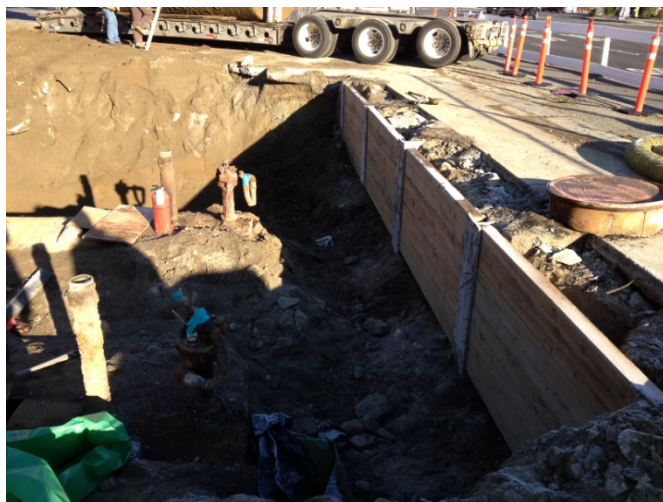
Photograph 4. Installation of lagging to support the Fautleroy sidewalk, December 3, 2013.
