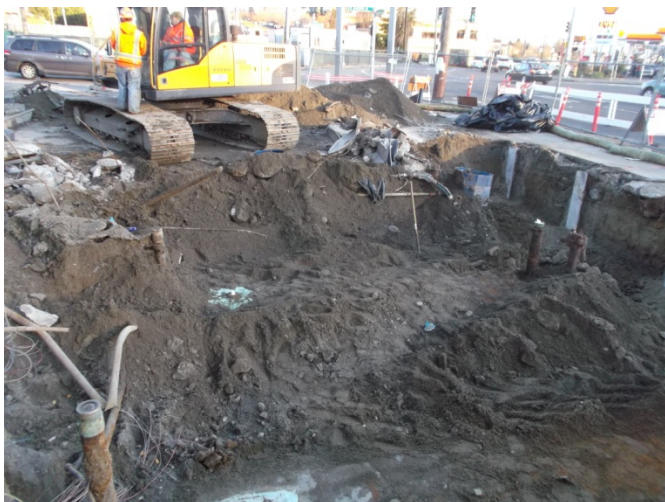
Photograph 3. Removal of overburden for USTs #2 and #3 on December 3, 2013.
