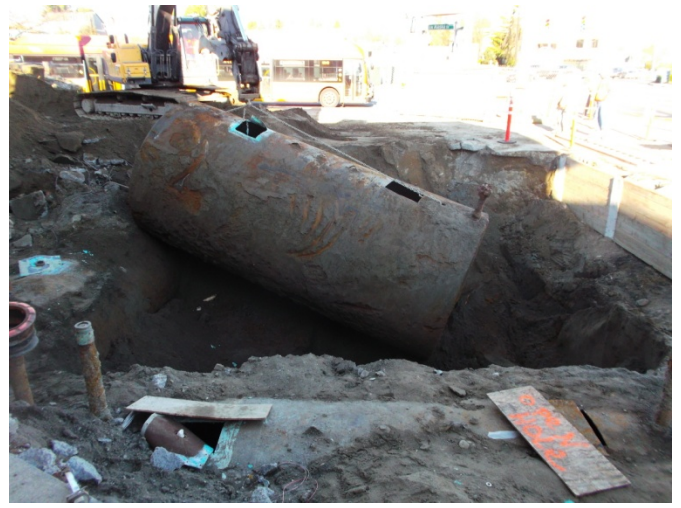
Photograph 8. Removal of UST #2 on December 4, 2013.
