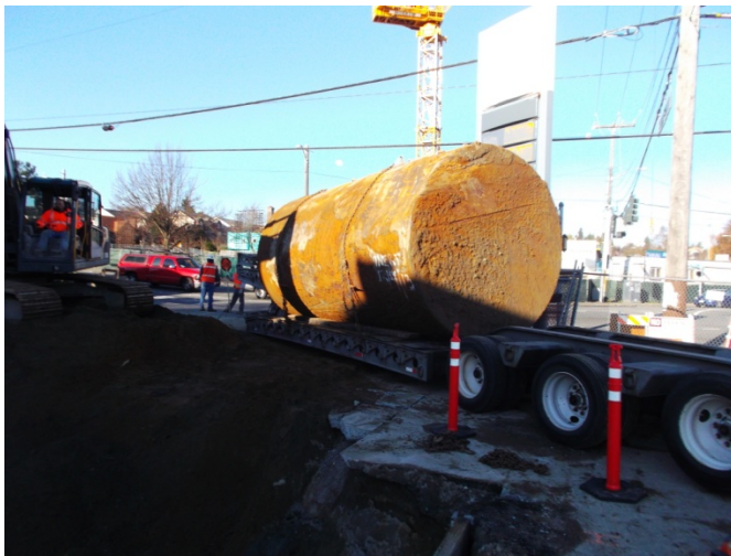
Photograph 9. Loading UST #1 on December 5, 2013.
