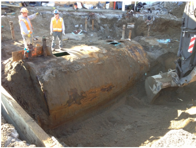
Photograph 7. Preparing for removal of UST #2 on December 4, 2013.
