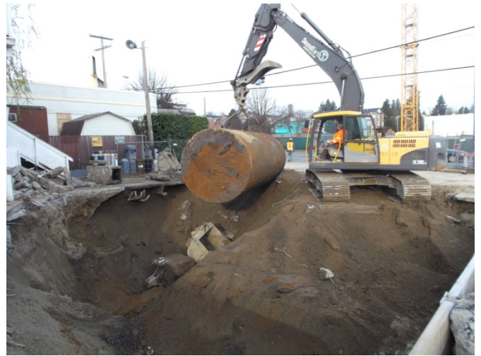
Photograph 10. Removal of UST #4 on December 5, 2013.
