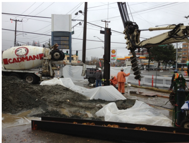
Photograph 2. Auger borings and installation of pilings by Kulchin, November 12, 2013.
