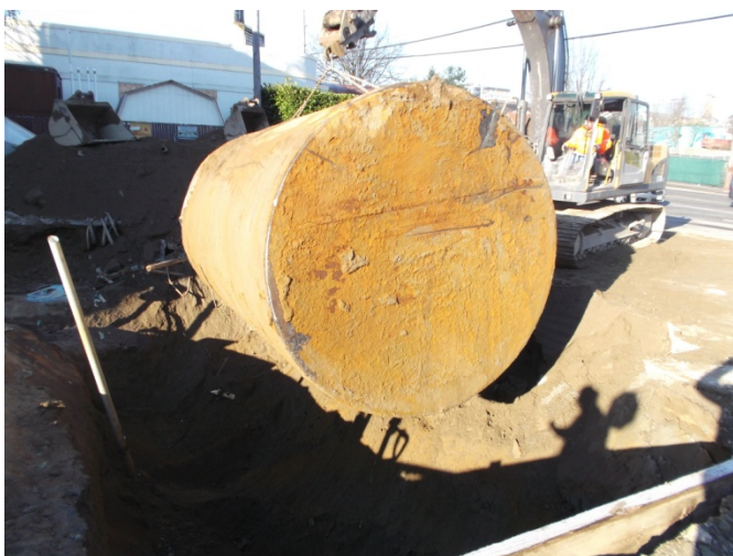
Photograph 5. Removal of UST #3 on December 4, 2013.
