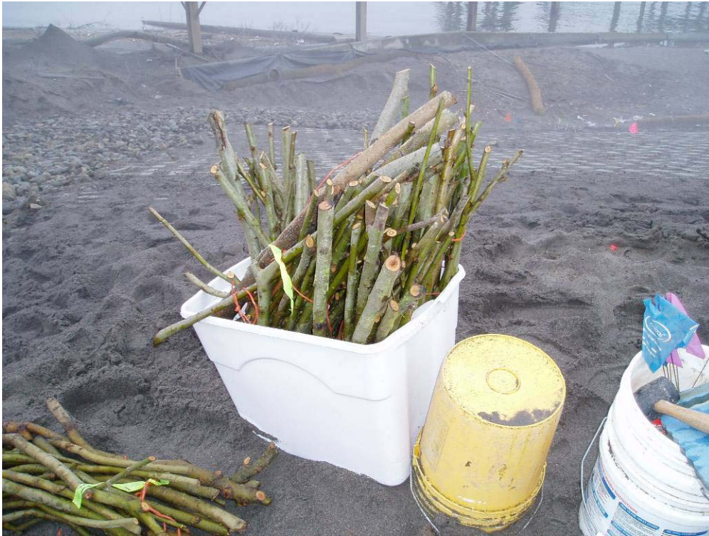
50017 December, 2003 - Live stakes delivered in container filled with water, per the requirements of the vendor and the specifications.
