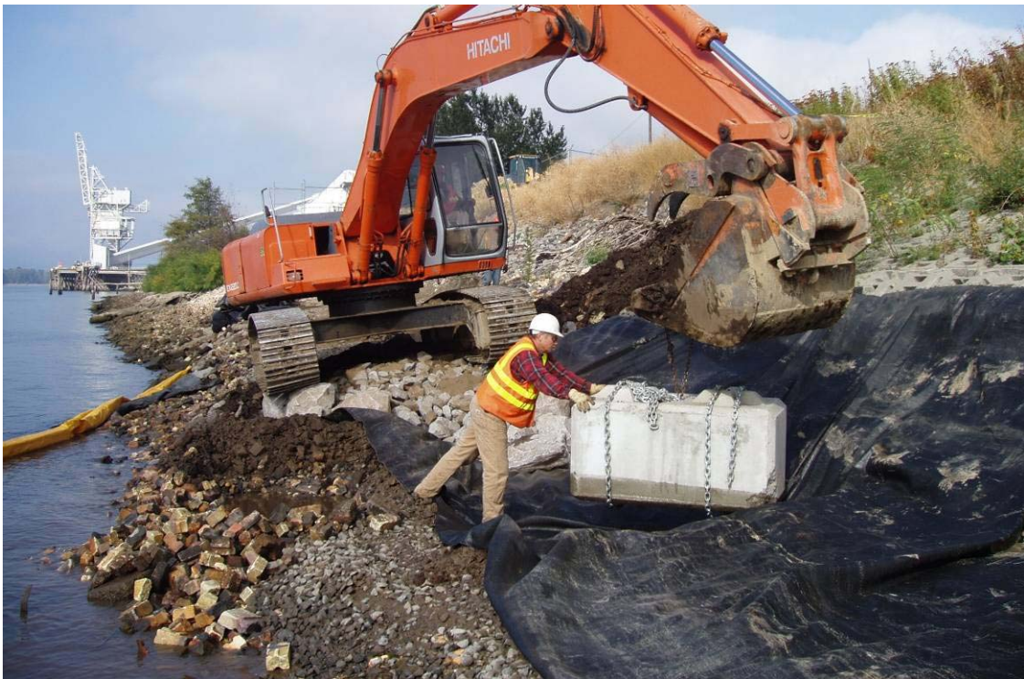
0603 October 5, 2006 – Placement of ecology block , in preparation for rootwad installation. Placement over filterfabric. Looking west.
