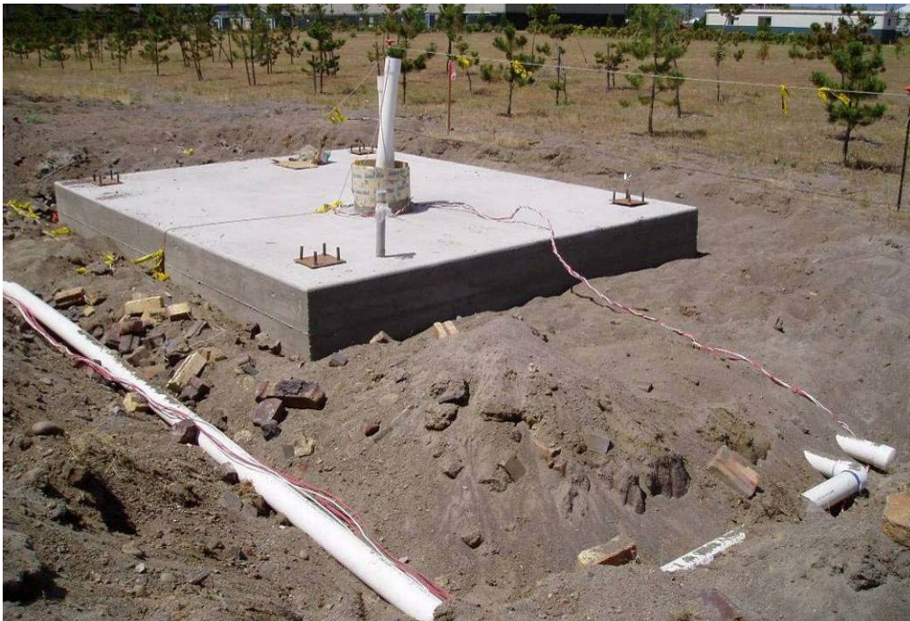
90004 July, 2004 - Concrete foundation and slab of Storage –Operations Building. Looking northwest.
