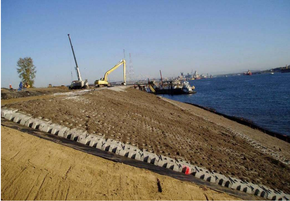
30086 December, 2003 – Placement of topsoil with open spaces of “Armorflex’ panels using extend reach excavator. Looking east.
