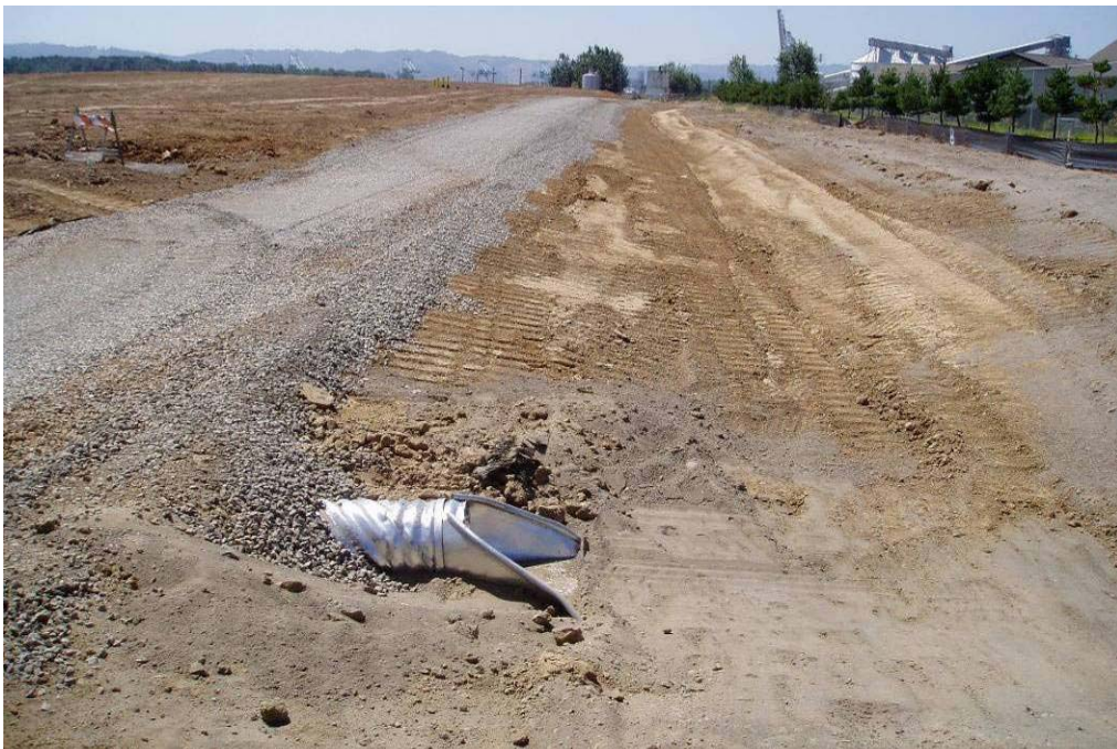
60043 July, 2004 – Gravel access road along north side of East Landfill. Culvert in foreground to transfer flow from drainage swale (sloping from background to foreground) to drainage swale on east side of landfill flowing to Columbia River.
