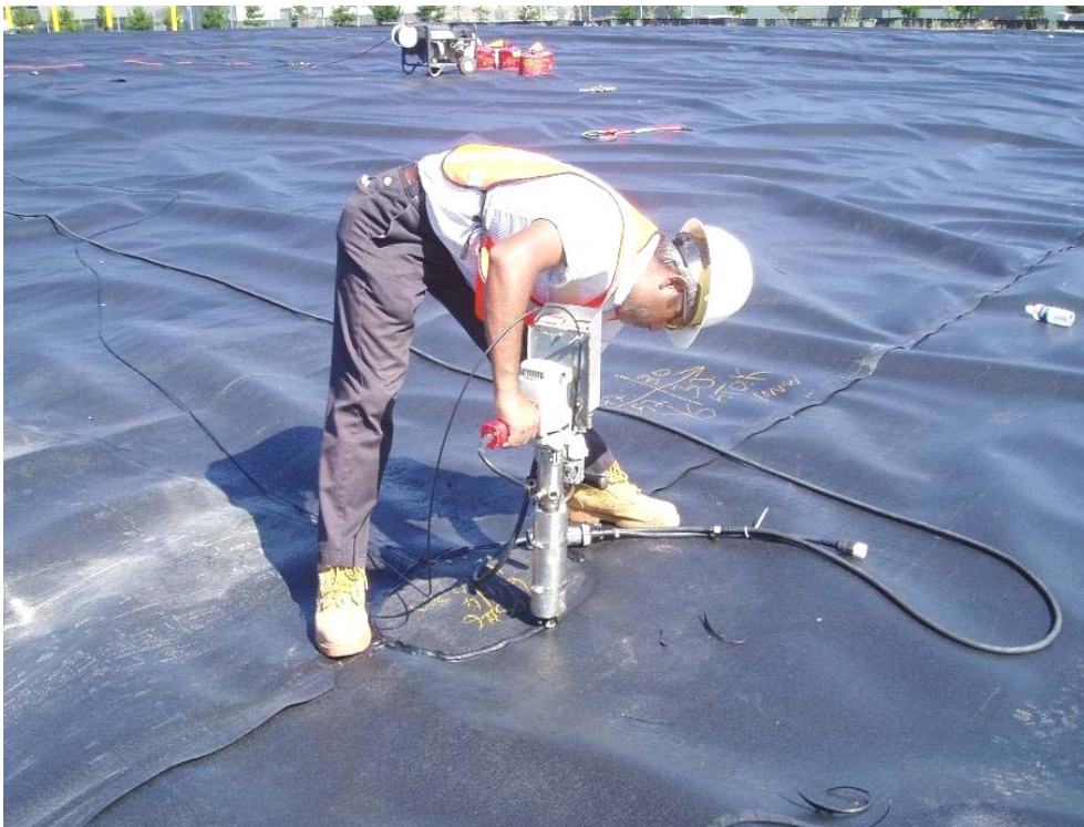
40181 June, 2004- Extrusion weld placed over end of air chamber test.
