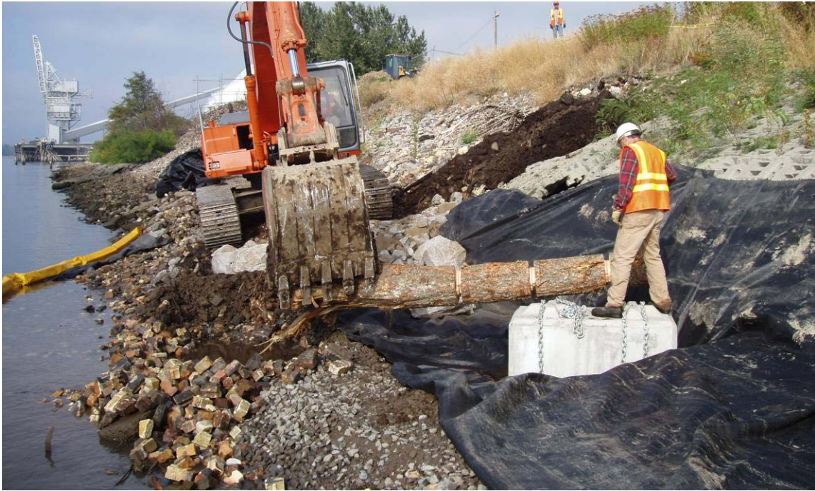
0605 October 6, 2006 – Installation of rootwad adjacent to ecology block. Looking west.
