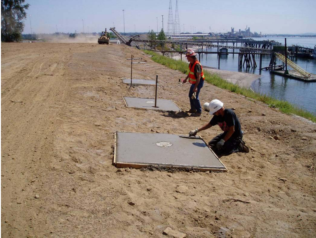
20058 August, 2004 – Laborers finishing concrete monitoring well pads. Looking east.
