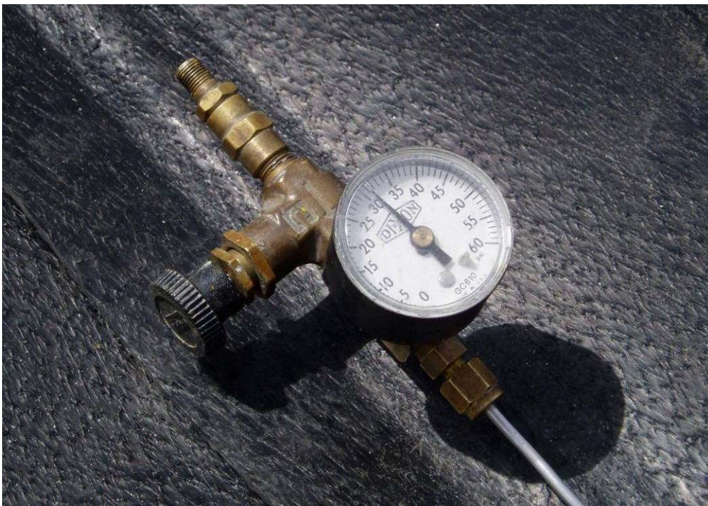
50083 May, 2004- Monitoring of air pressure in channel between welds with gauge.
