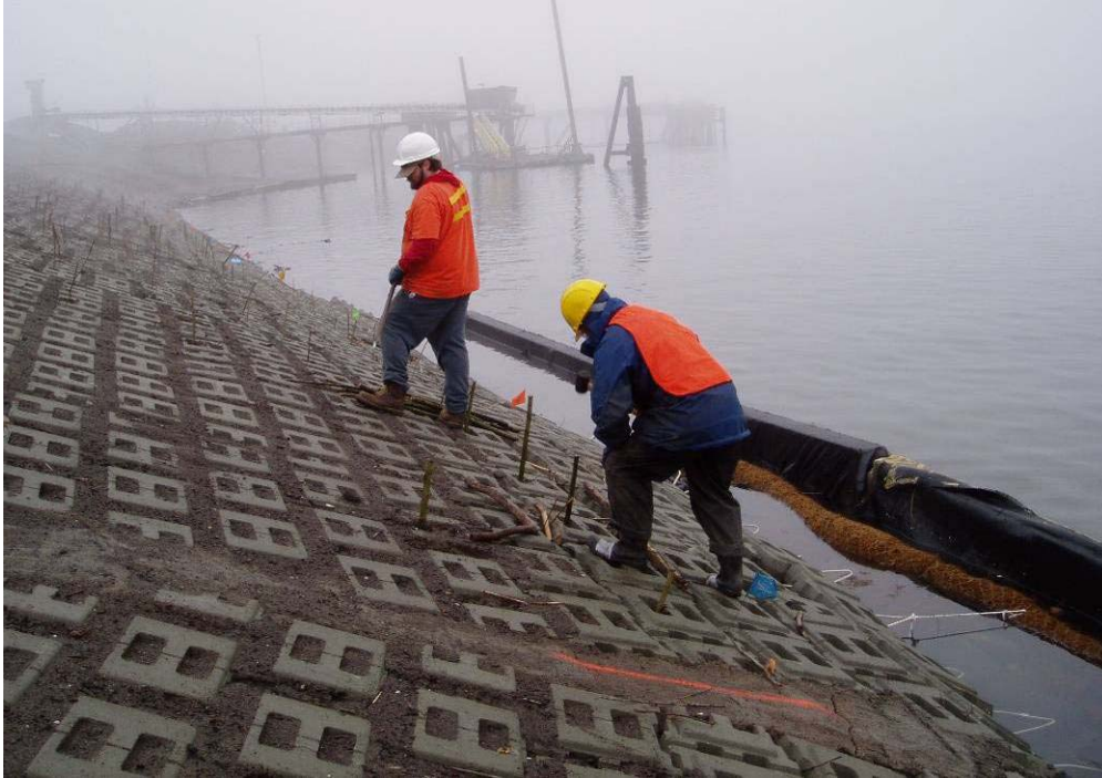
50011 December, 2003 – Marking of locations and driving of rods into subsoils through openings in 'Armorflex' panels prior to insertion of live stakes. Looking east.
