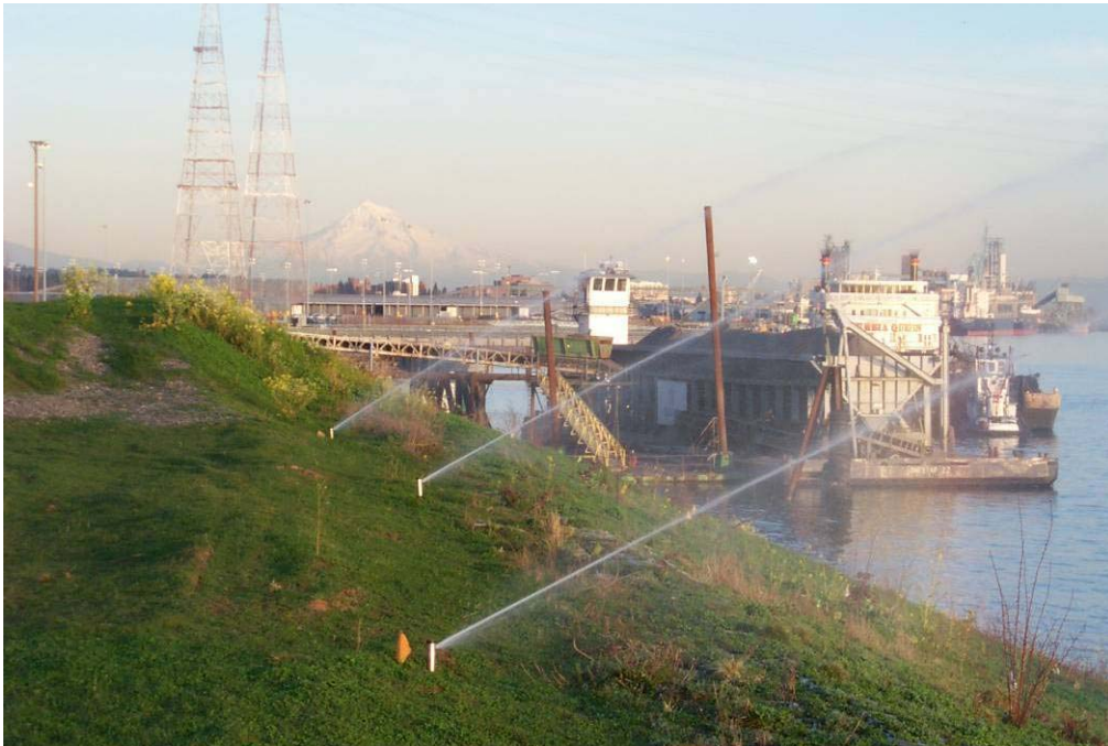
5208 March, 2005 – Active sprinkler system for maintaining vegetation within open space of 'Armorflex' revetment. Sprinkler heads spaced on 50 feet centers and designed to water 65 feet radius. Looking east.
