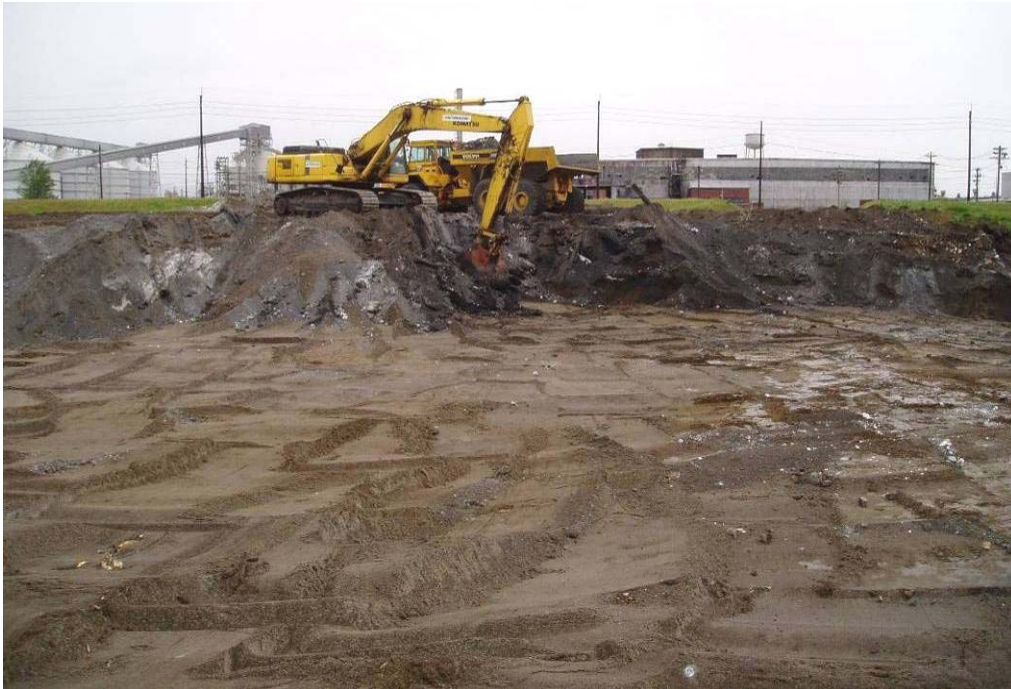
90061 April, 2004 – Excavation of Waste Soils from North 2 Landfill. Looking west.
