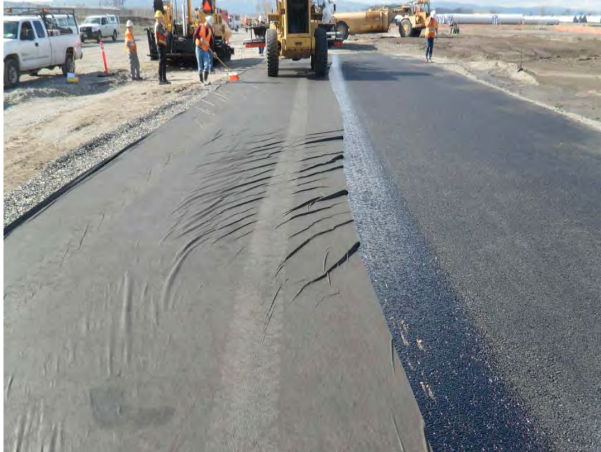
Photo 13 SPL Test Pad Geotextile Inerlayer Application 3/05/2010
