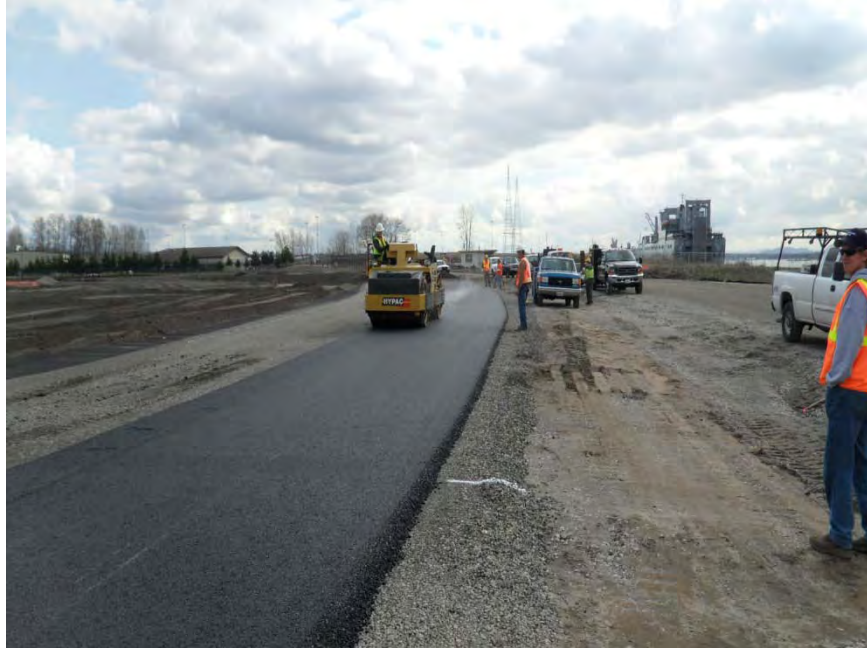
Photo 5 SPL Test Pad HMA Base Layer 2 1/2" Placement and Compaction 3/05/2010
