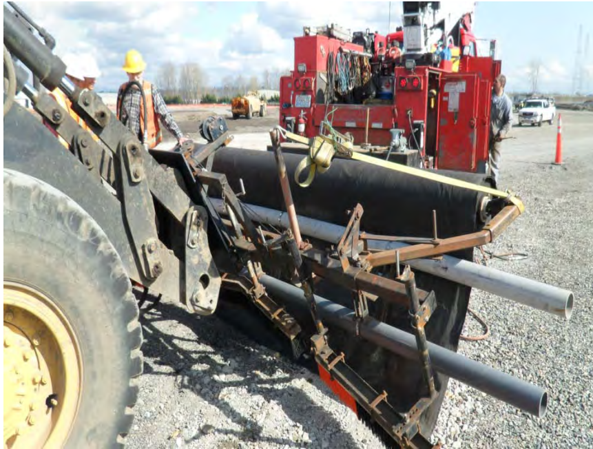
Photo 7 SPL Test Pad Geotextile Roll Placement Equipment 3/05/2010
