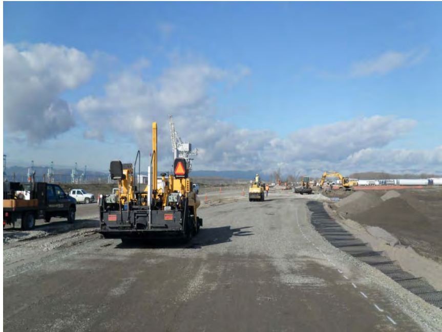
Photo 3 SPL Test Pad Subgrade Placement and Compaction 3/05/2010
