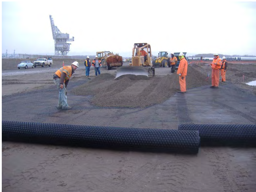
Photo 2 SPL Test Pad Triaxial Geogrid and Subgrade Installation 2/23/2010
