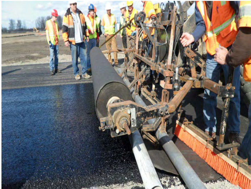
Photo 10 SPL Test Pad Geotextile Inerlayer Application 3/05/2010
