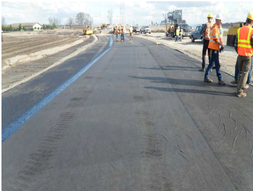
Photo 14 SPL Test Pad Geotextile Interlayer Application 3/05/2010
