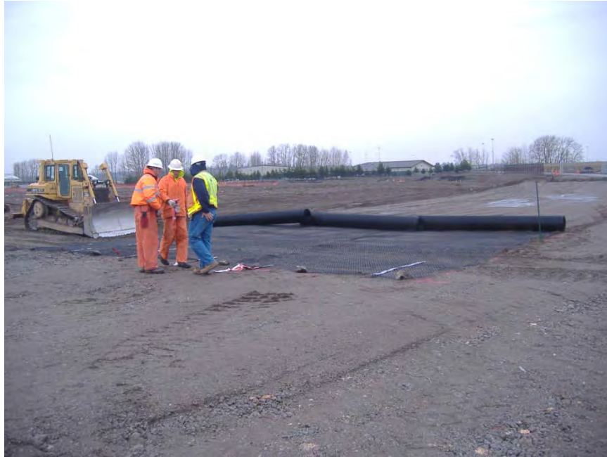
Photo 1 SPL Test Pad Triaxial Geogrid Installation 2/23/2010
