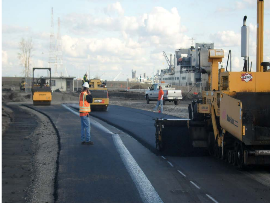
Photo 17 SPL Test Pad HMA Top Layer Application
