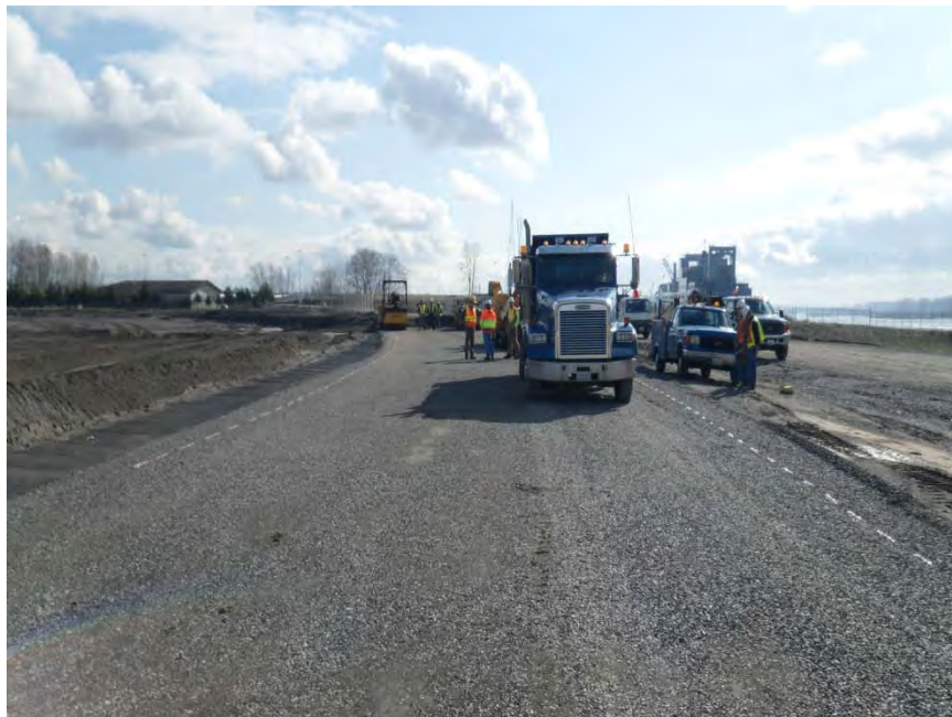
Photo 4 SPL Test Pad Subgrade Preparation 3/05/2010
