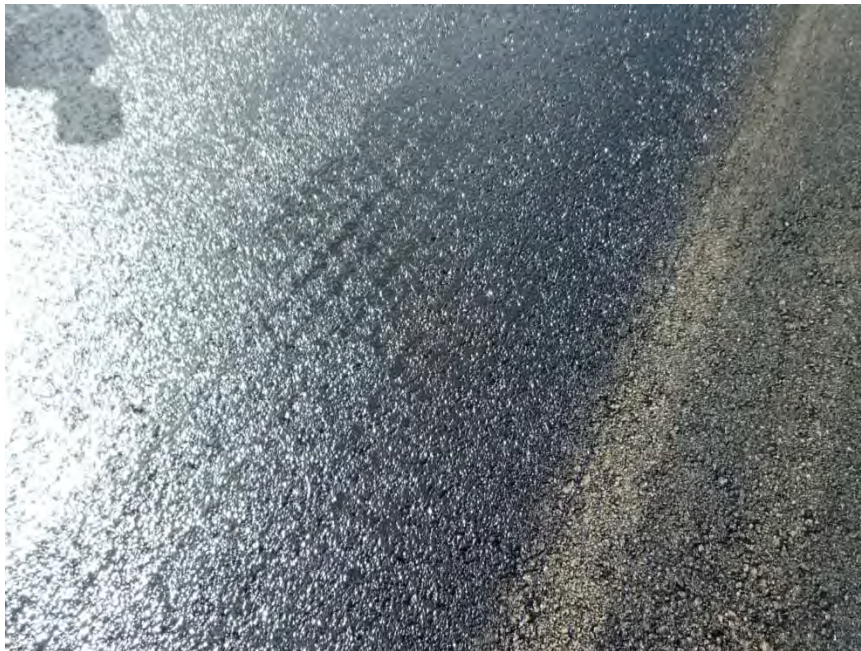
Photo 8 SPL Test Pad Tack Coat Application 3/05/2010
