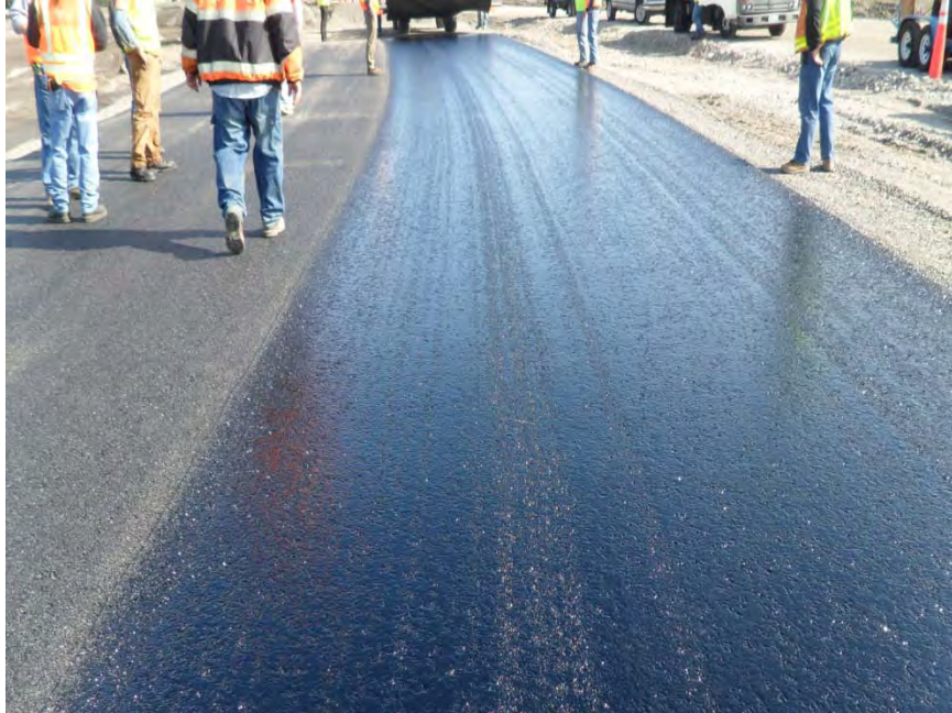
Photo 9 SPL Test Pad Tack Coat Application 3/05/2010
