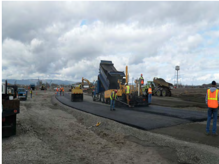
Photo 6 SPL Test Pad HMA Base Layer 2 1/2" Placement and Compaction 3/05/2010
