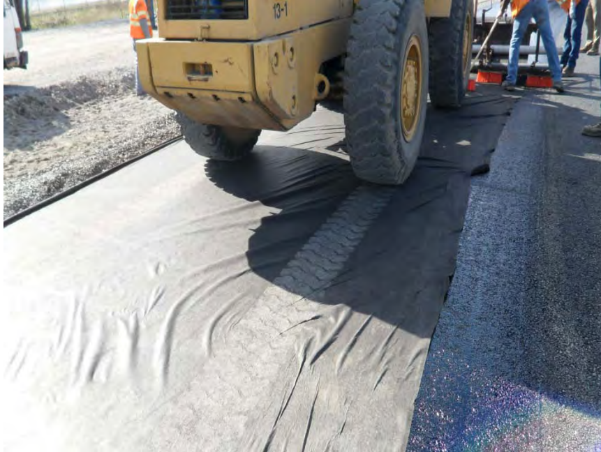
Photo 11 SPL Test Pad Geotextile Inerlayer Application 3/05/2010
