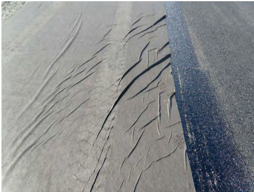
Photo 12 SPL Test Pad Geotextile Inerlayer Application 3/05/2010
