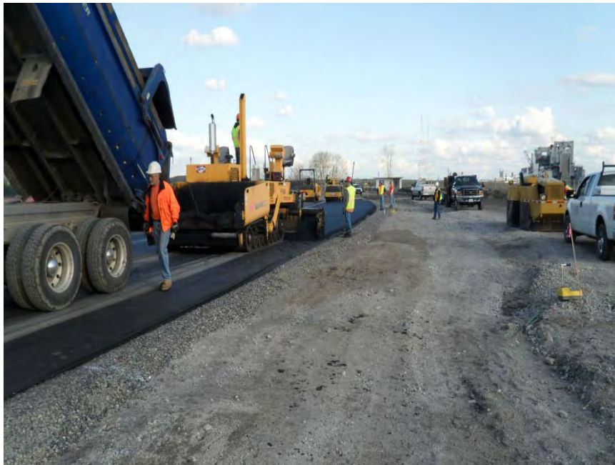
Photo 16 SPL Test Pad HMA Top Layer Application
