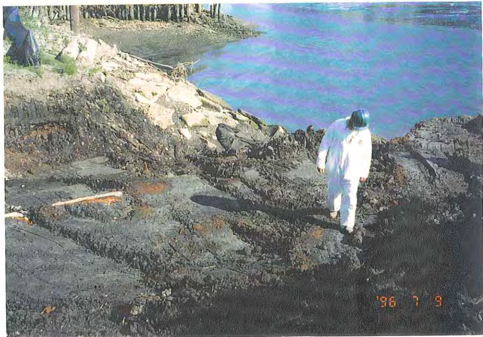
Excavation Below High Water Line Along Waterway
