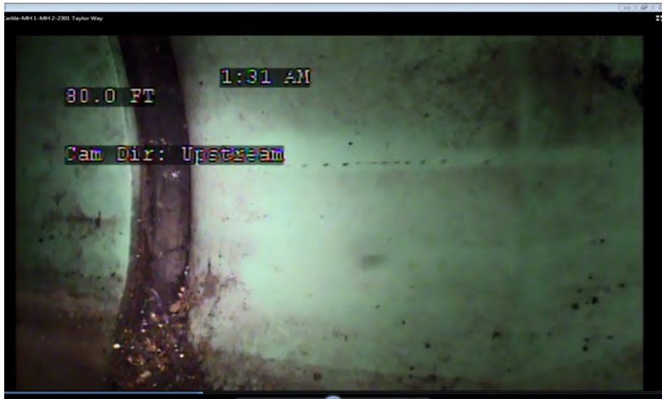
Photo #4 - 84 Feet Upstream of MH2 Showing Section of Pipe with an Incorrectly Set Gasket
