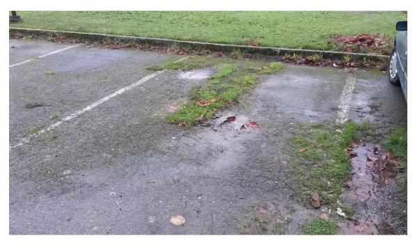
Photo Location 1 showing pavement deterioration (1st view), 12/5/16 site inspection
