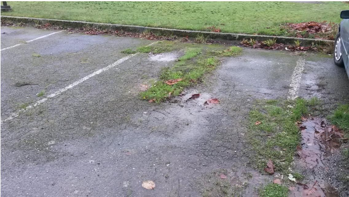
Photo Location 1 showing pavement deterioration (1<sup>st</sup> view), 12/5/16 site inspection
