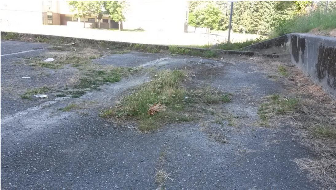
Photo Location 1 showing pavement deterioration, 6/7/16 site inspection
