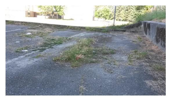
Photo Location 1 showing pavement deterioration, 6/7/16 site inspection
