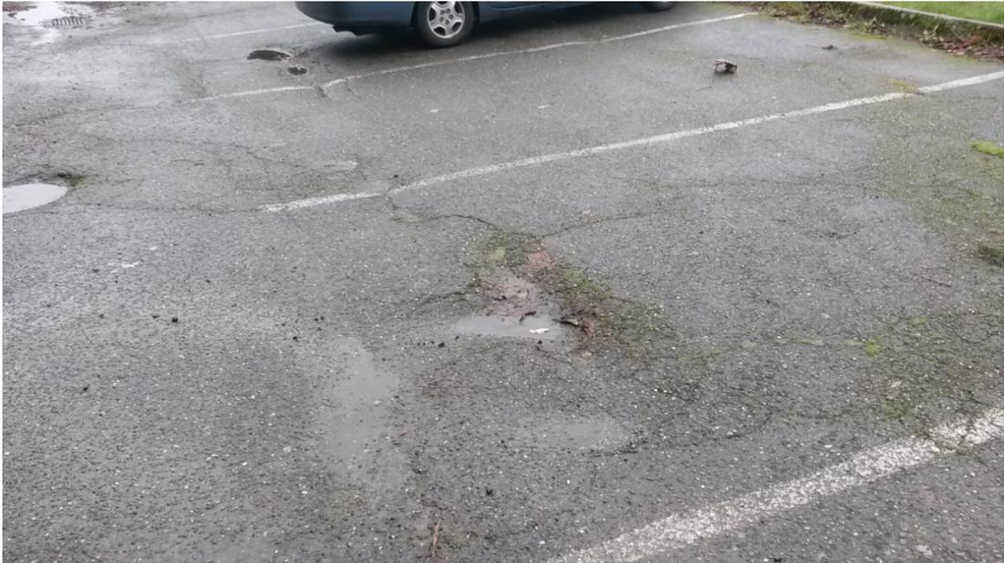
Photo Location 1 showing pavement deterioration (2nd view), 12/5/16 site inspection
