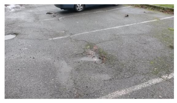
Photo Location 1 showing pavement deterioration (2nd view), 12/5/16 site inspection
