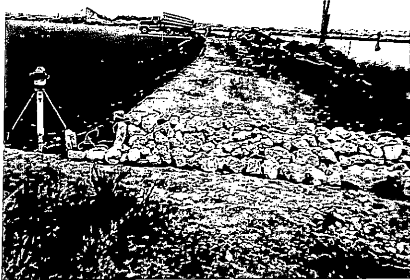
5-27-99 QC east edge drainage trench. note: Background; filling/forming drainage trench with asphalt.
