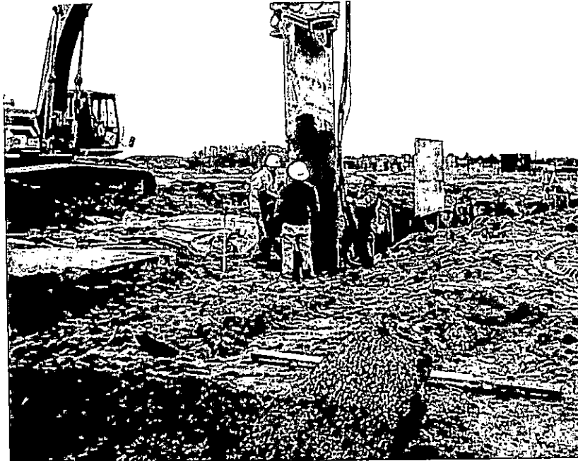
1-11-99 Removing Panel 202. Background - Successfully installed panes
