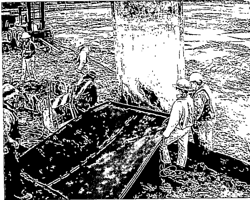
3-25-99 Last panel # 005 installation setup at 6+42 (note weld in middle of panel).
