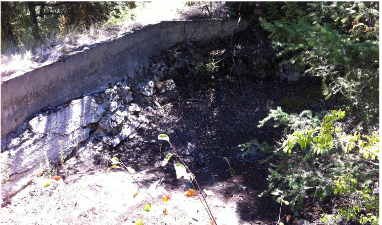
Small reservoir area, with a concrete wall across a low notch in the bedrock formation.
