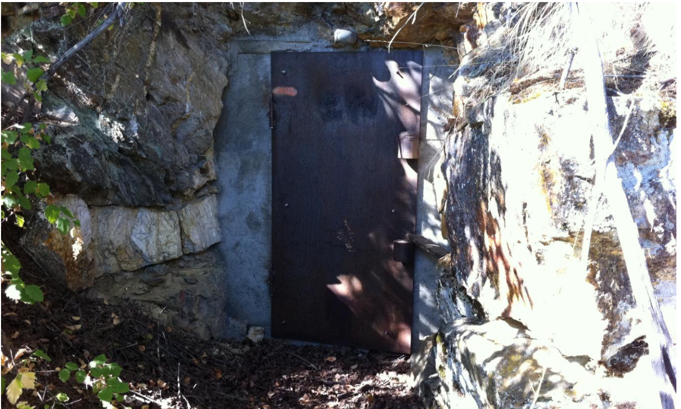
Concrete and steel door of the old powder magazine.
