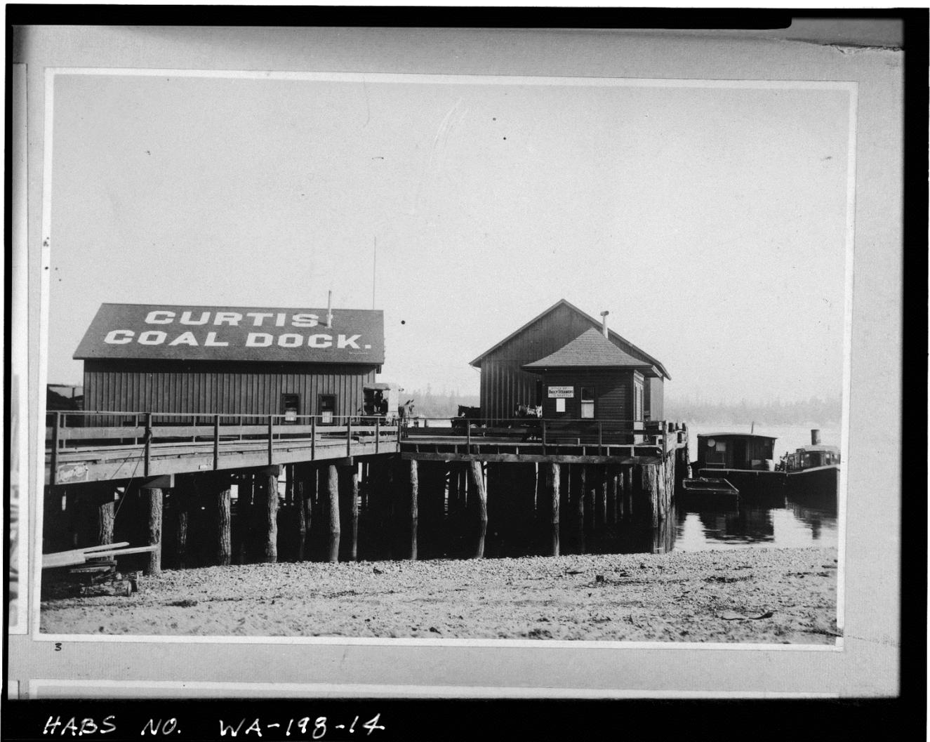
Photocopy of photograph (Original print, Anacortes Museum.) Published in the Anacortes American, April 1907. Tacoma Engineering Company, Photographer. View to the north. On the right; early ticket office, south facade; behind it, a warehouse, east section of the present building; on the left, the original freight warehouse, the west section of the present building. Note wharf configuration in front of Ticket Office. - Curtis Wharf, O & Second Streets, Anacortes, Skagit County, WA
