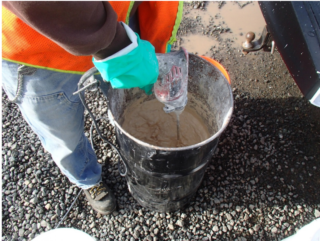
Photograph 17. Mixing of oxygen-releasing compound.
