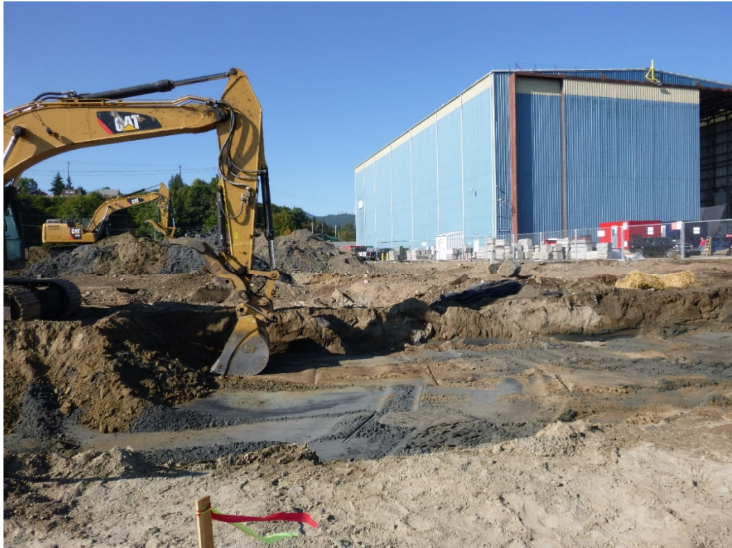
Photograph 5. Excavation Area 5, week of August 17, 2015.
