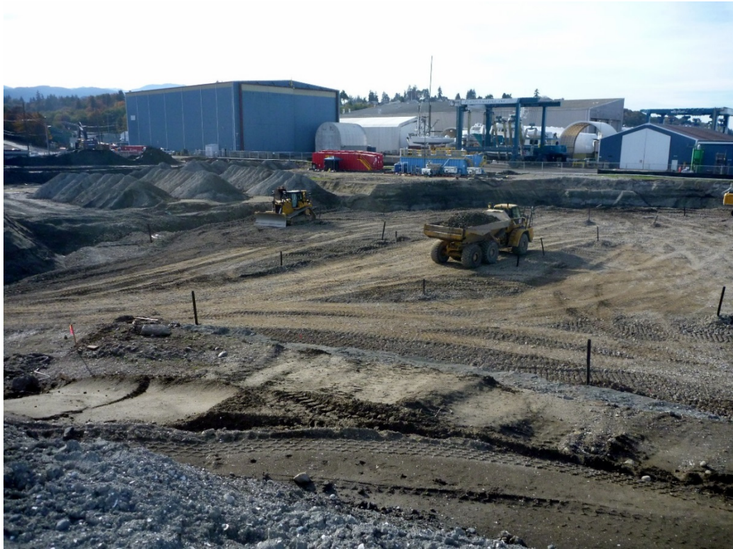
Photograph 21. Excavation Area 6, week of October 12, 2015.
