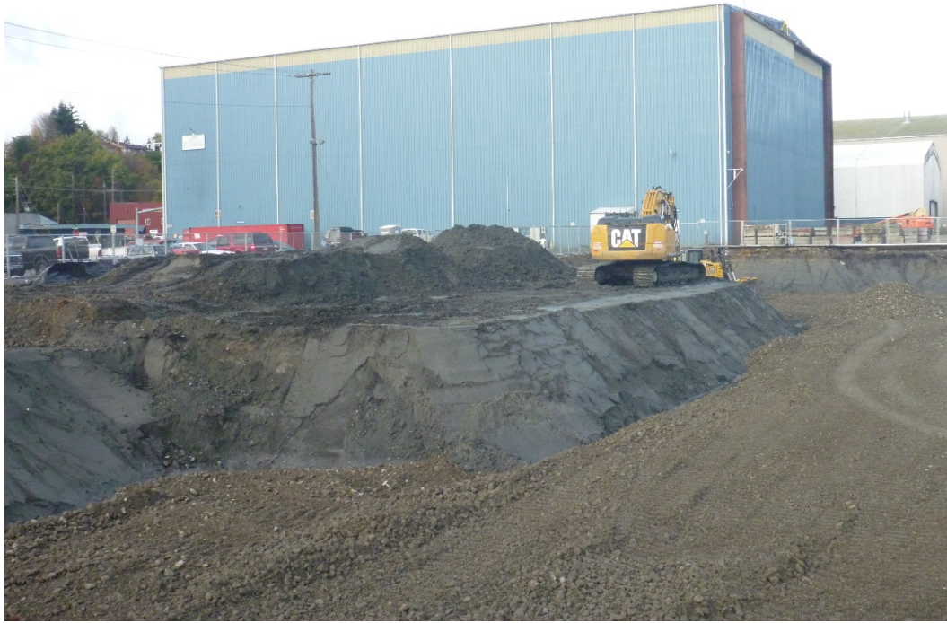
Photograph 25. Excavation Area 5, week of October 26, 2015.
