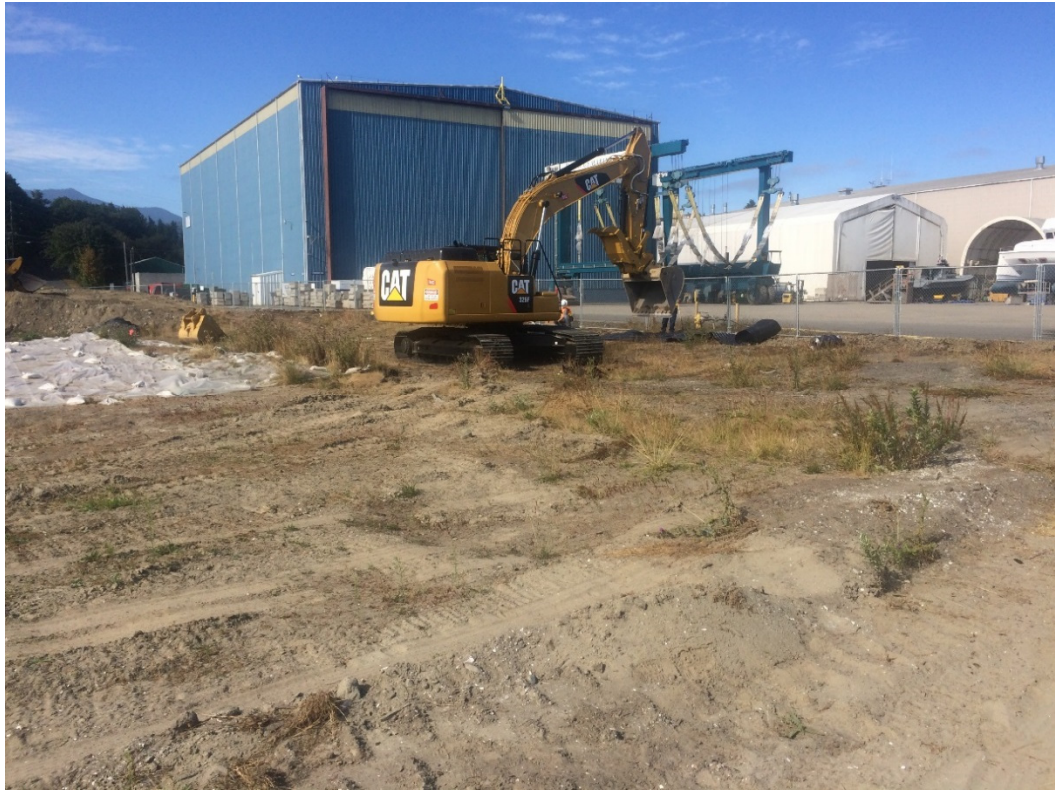
Photograph 1. Excavation Area 5, week of August 3, 2015.
