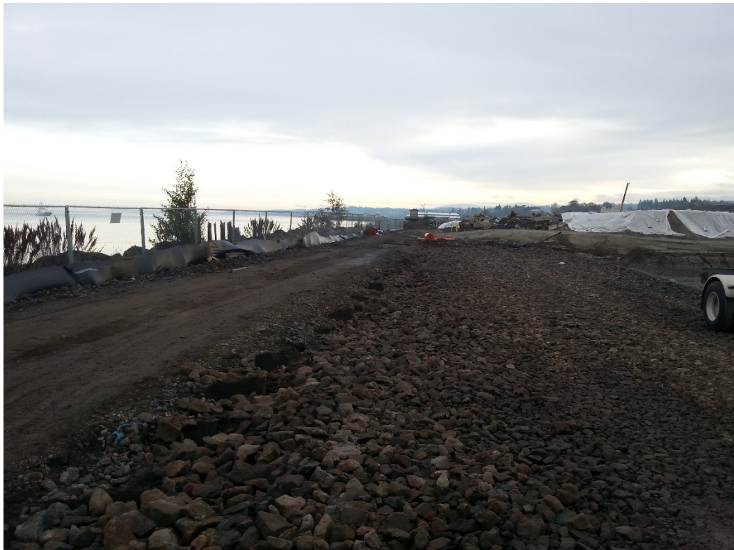
Photograph 36. Excavation Area 6, week of November 21, 2015.
