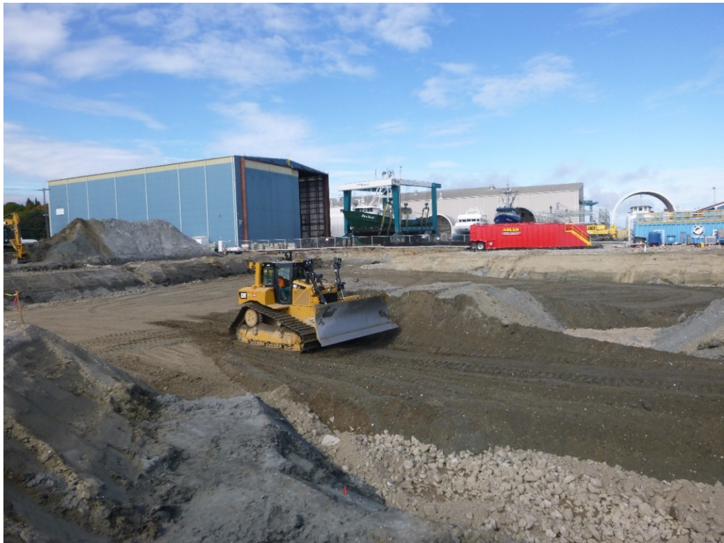
Photograph 12. Excavation Area 5, week of September 14, 2015.
