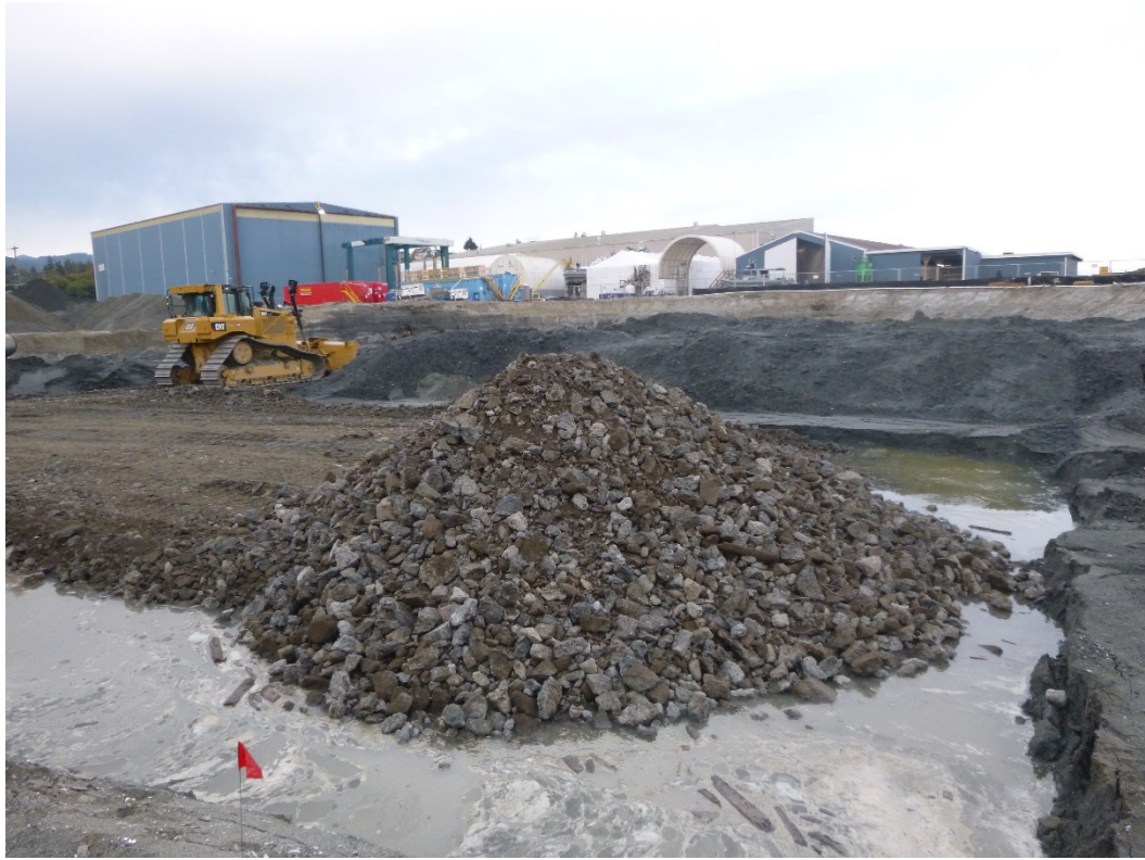
Photograph 17. Excavation Area 6, week of October 5, 2015.
