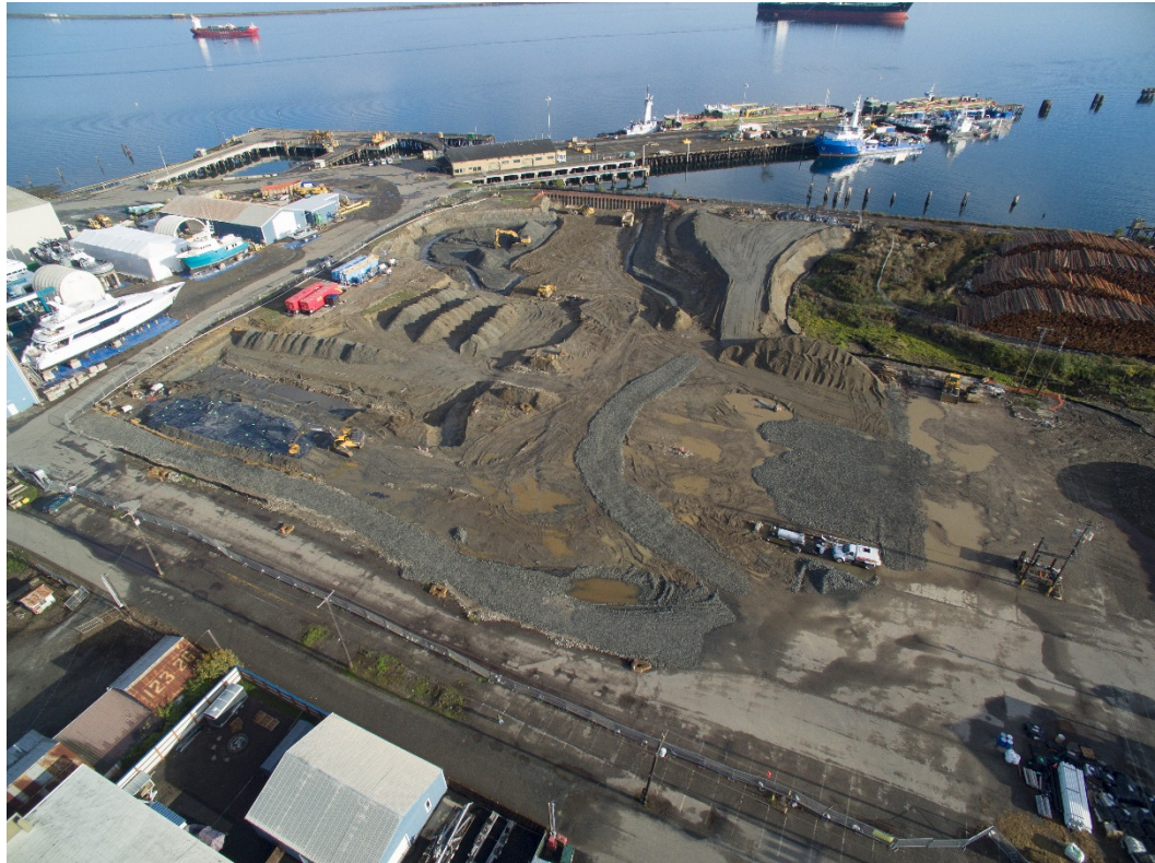
Photograph 19. Aerial photo of site, week of October 12, 2015.
