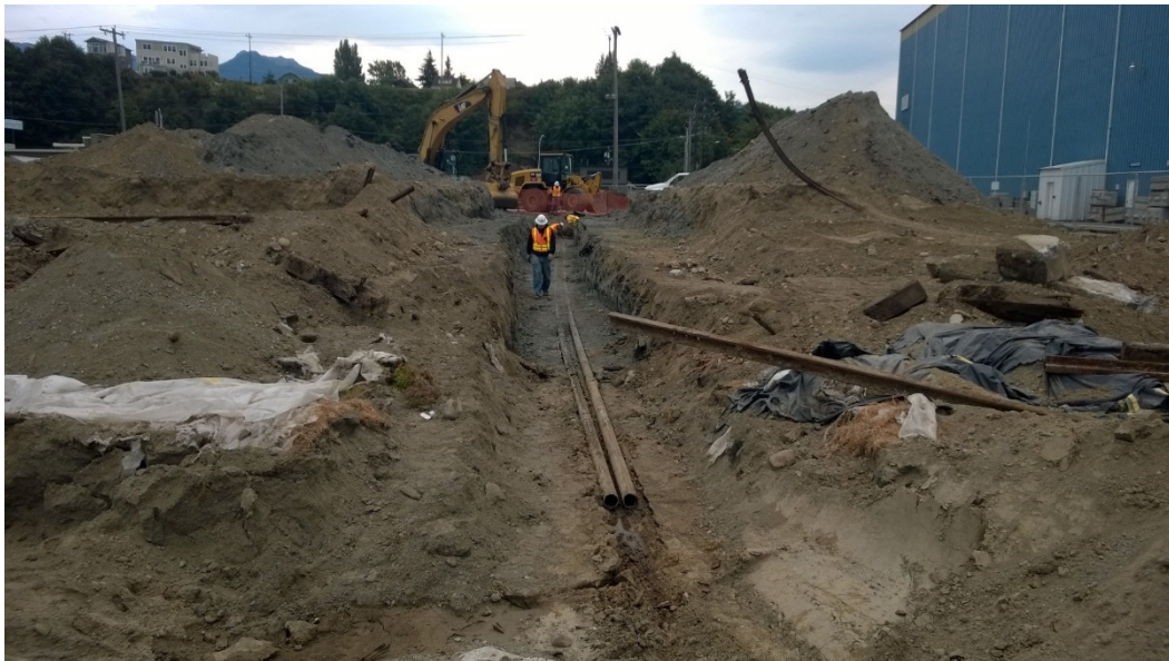
Photograph 2. Removal of Pipeline 8.
