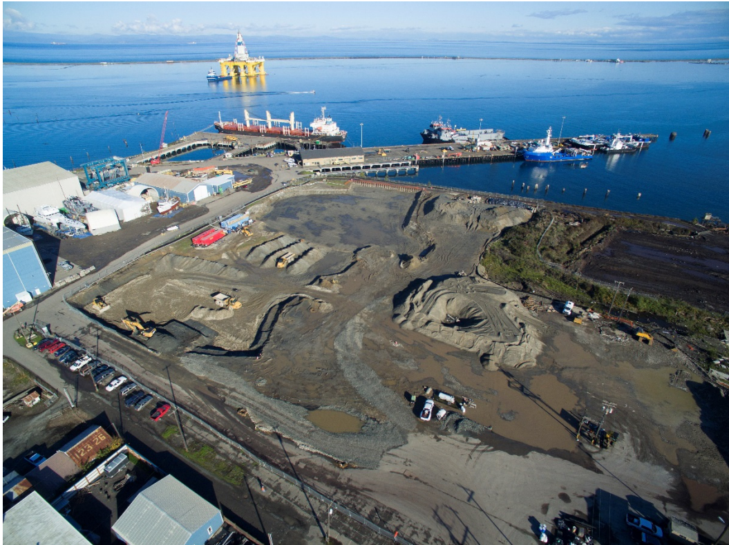
Photograph 26. Aerial photo of site, week of November 2, 2015.
