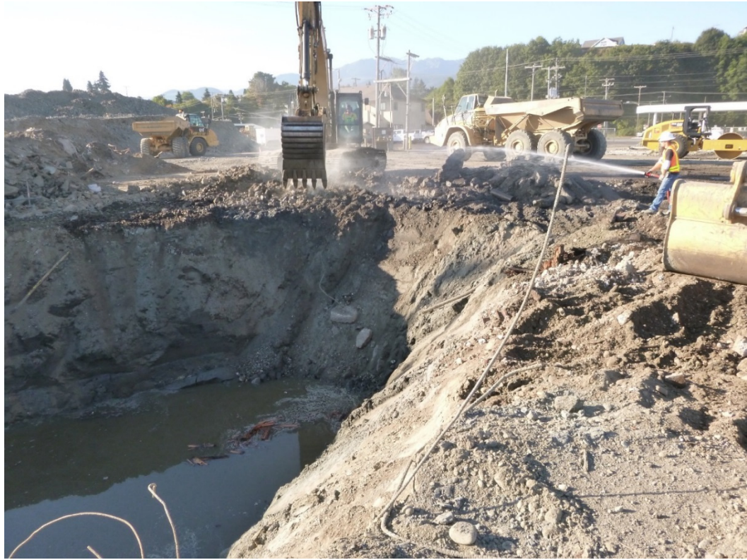
Photograph 7. BMP; watering to reduce dust during excavation.
