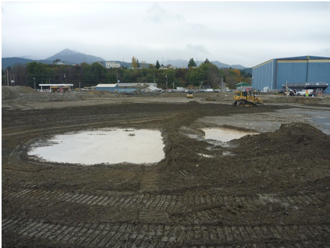
Photograph 32. Excavation Area 5, week of November 9, 2015.
