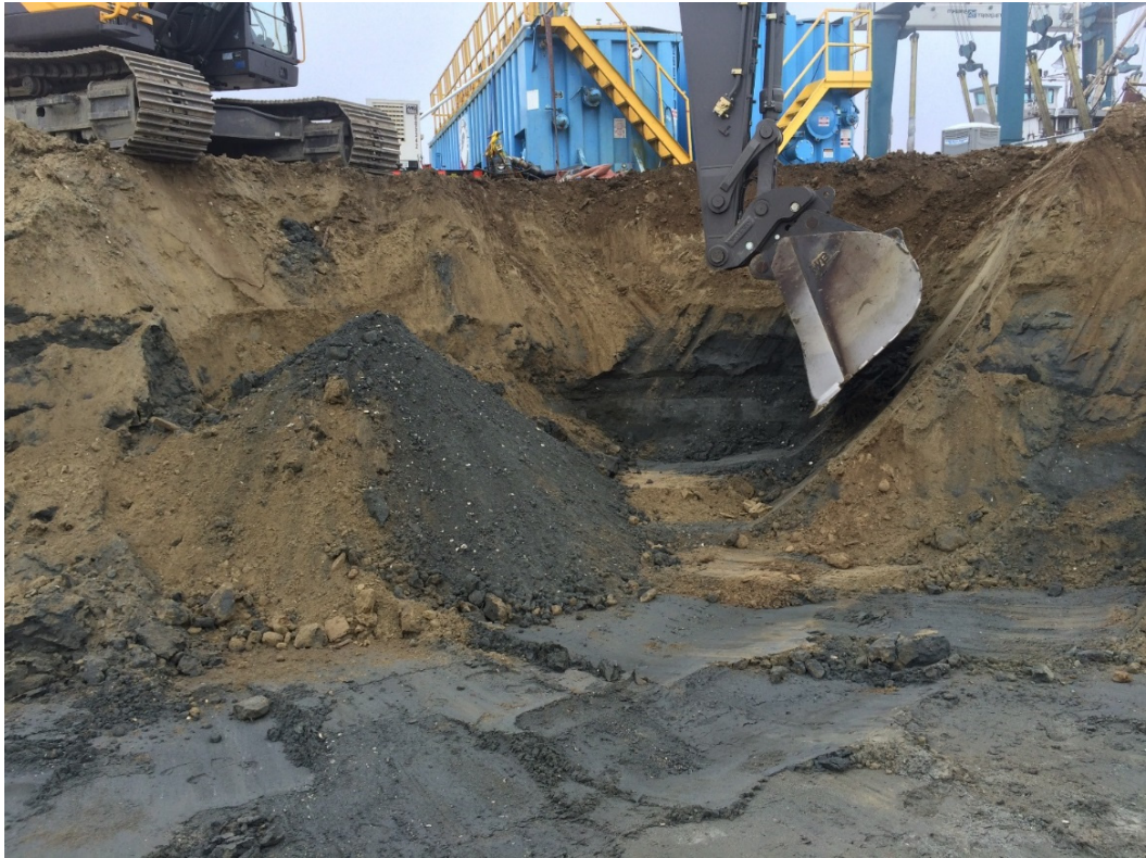
Photograph 15. Extended excavation of contaminated sidewall in Excavation Area 6.
