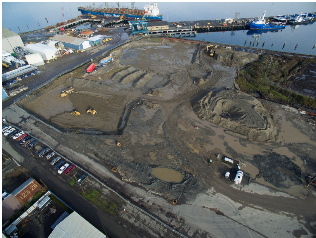
Photograph 30. Aerial photo of site, week of November 9, 2015.
