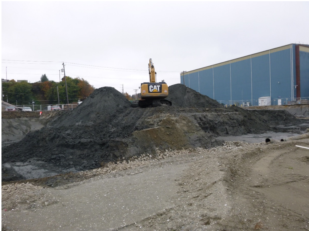
Photograph 24. Excavation Area 5, week of October 19, 2015.
