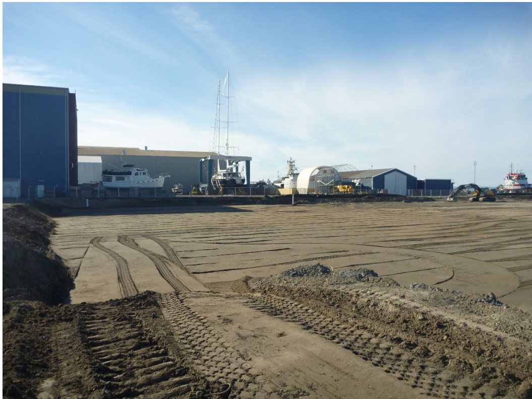
Photograph 40. Final grade of Excavation Area 5, week of May 9, 2016.
