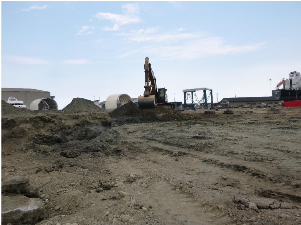
Photograph 4. Excavation Area 6, week of August 10, 2015.
