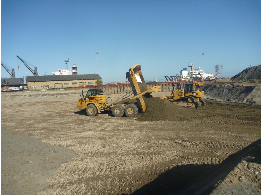
Photograph 23. Excavation Area 6, week of October 19, 2015.
