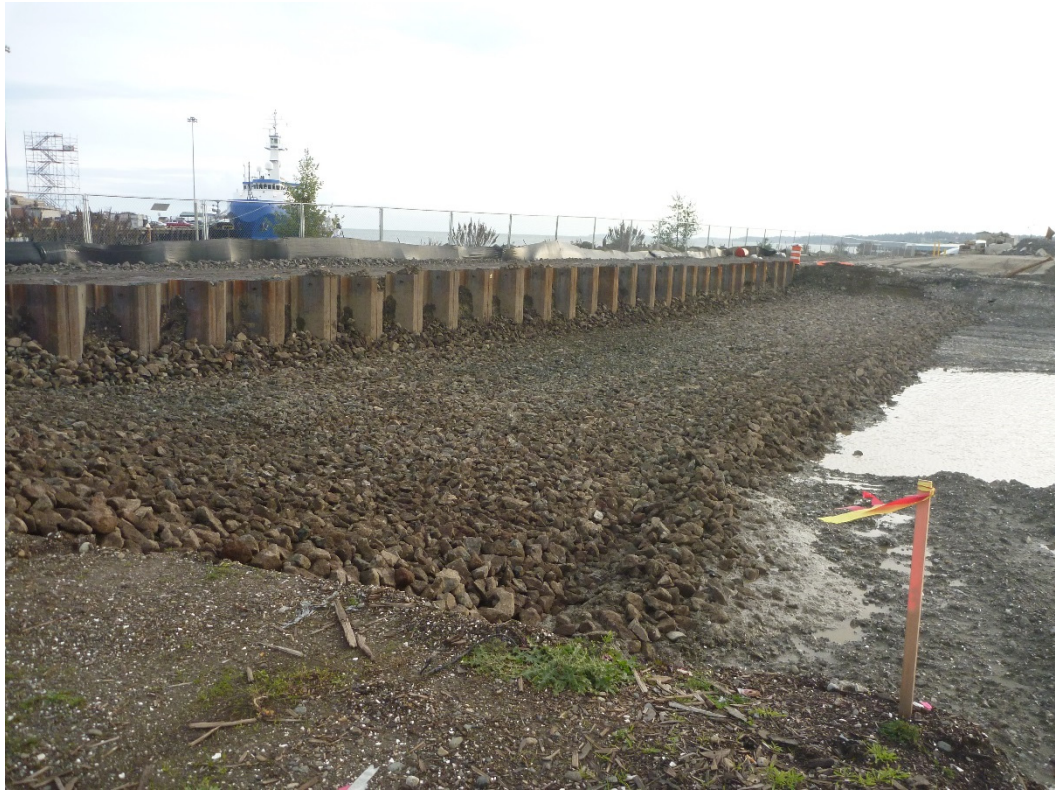
Photograph 35. Excavation Area 6, week of November 16, 2015.
