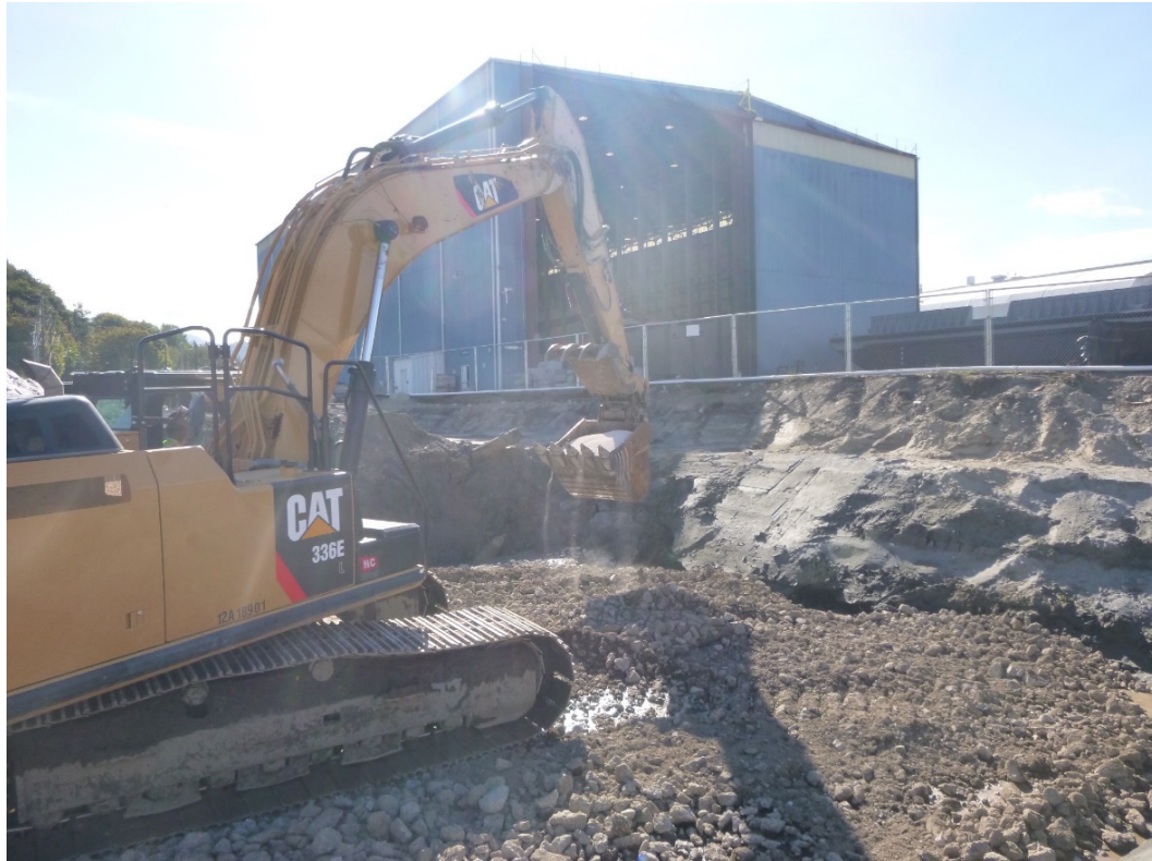
Photograph 11. Spreading of bioamendment in Excavation Area 5.
