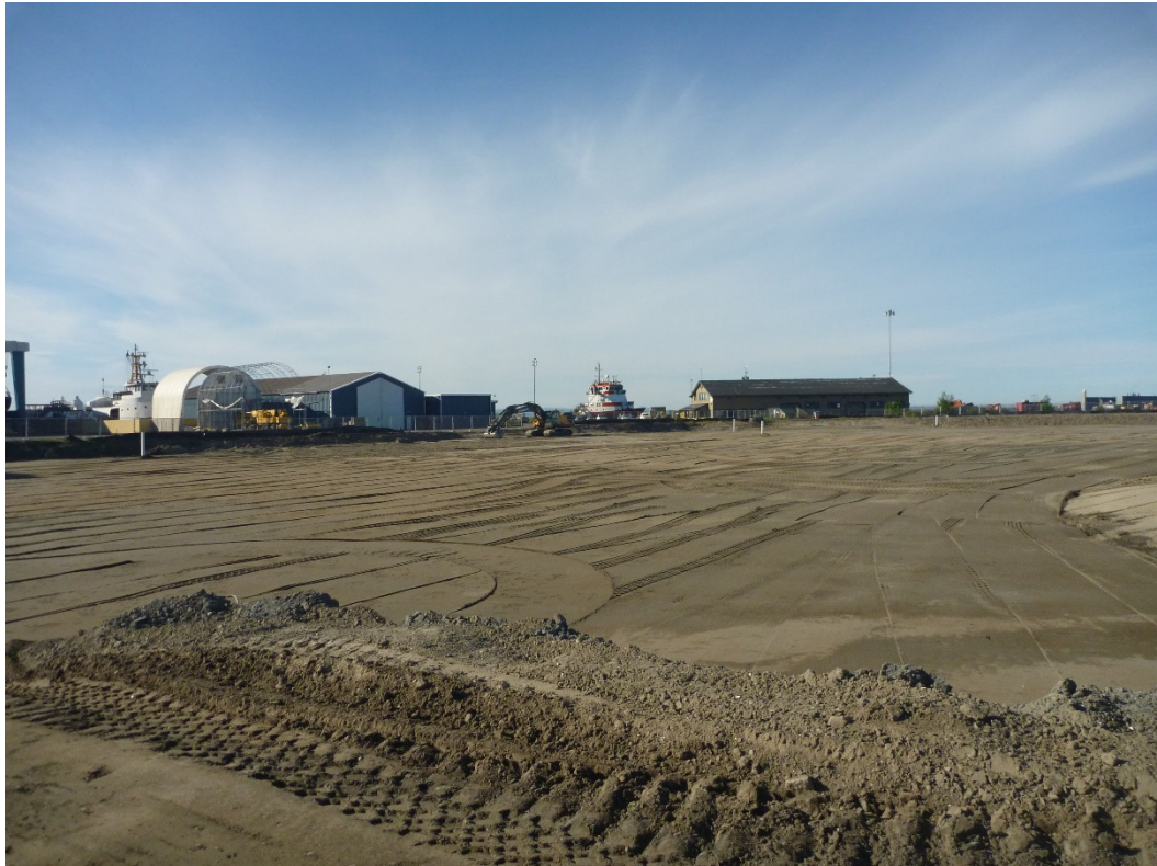
Photograph 39. Final grade of Excavation Area 6, week of May 9, 2016.
