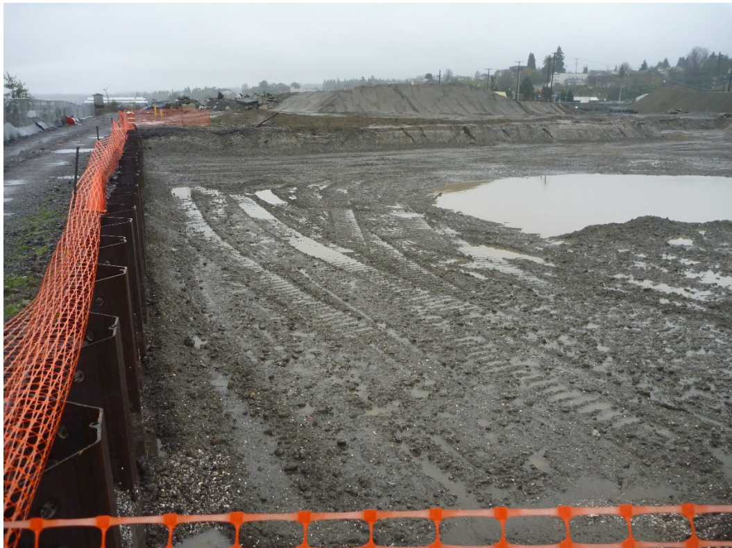
Photograph 34. Excavation Area 6, week of November 13, 2015.
