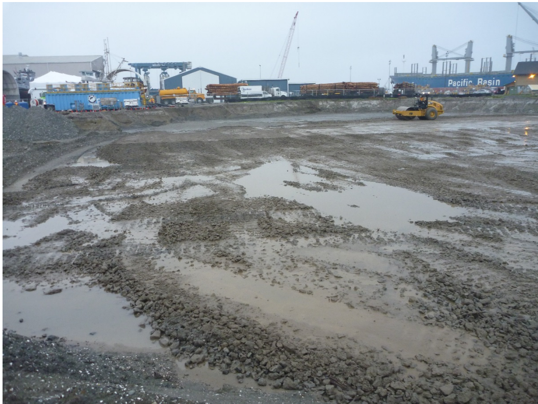
Photograph 28. Excavation Area 6, week of November 2, 2015.
