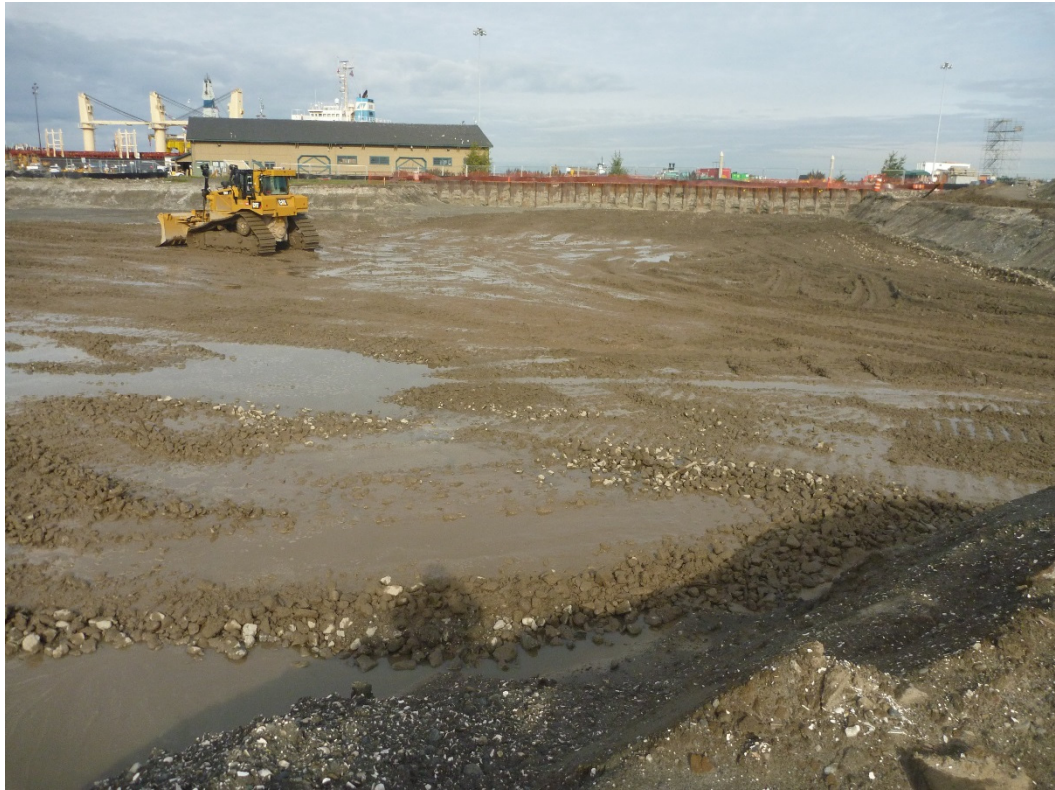
Photograph 27. Excavation Area 6, week of November 2, 2015.
