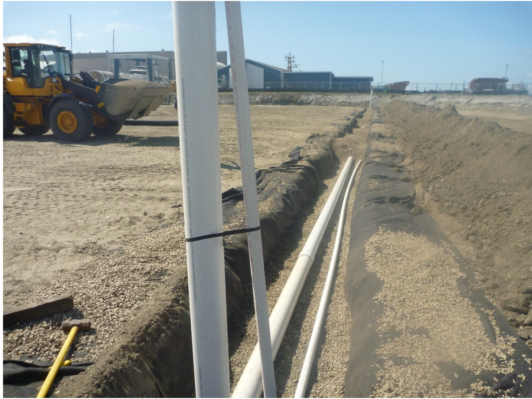
Photograph 19. Installation of infiltration gallery.
