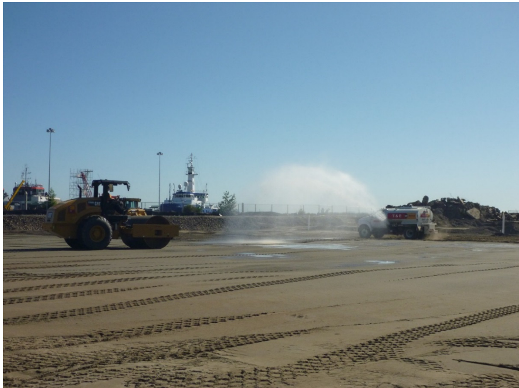
Photograph 20. Rolling backfilled surface.
