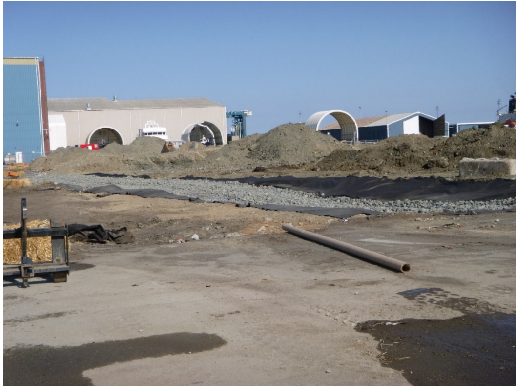
Photograph 5. Installation of wheel wash.
