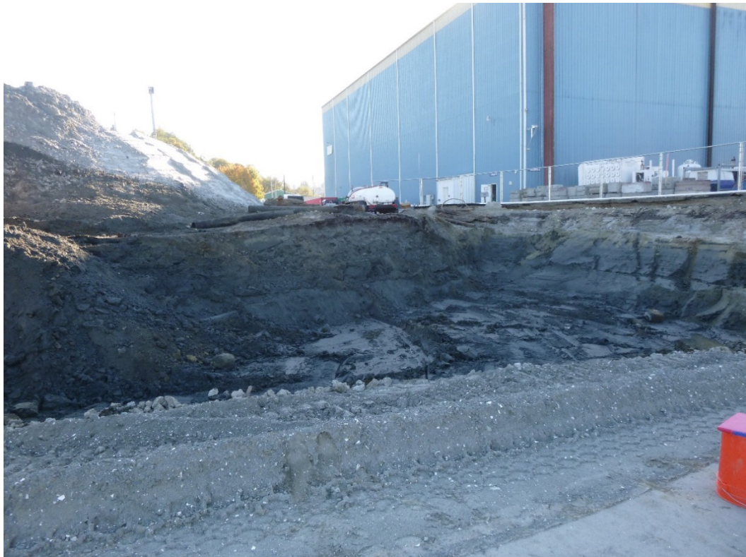
Photograph 16. Excavation Area 5, week of September 28, 2015.
