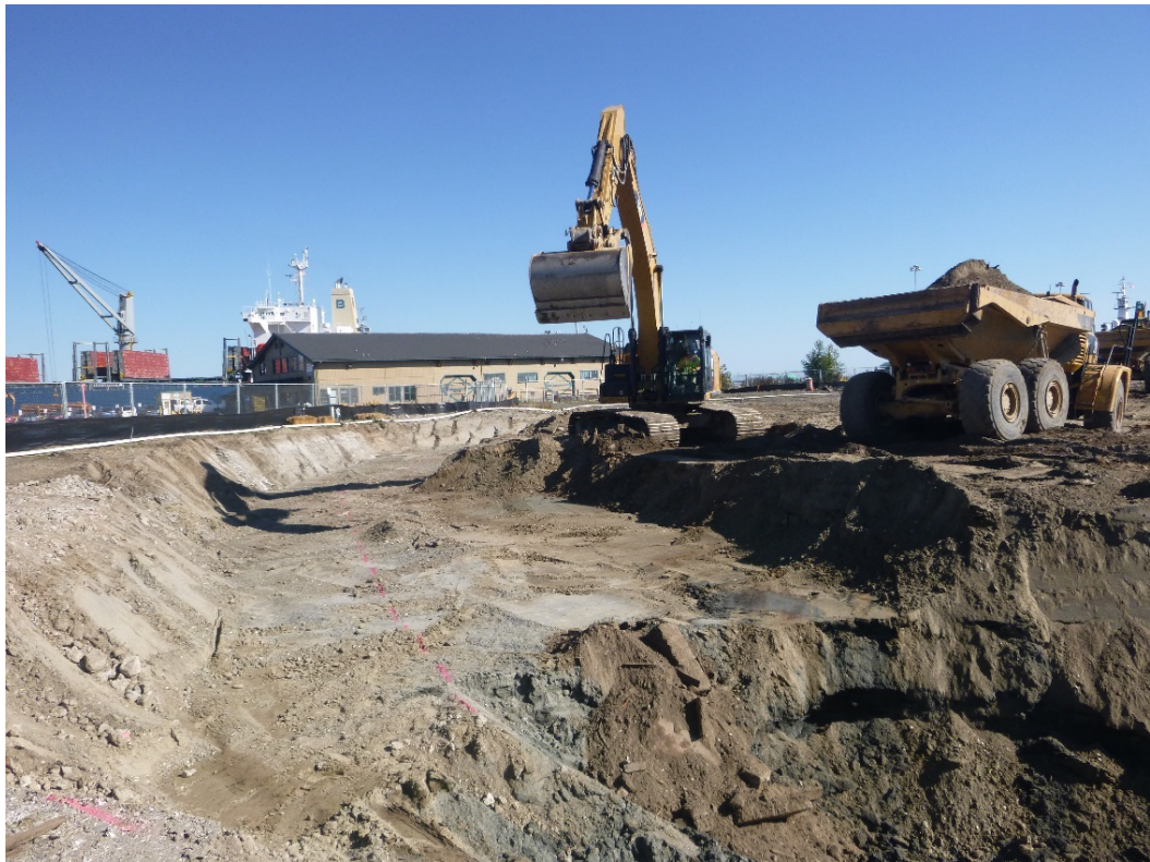
Photograph 10. Excavation Area 6, week of September 7, 2015.
