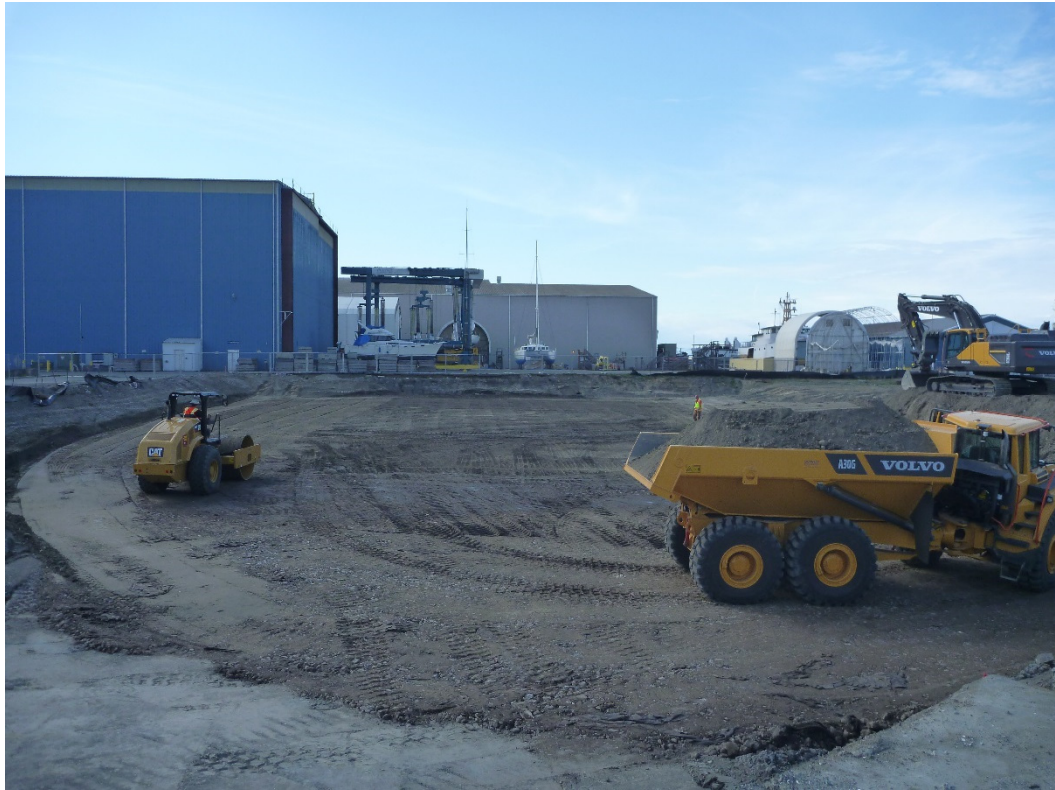
Photograph 37. Excavation Area 5, week of April 25, 2016.
