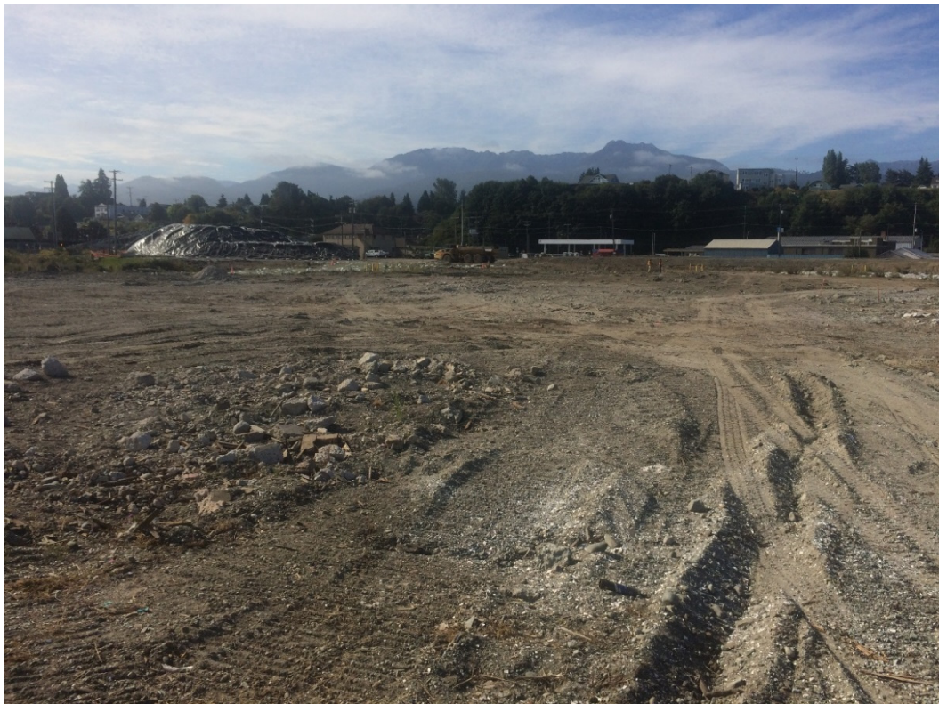
Photograph 2. Excavation Area 5, week of August 3, 2015.
