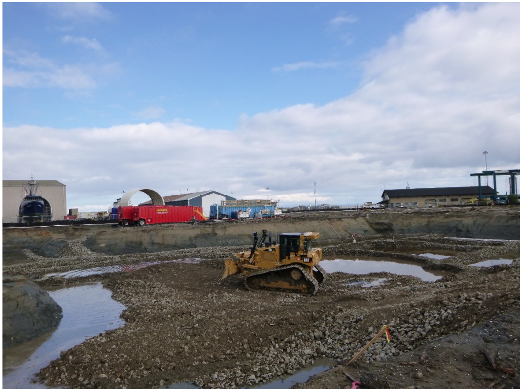
Photograph 8. Excavation Area 5, week of August 31, 2015.
