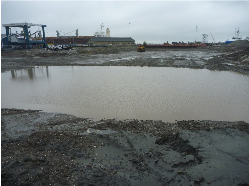
Photograph 33. Excavation Area 6, week of November 3, 2015.
