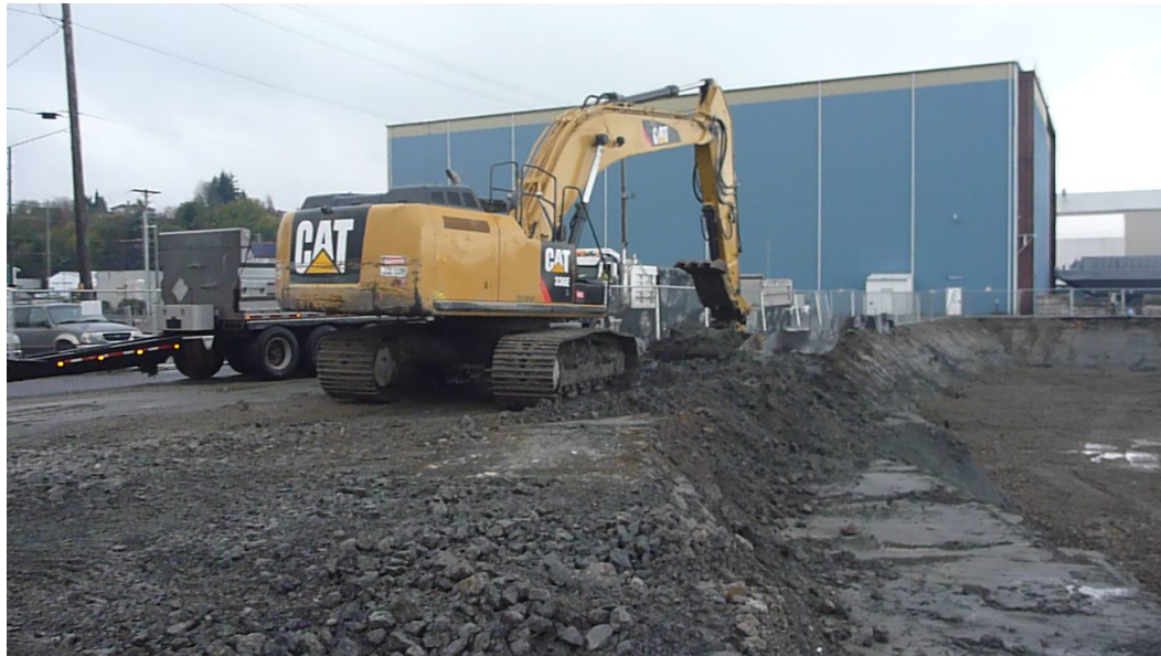
Photograph 29. Excavation Area 5, week of November 2, 2015.
