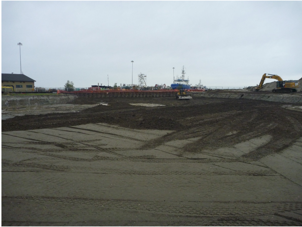
Photograph 31. Excavation Area 6, week of November 9, 2015.
