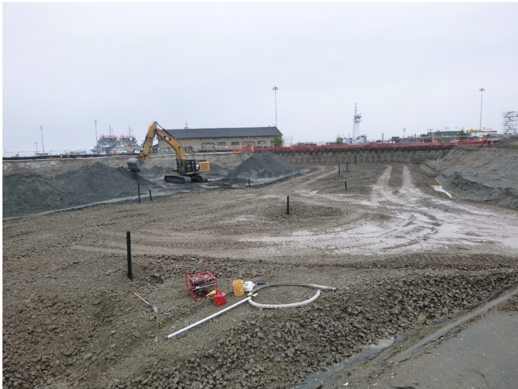
Photograph 18. Excavation Area 6, week of October 5, 2015.
