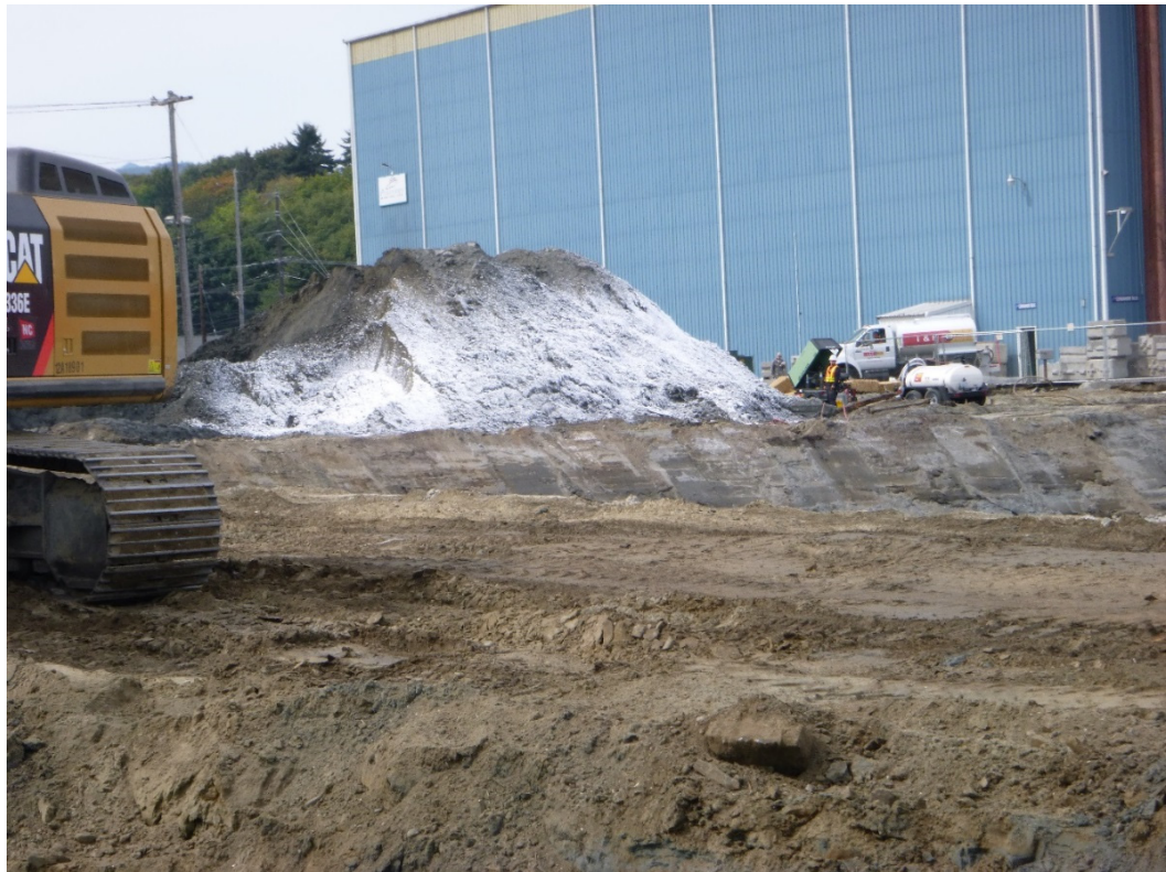
Photograph 8. Foam applied to stockpiles to address odor complaint.
