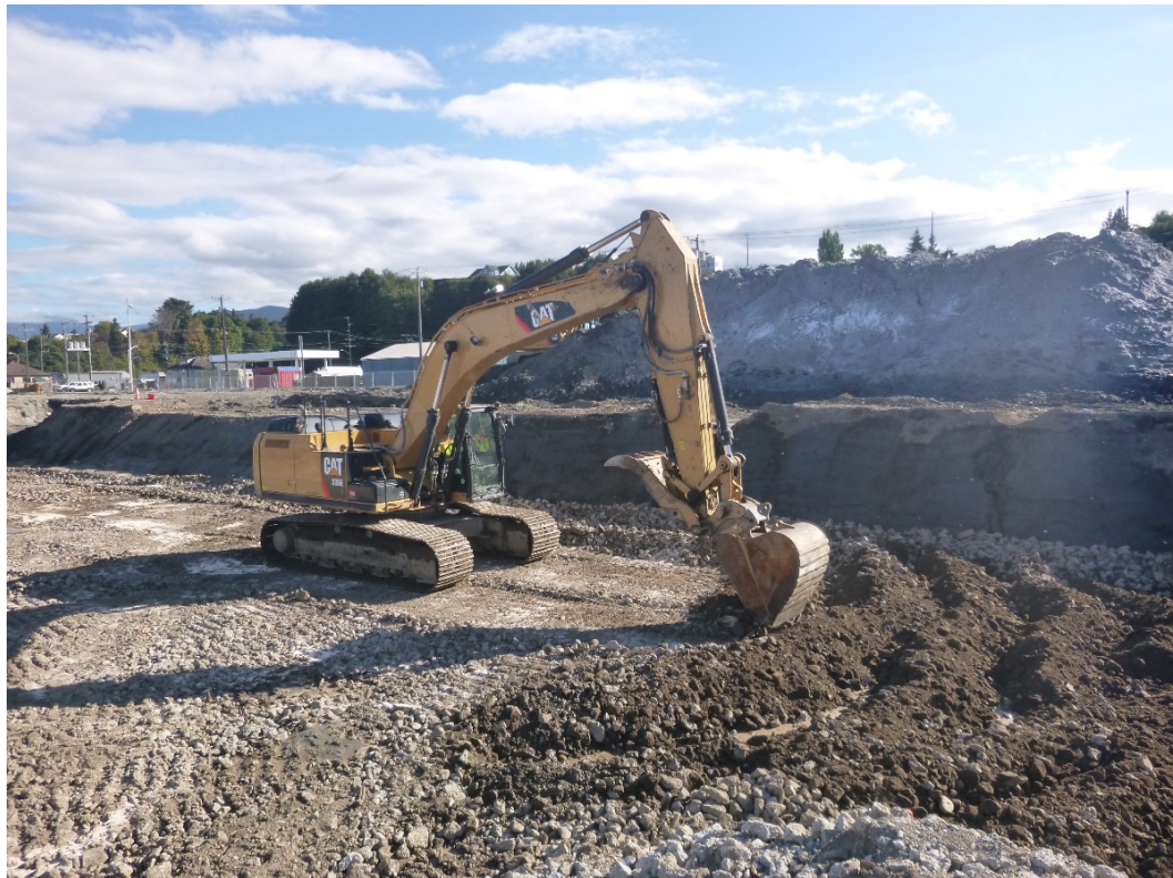
Photograph 12. Tilling of bioamendment in Excavation Area 5.
