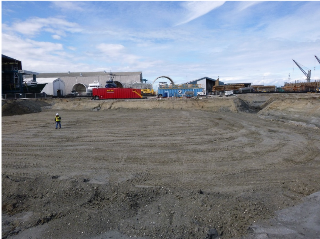
Photograph 13. Excavation Area 6, week of September 14, 2015.
