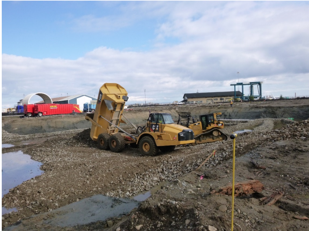
Photograph 9. Example of base fill in Excavation Area 5.
