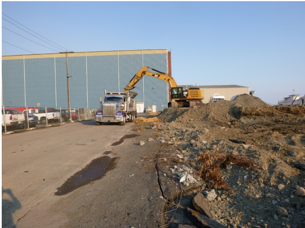
Photograph 6. Loading trucks for off-site disposal of contaminated soil.
