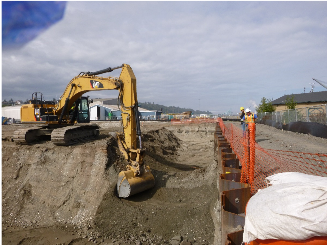
Photograph 11. Excavation Area 5, week of September 14, 2015.
