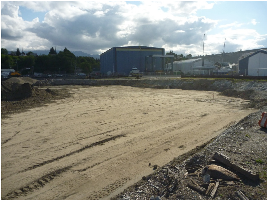
Photograph 38. Excavation Area 5, week of April 25, 2016.
