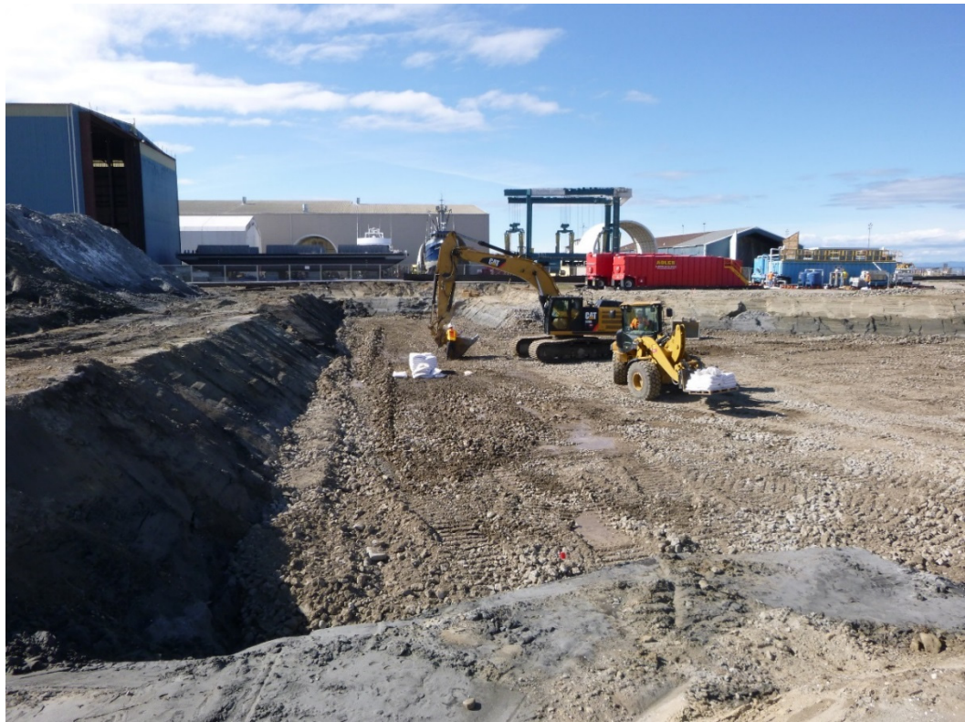
Photograph 10. Application of bioamendment in Excavation Area 5.
