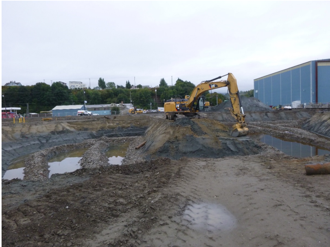
Photograph 7. Excavation Area 5, week of August 24, 2015.
