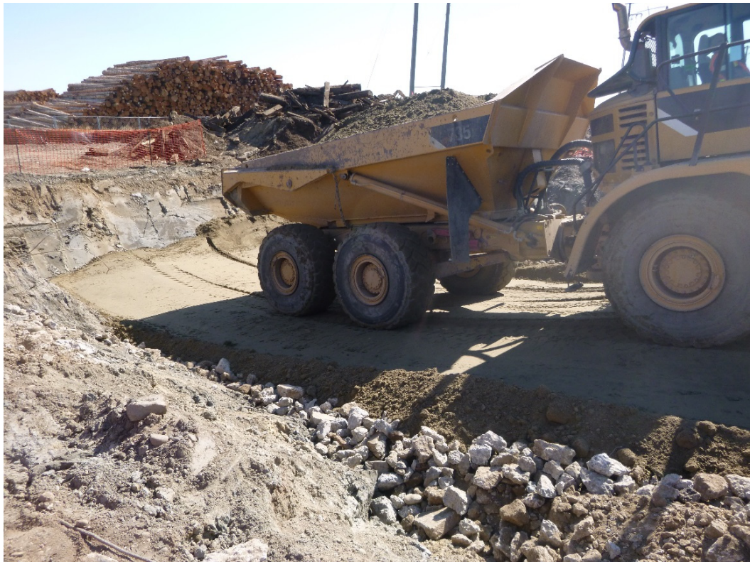
Photograph 6. Excavation Area 2, week of August 17, 2015.
