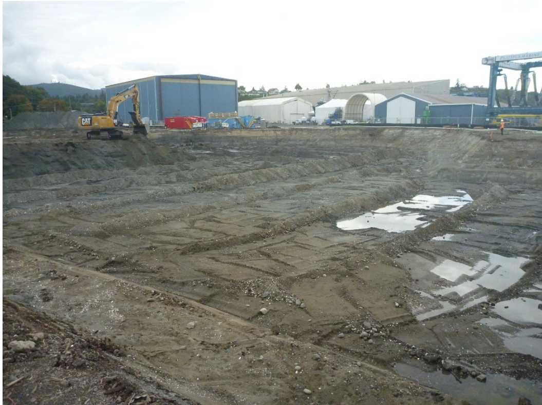
Photograph 15. Excavation Area 5, week of September 28, 2015.
