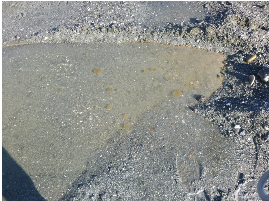
Photograph 14. LNAPL within Excavation Area 6.
