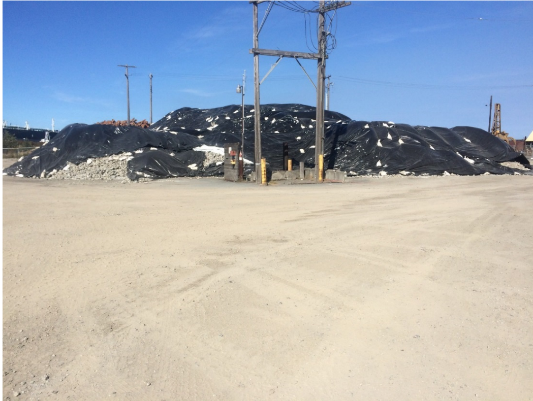
Photograph 1. Covered crushed concrete stockpile.
