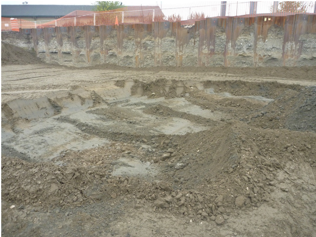
Photograph 16. Backfilling soft spot in Excavation Area 6 near sheetpile.
