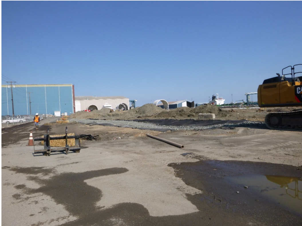
Photograph 3. Excavation Area 5, week of August 10, 2015.
