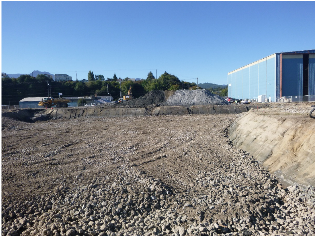
Photograph 9. Excavation Area 5, week of September 7, 2015.
