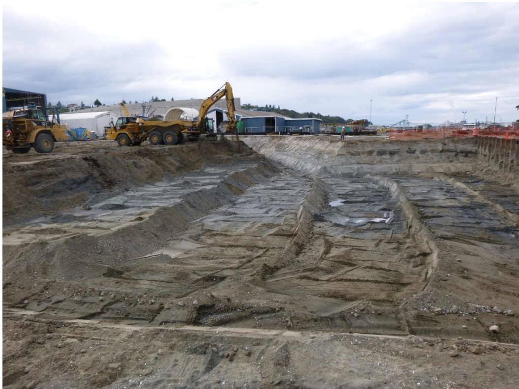
Photograph 14. Excavation Area 6, week of September 21, 2015.
