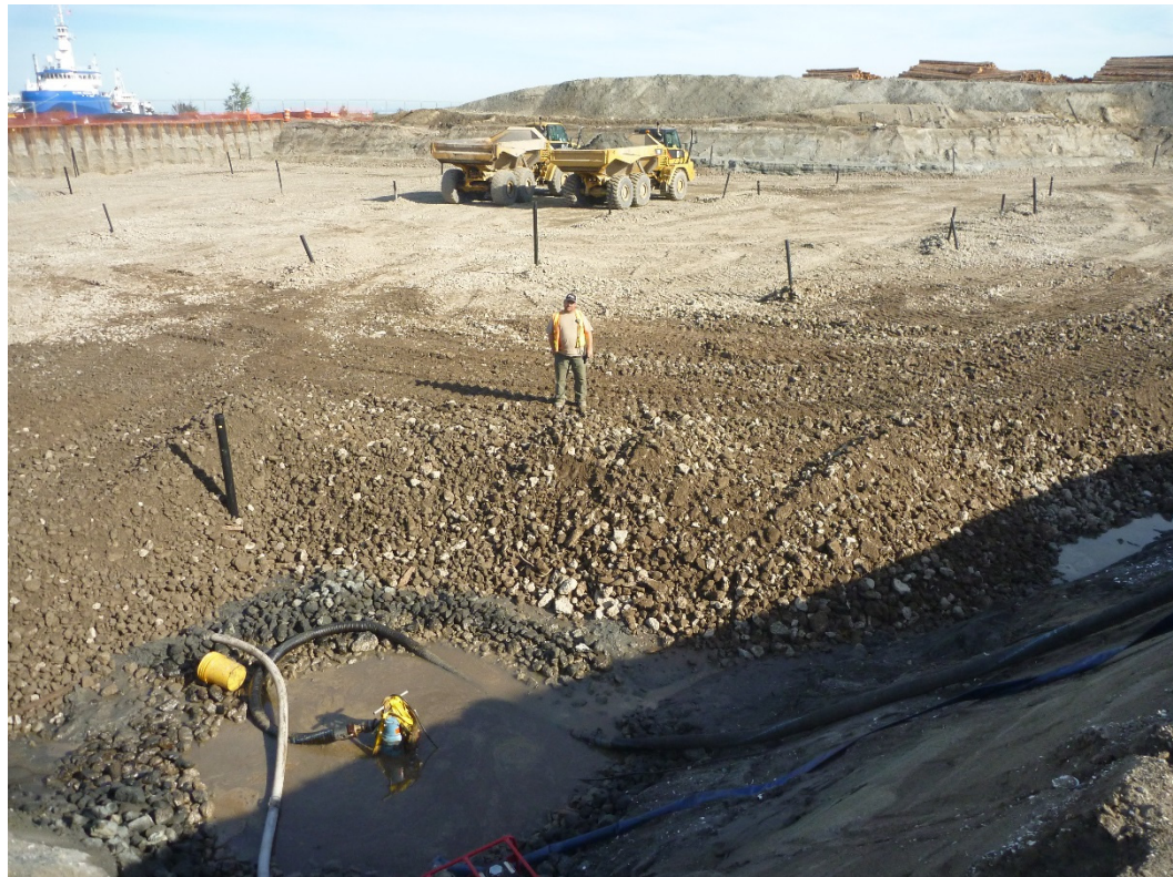
Photograph 20. Excavation Area 6, week of October 12, 2015.
