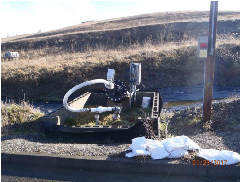
Photo 5: Leachate side slope riser #2
