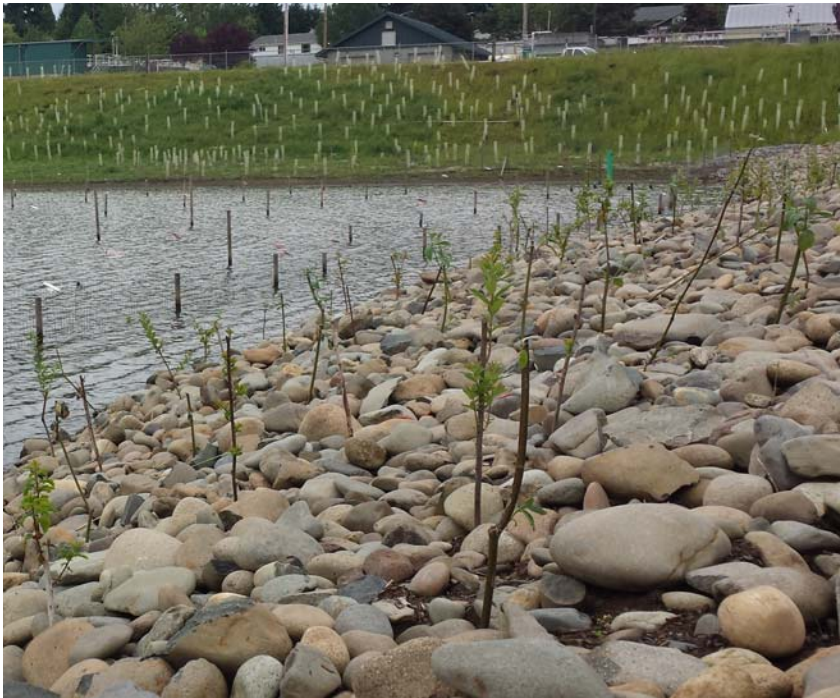
Looking northeast at live stakes at foot of south embankment. 5/11/15
