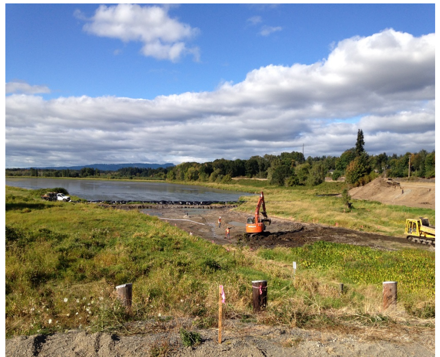
Looking north at sediment excavation operations.
