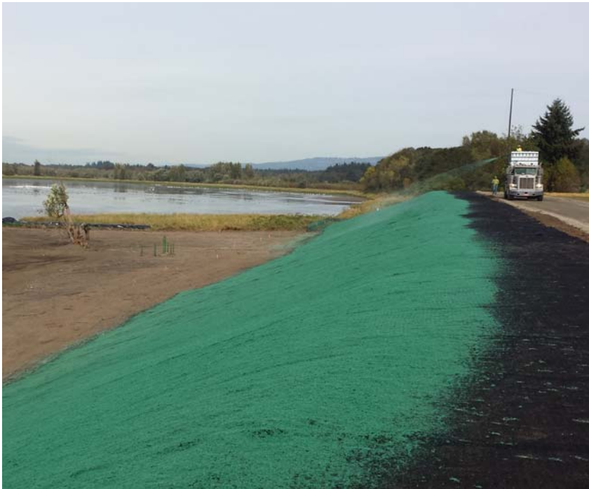
Looking north at hydroseeding of east embankment 10/13/14
