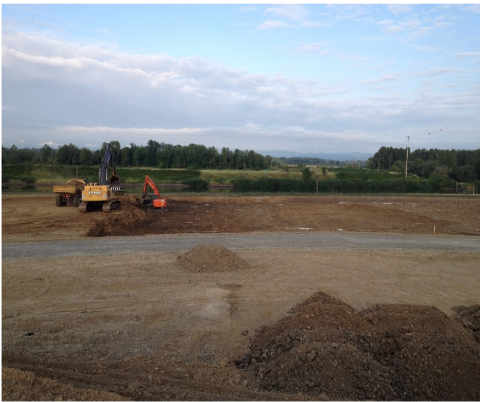
Clean soil cap removal.
