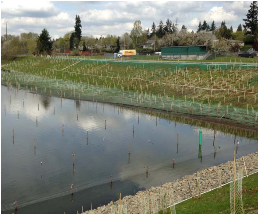
Looking northeast at planted east embankment, above ground irrigation and temporary in-water fencing. 3/28/15
