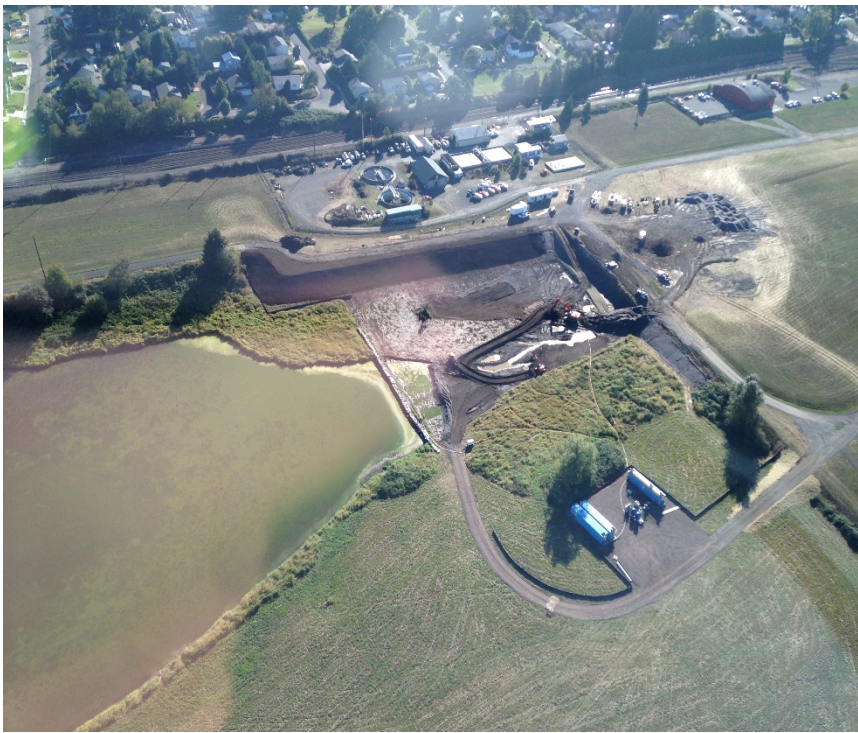
Looking southeast at progress to date from a helicopter.
