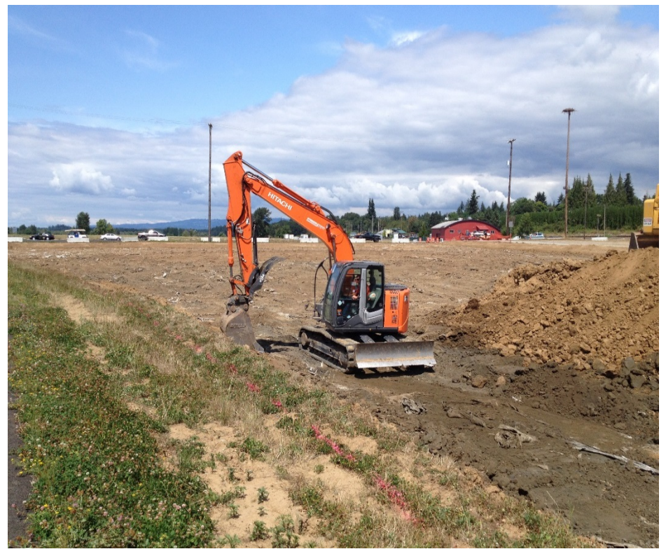
Clean soil cap removal.
