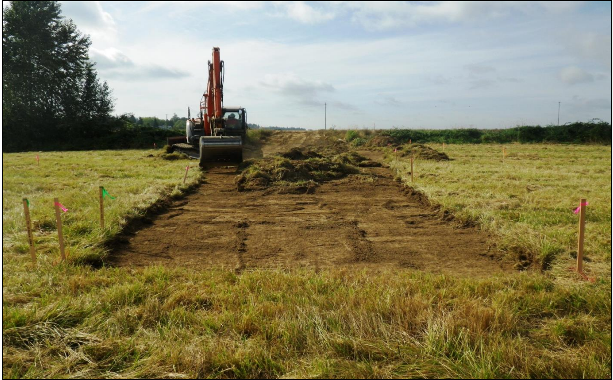
Figure 6. Overview of grubbing for ramp construction, facing south.
