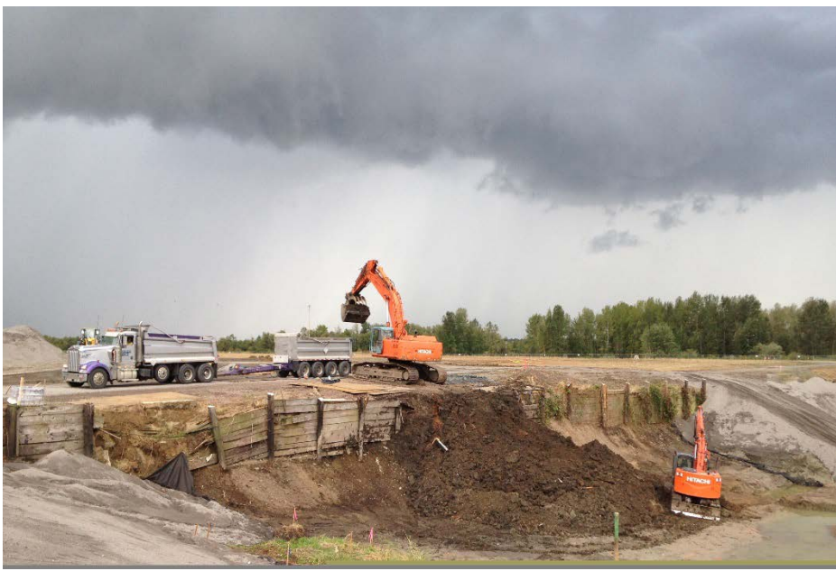
Looking southwest at the progress on the stockpile.
