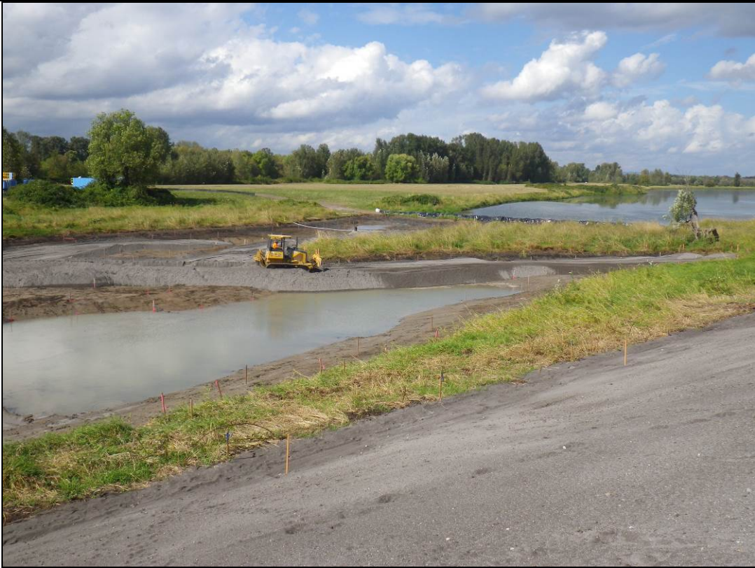
Photo 2. Overview of area where 12-35-5IF was identified, facing northwest.
