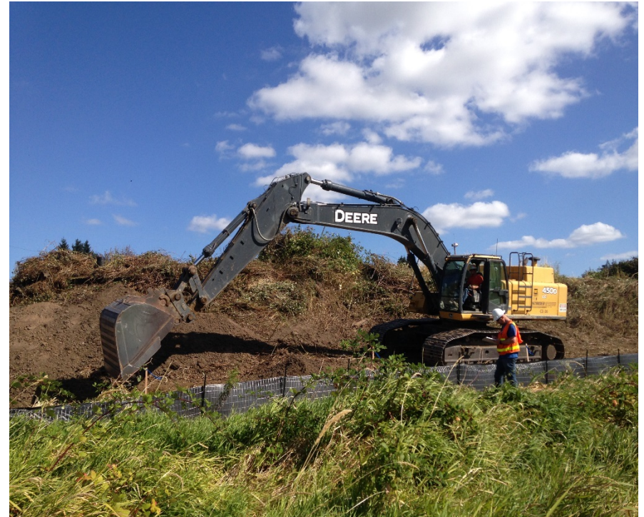
Looking east at the 450 excavating the keyway on the east embankment.
