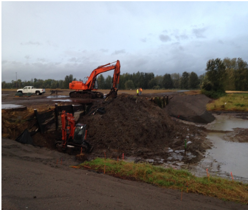
Looking southeast at the sediment stockpile.
