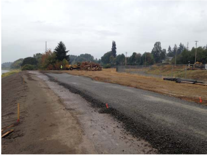
Photo 1: Looking southeast at the crushed surfacing placed on the hard trail.
