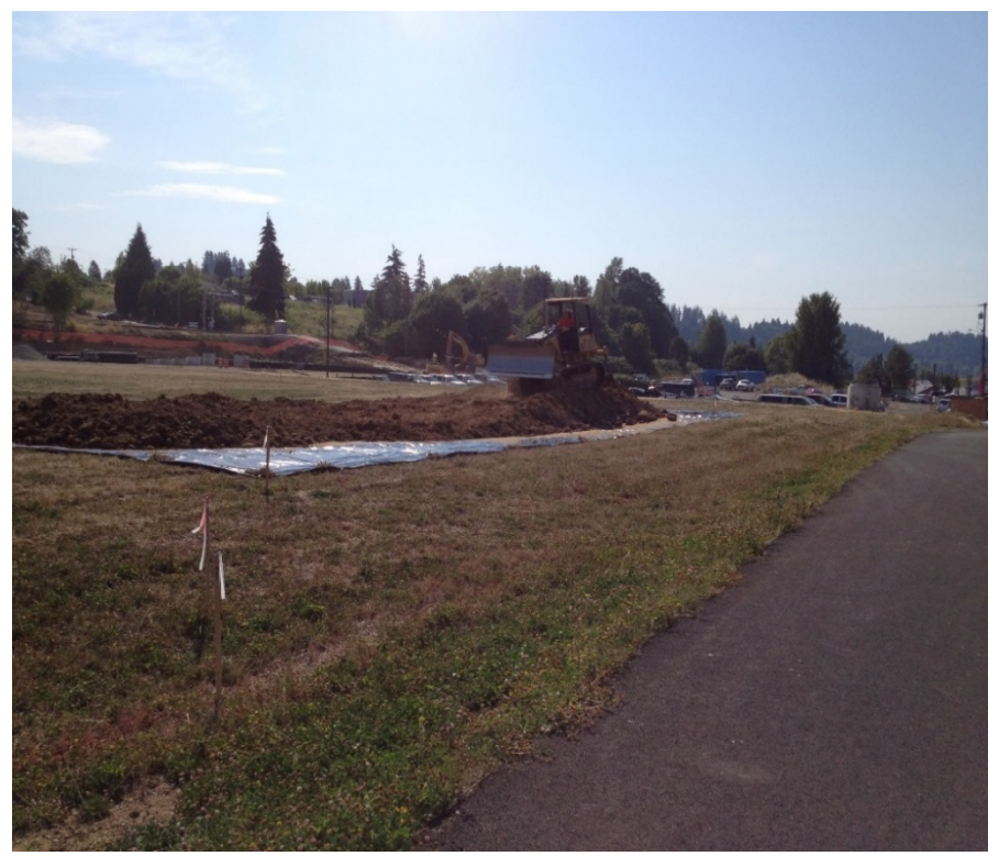
Clean soil cap stockpiled on liner
