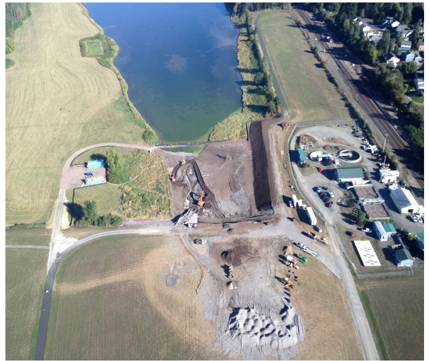
Looking north at progress to date from a helicopter.
