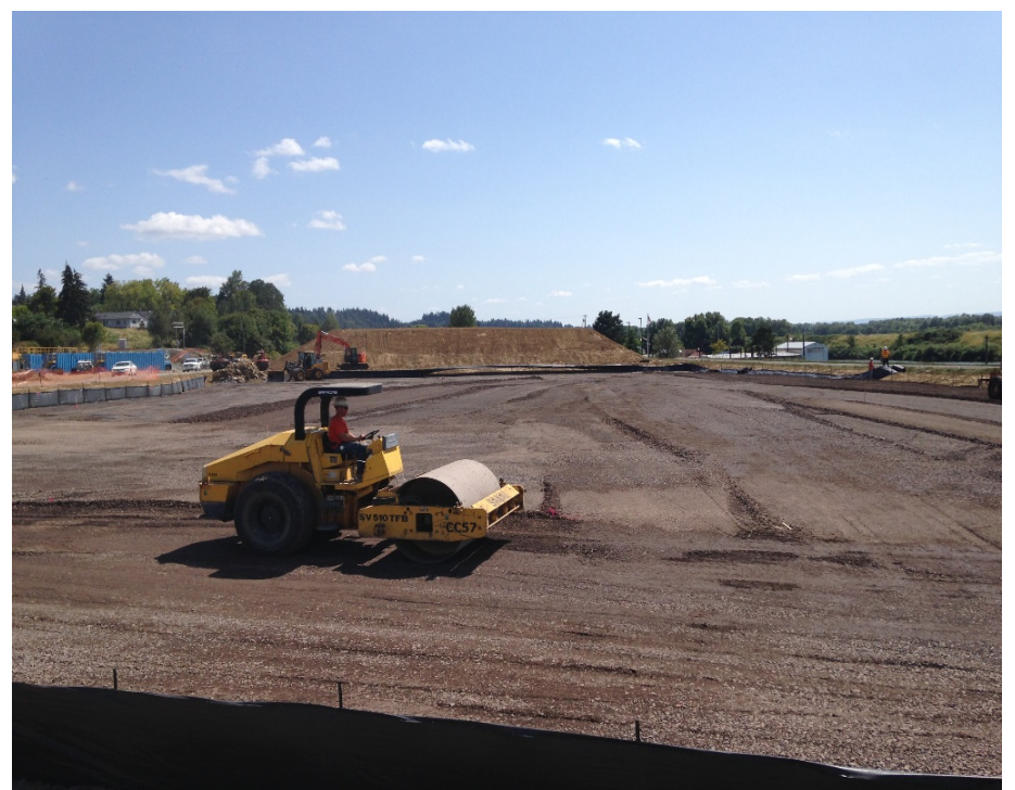
Looking south at roller compacting recently placed ballast.
