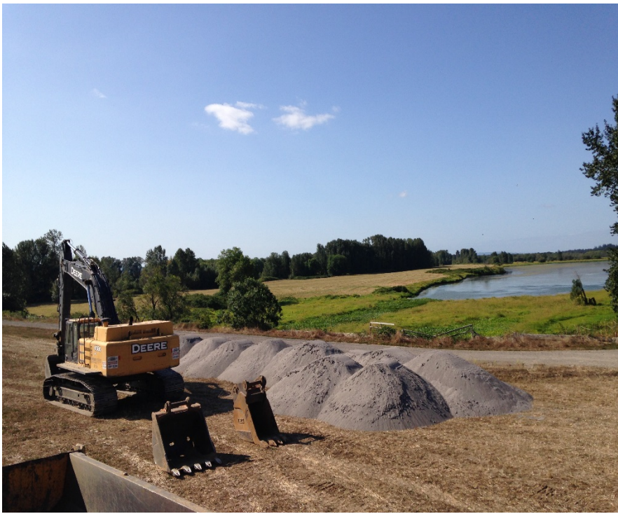
Looking southwest at stockpiled clean sand and Carty lake.
