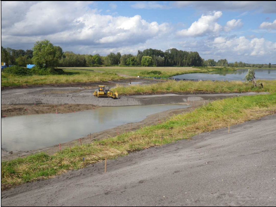
Photo 2. Overview of area where 12-35-4 was identified, facing northwest.
