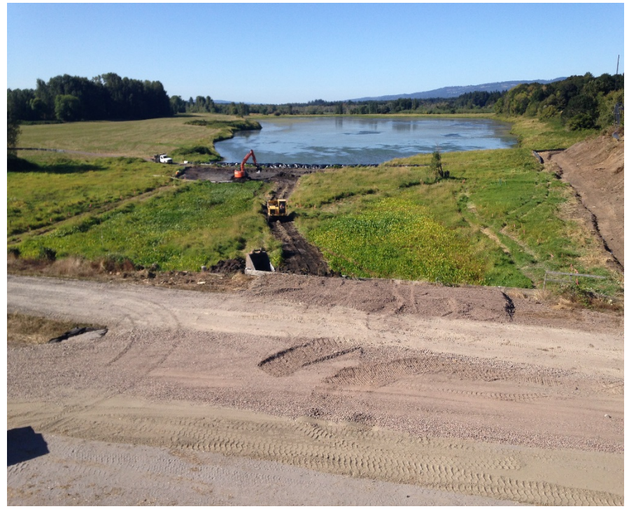
Looking north at sediment excavation activities.
