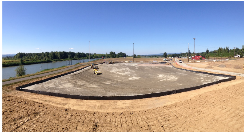
Looking north at the nearly completed upland sediment handling area.
