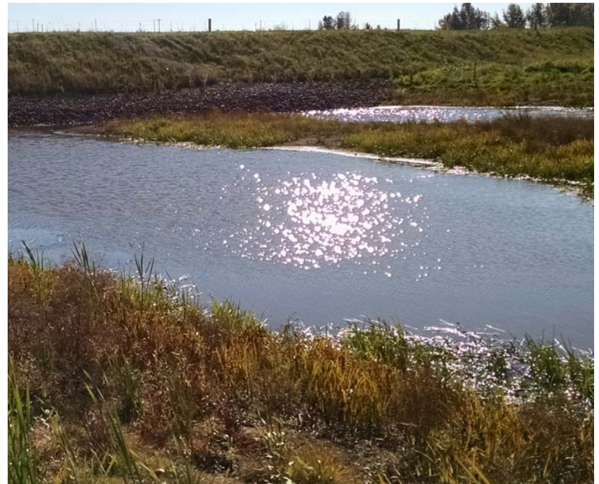
Looking southwest at established transitional vegetation adjacent to deep in-water areas. 10/1/15
