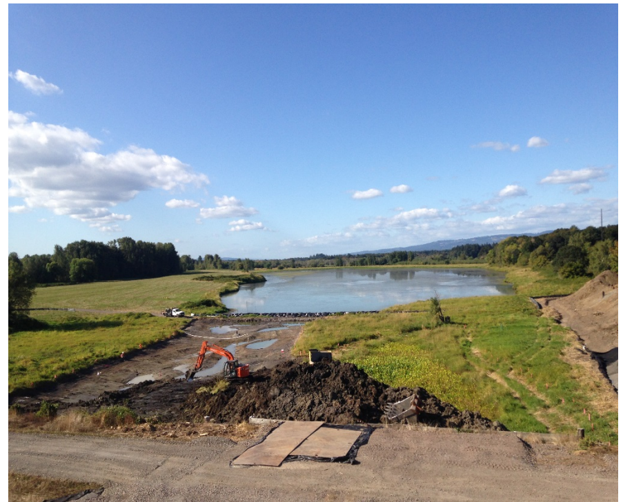
Looking north at sediment excavation operations from the sand stockpile.
