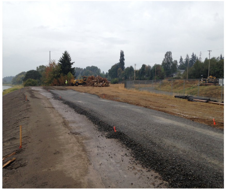
Looking southeast at the crushed surfacing placed on the hard trail.
