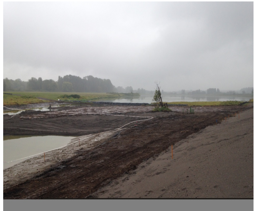
Looking north at the extents of clearing and grubbing completed.
