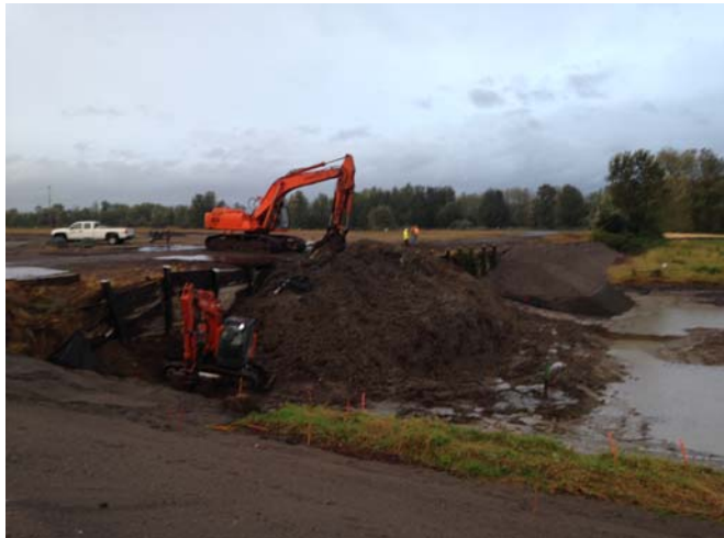
Photo 2: Looking southeast at the sediment stockpile.
