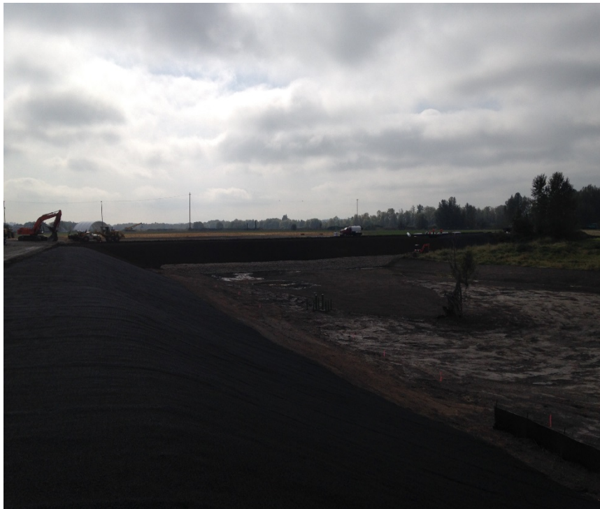
Looking south at the completed project.
