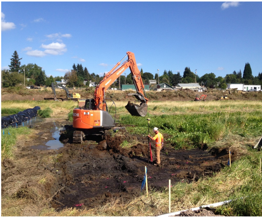
Looking east at the beginning of sediment excavation activities.
