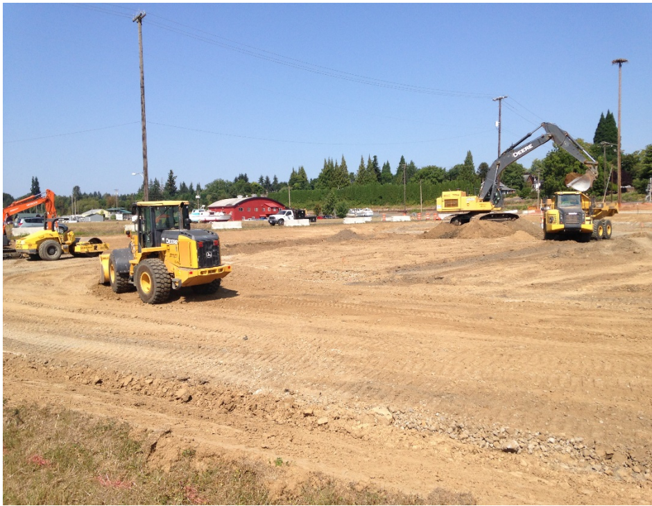
Looking northeast at grading of the sediment handling area.
