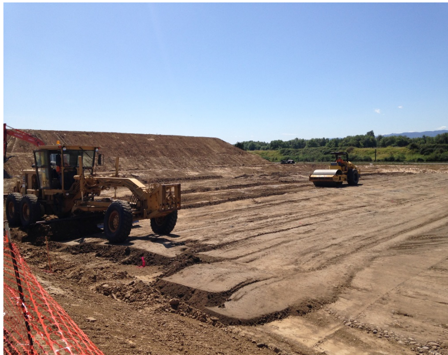
Looking southwest at grader and roller grading out the subgrade.
