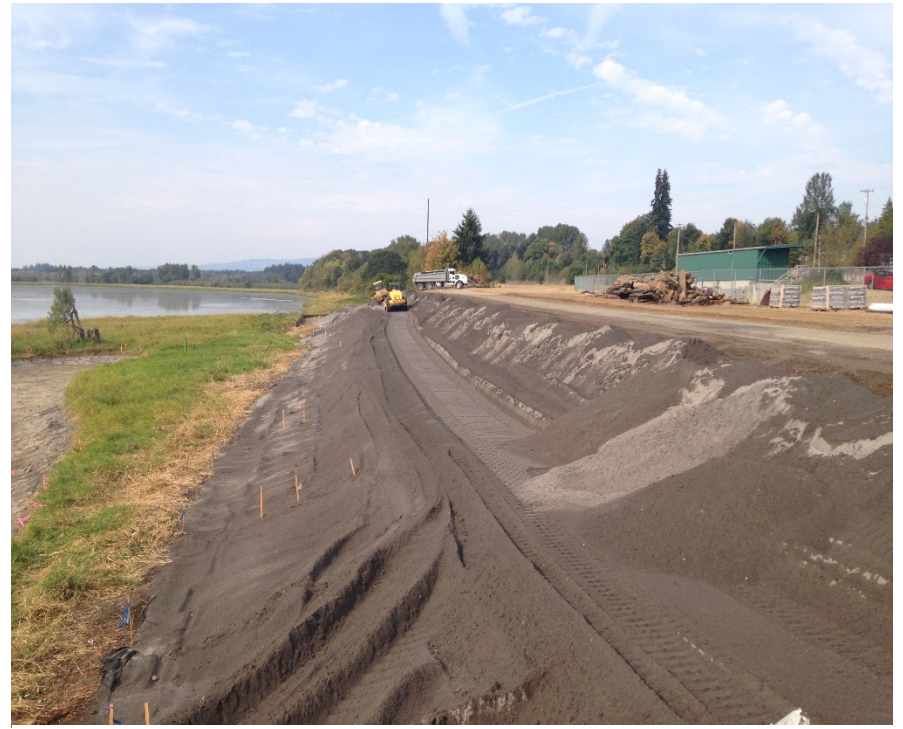
Looking north at compactive efforts on the east embankment.
