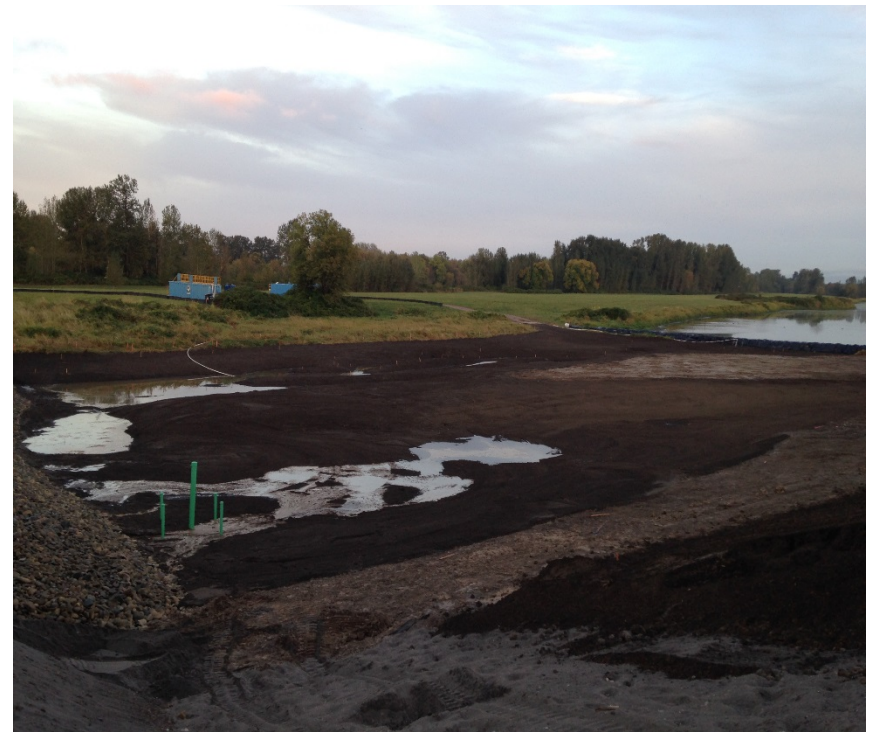
Looking northwest at the substantially completed clean sand placement.
