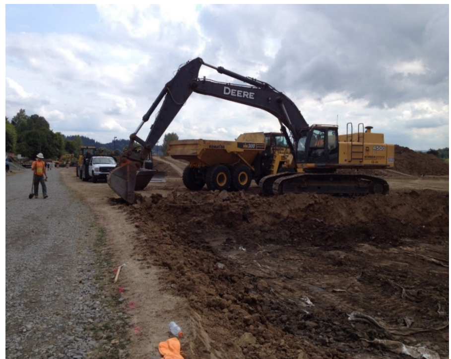
Clean soil cap removal.
