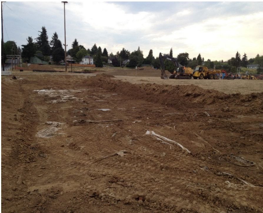
Clean soil cap removal.
