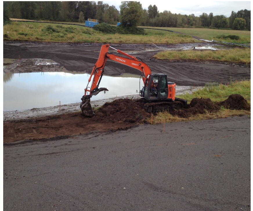
Looking west at scraping of reed canary grass.
