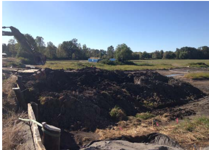
Photo 2: Looking west at the stockpile of contaminated sediment awaiting transport and disposal.
