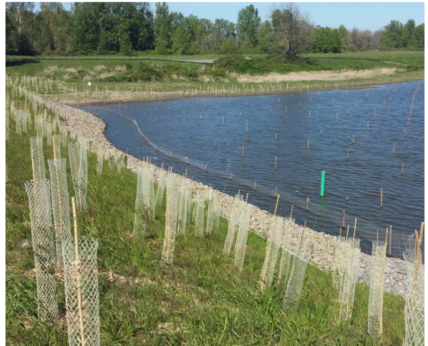
Looking west at planted south and west embankment. 4/17/15
