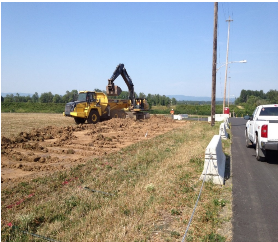
Clean soil cap removal.
