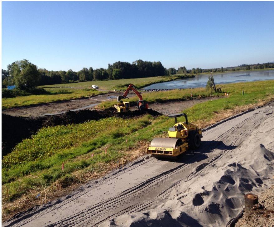
Looking northeast at sediment excavation activities and east embankment construction.
