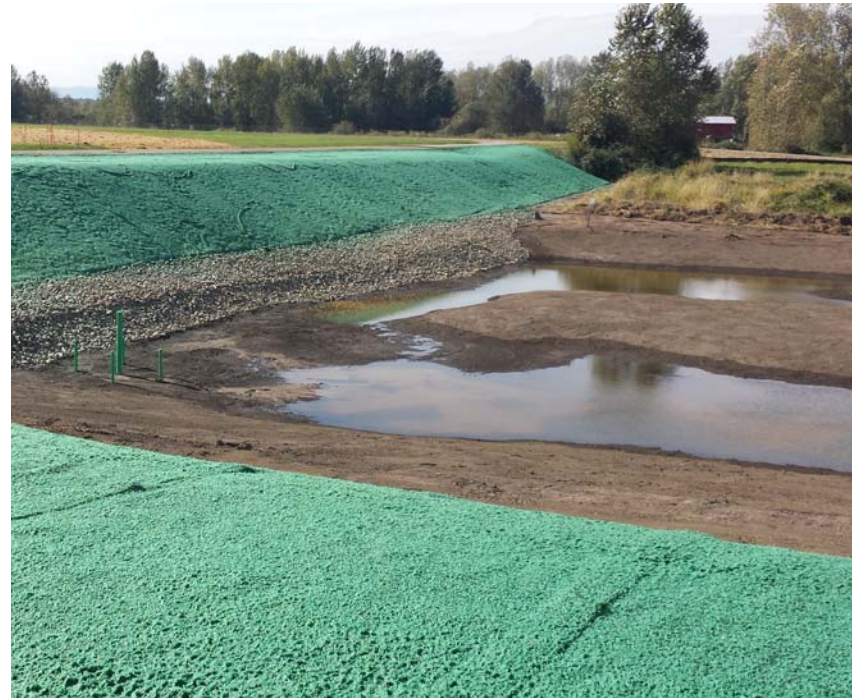
Looking southwest at hydroseeded south embankment. 10/13/14
