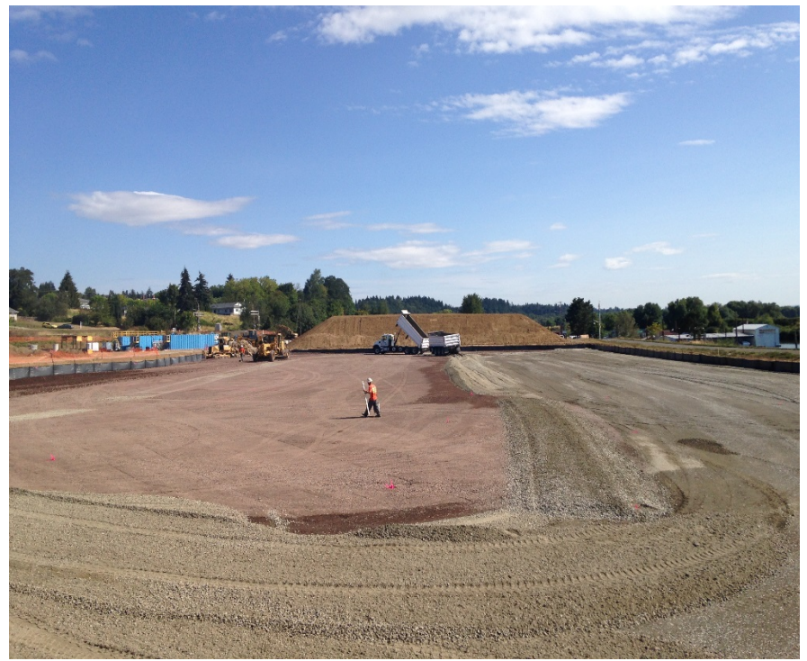
Looking south at grader grading ballast and truck delivering crushed surfacing
