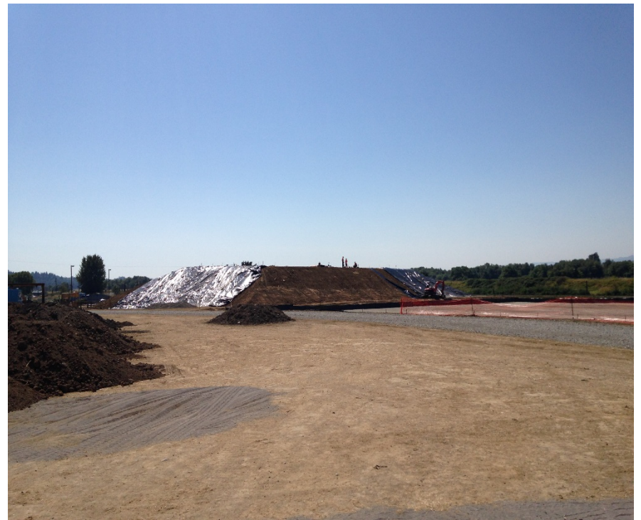
Looking southwest at the covering of the clean soil cap stockpile.
