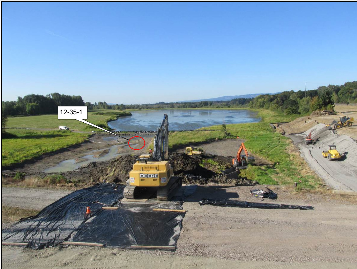
Photo 3. Overview of site location, facing north. Carty Lake in background.
