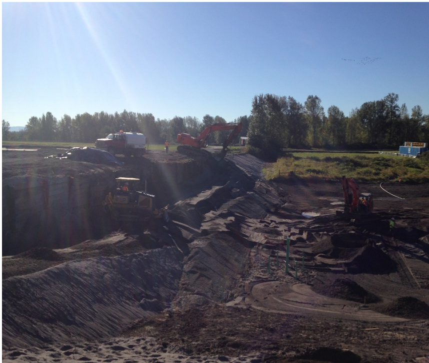
Looking west at the south embankment being constructed.
