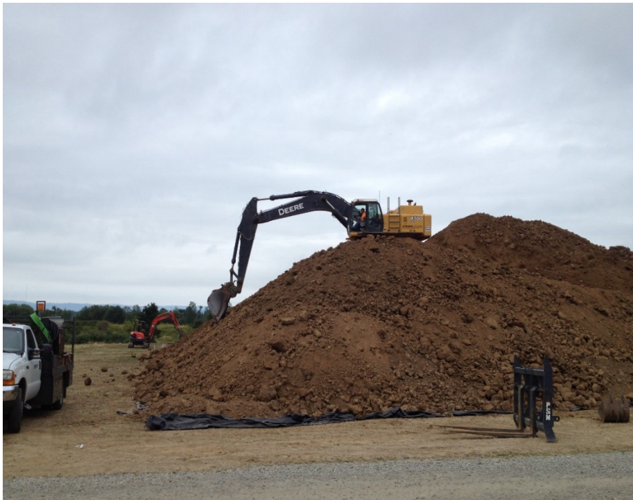
Dressing clean soil stockpile.
