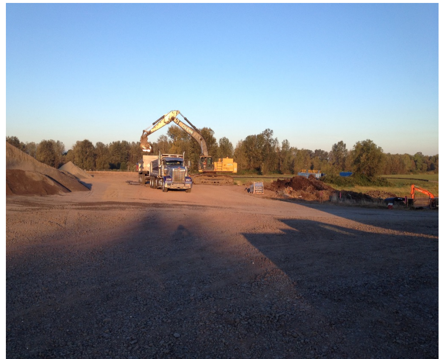
Looking west at a truck getting loaded with sediment for disposal.
