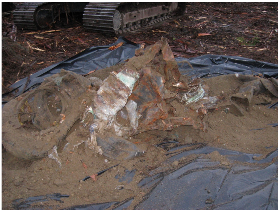
Photograph 8 Metal siding at TP-G-5.
