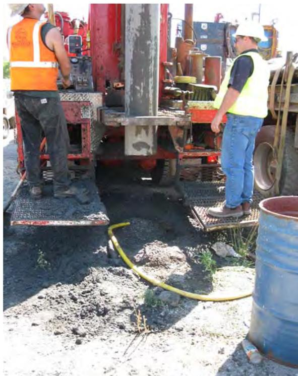
**Photograph 2** – Hydrating the bentonite surface seal at AW-1.
