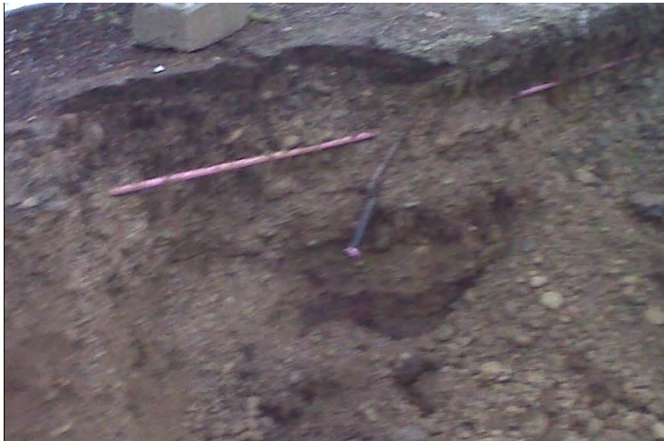
CNF-3 Excavation, looking east
