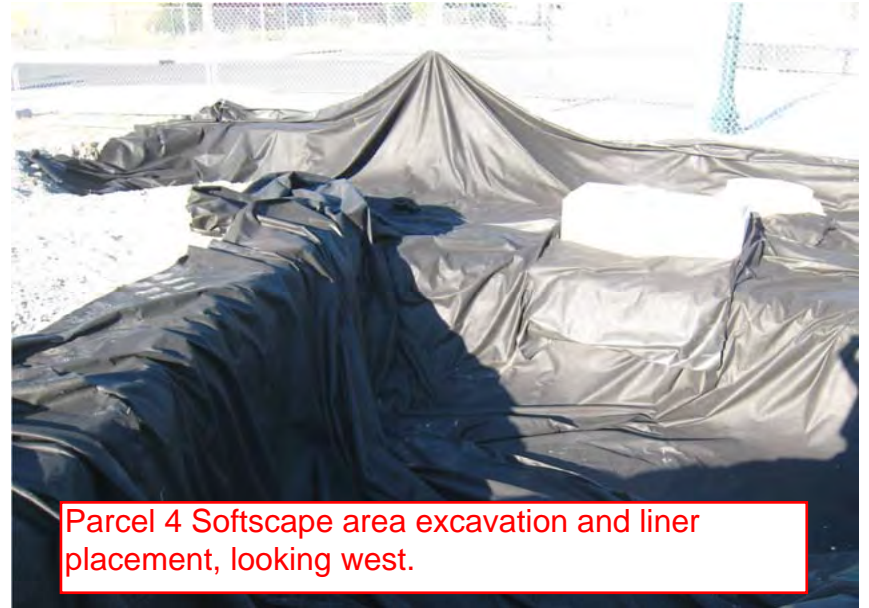
Parcel 4 Softscape area excavation and liner placement, looking west.
