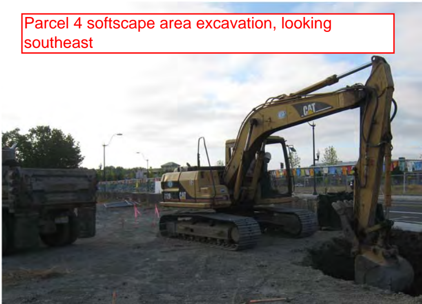
Parcel 4 softscape area excavation, looking southeast
