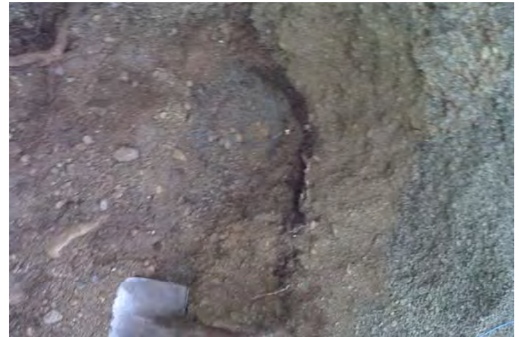
CNF-4 Excavation, looking down at west edge
