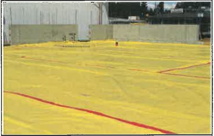
Photo 8. Overlapping seams taped.
