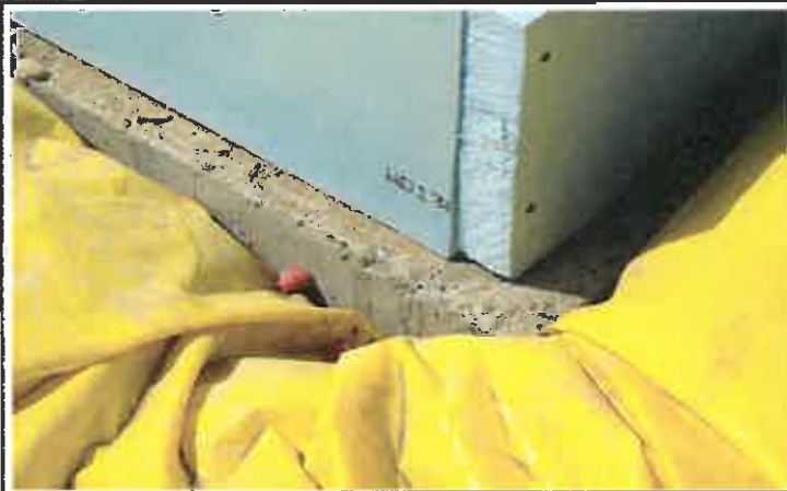
Photo 3. Stego vapor barrier extending beneath perimeter concrete footing of northern building.
