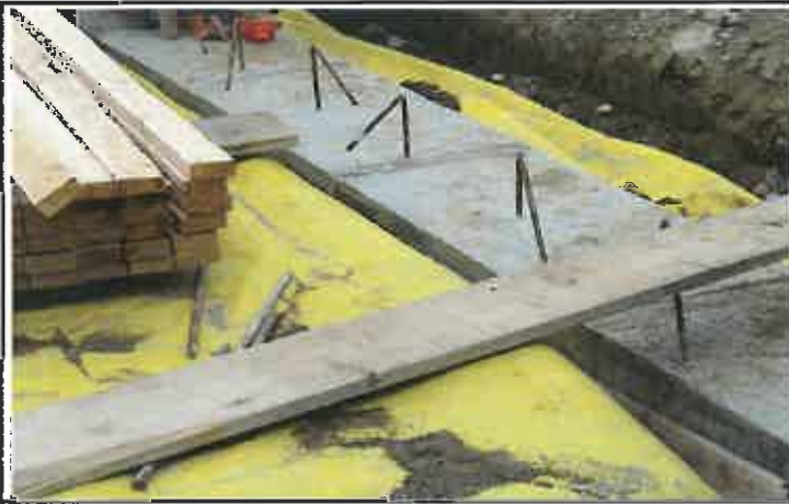
Photo 1. Stego barrier extending under perimeter footing.
