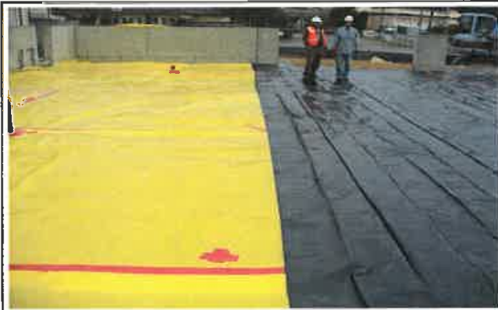
Photo 9. Placing layer of 10-mil visqueen over stego vapor barrier.
