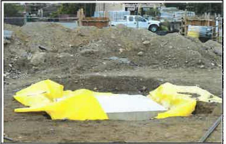
Photo 2. Stego vapor barrier installed under utility vault south of northern building.
