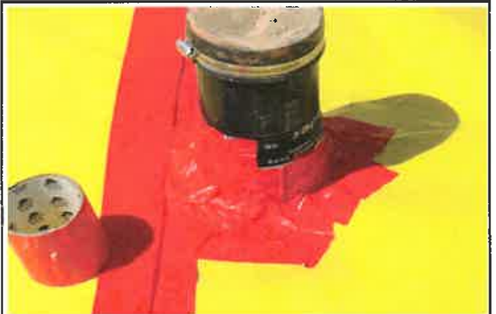
Photo 6. Pipe penetrations taped.
