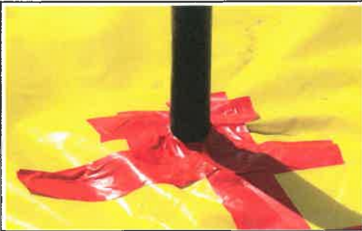
Photo 7. Pipe penetration taped.
