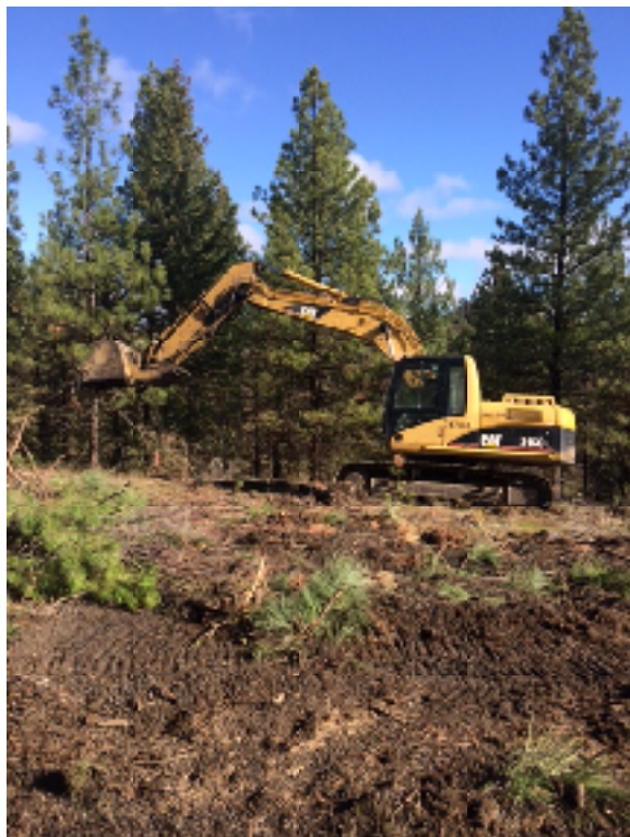
Photo 4 Excavating contaminated soil at former skeet shooting range.
