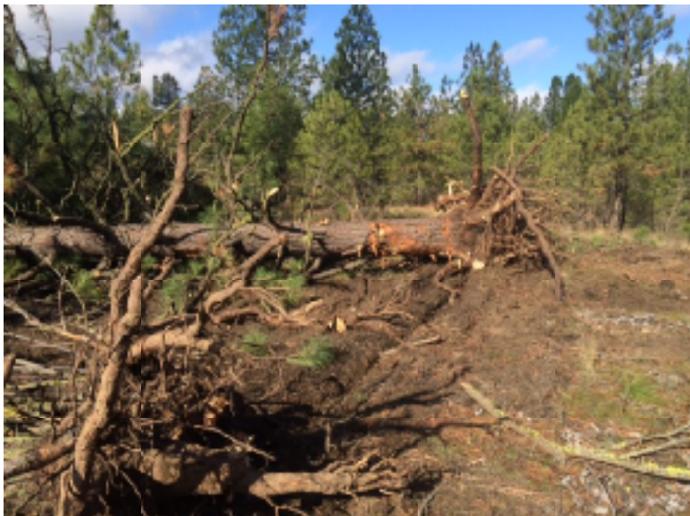
Photo 3 Beginning stages of soil re mediation - removal of existing pine trees.
