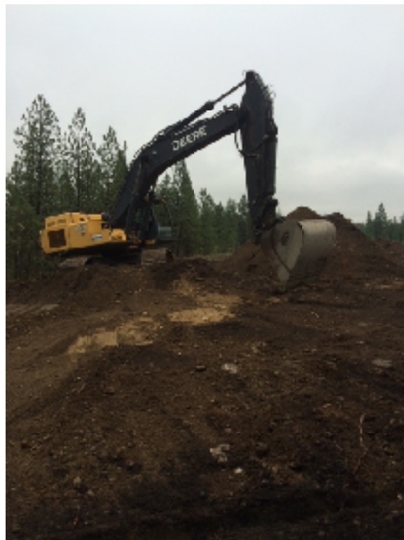
Photo 5 Clearing surficial clay pigeon debris from property.
