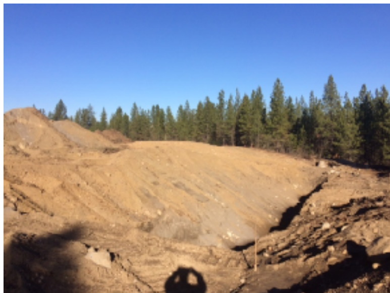
Photo 6 View of sewer pipeline trench excavation at the site.
