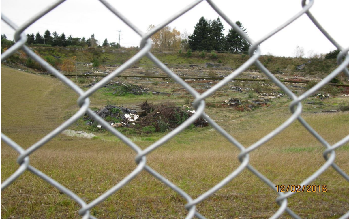
Photo 7: Aeration Stabilization Basin– From the West
