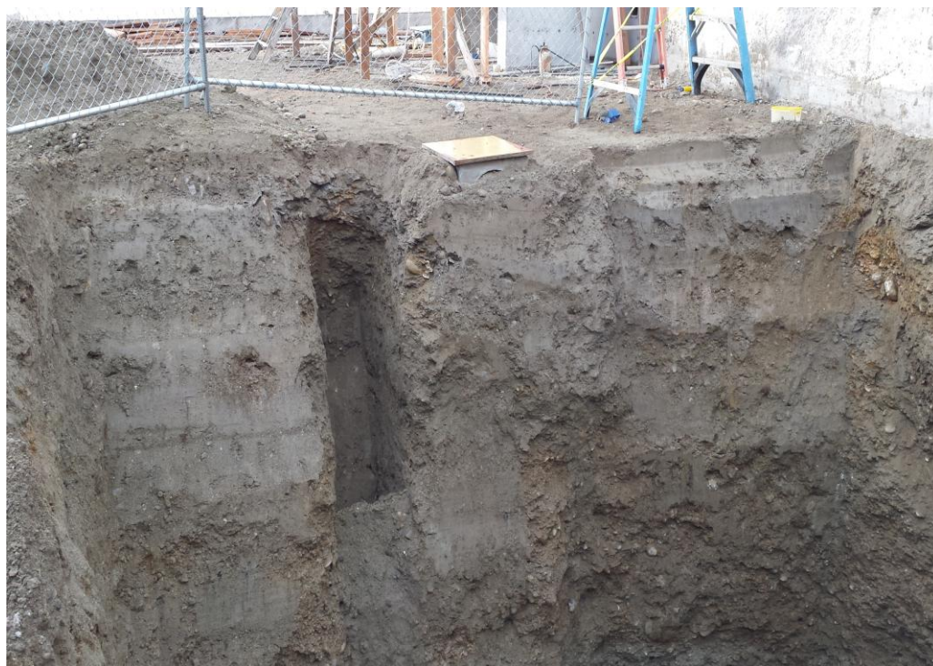
4. Delineation of plume began with a slot to the south. Contamination limits were recognized southward of the slot in this photo.
