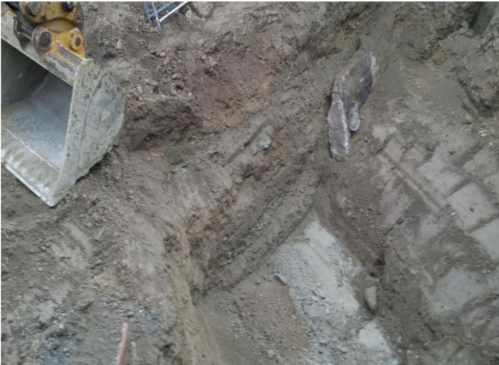
5. Higher concentrations of contamination were exposed as investigation and excavation continued. This was in the central area of the site.
