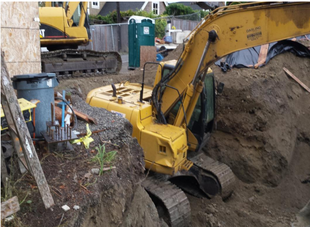
6. As contaminant continued deeper, a ramp was cut from the north.
