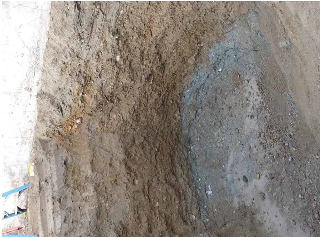
3. Contamination in the northeast corner was exposed, sampled, and tested. Concentration of diesel home heating oil was above MTCA Method A cleanup standards.
