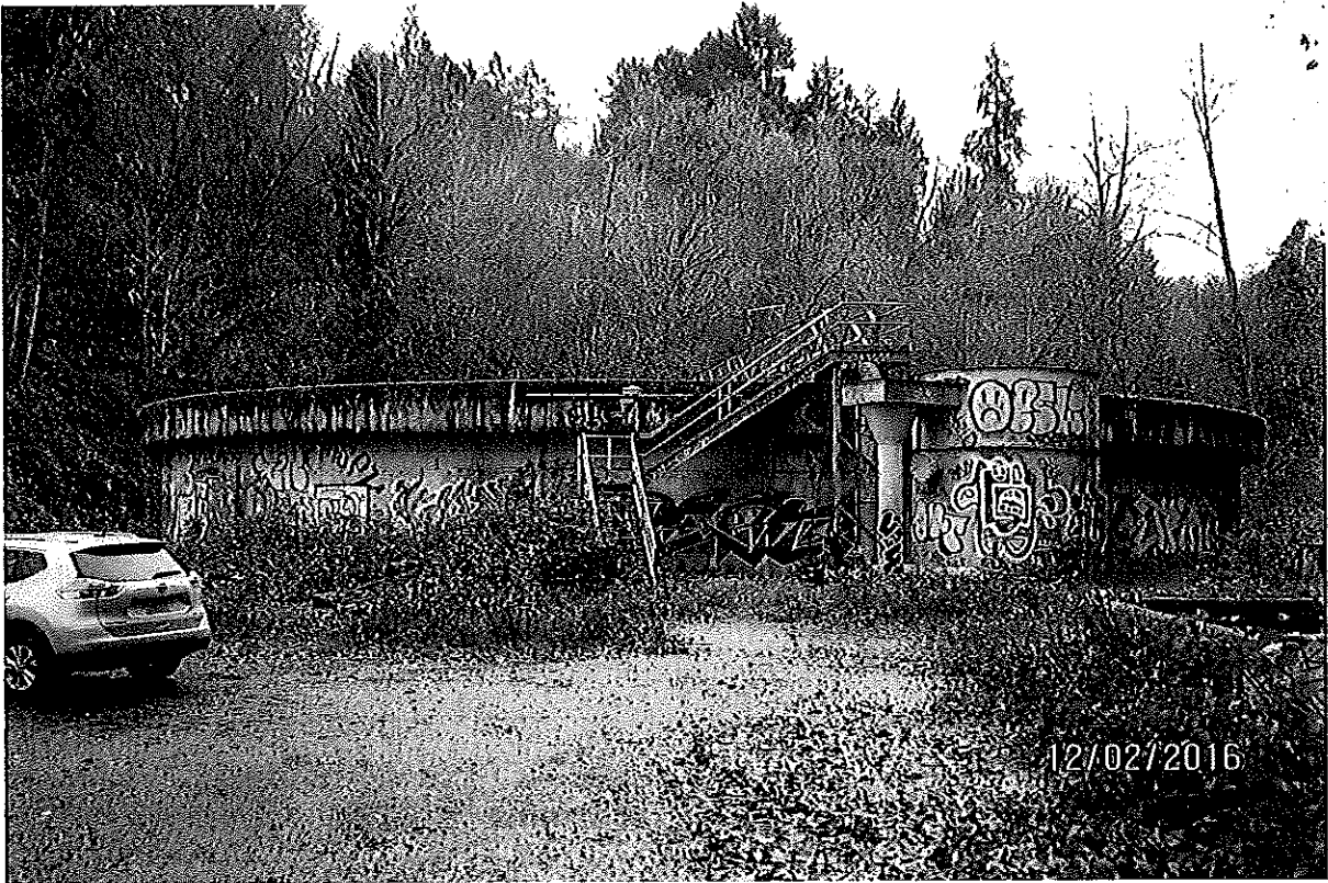
Photo 8: Wastewater/Processed Water Treatment Clarifier – From the East
