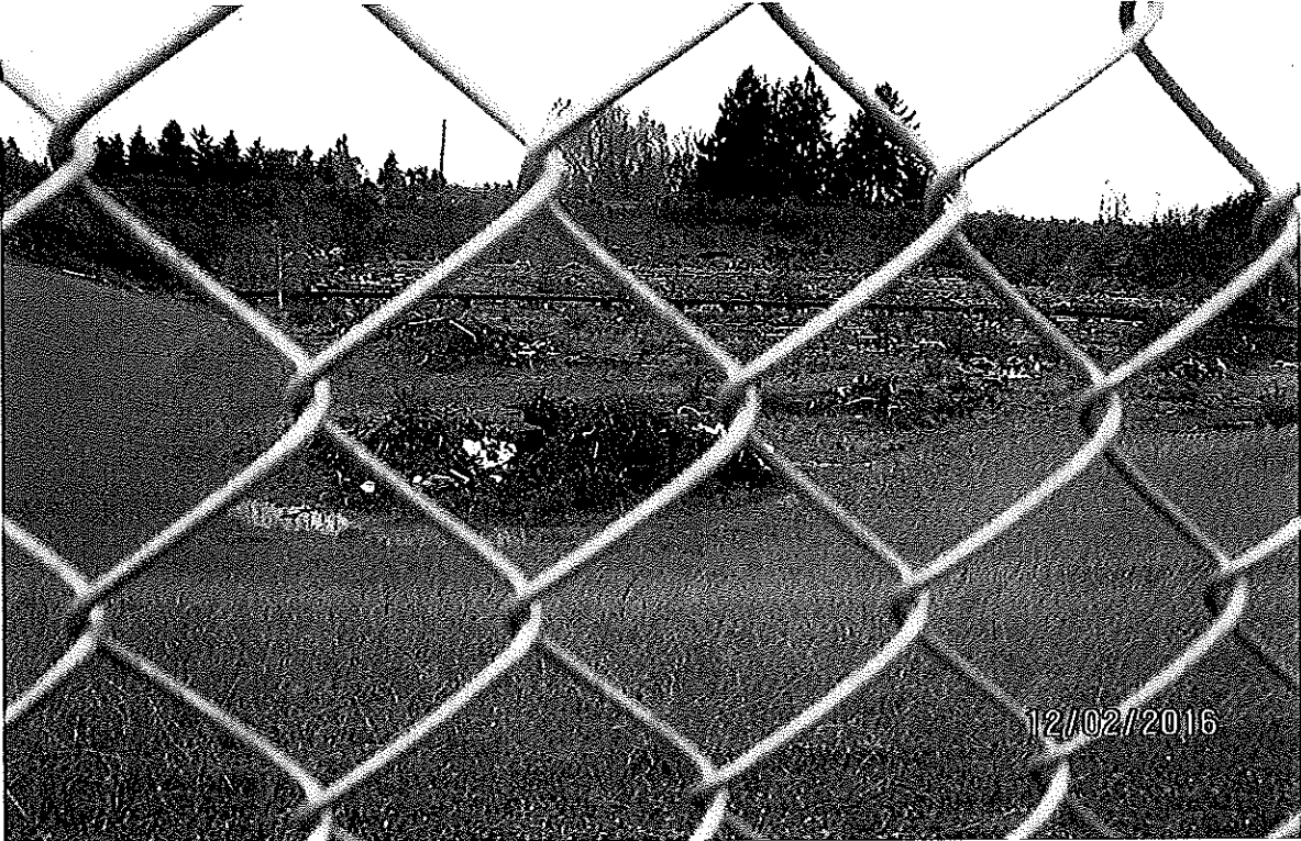
Photo 7: Aeration Stabilization Basin– From the West
