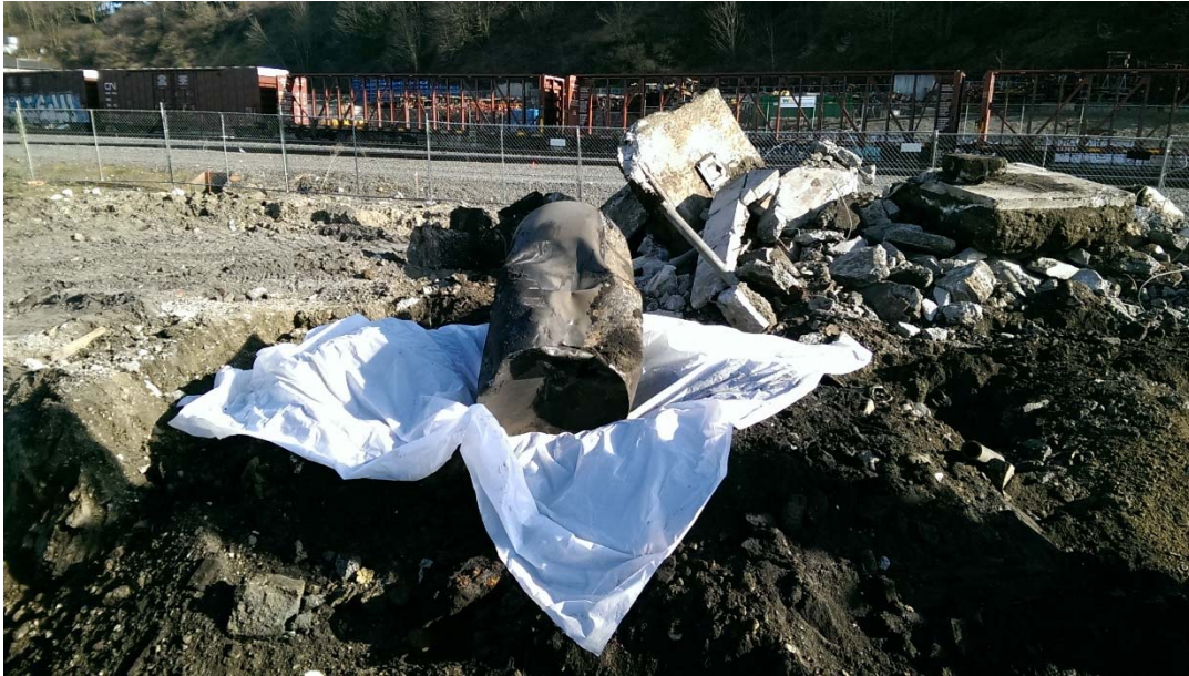
Photograph 3 UST after moving to temporary staging area. View is to the east.
