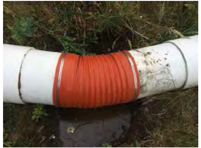
Flex-hose repair east of well E-25
