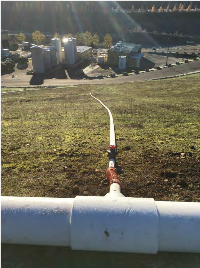
Removed 10 inch wye and rerouted lateral at well E-2
