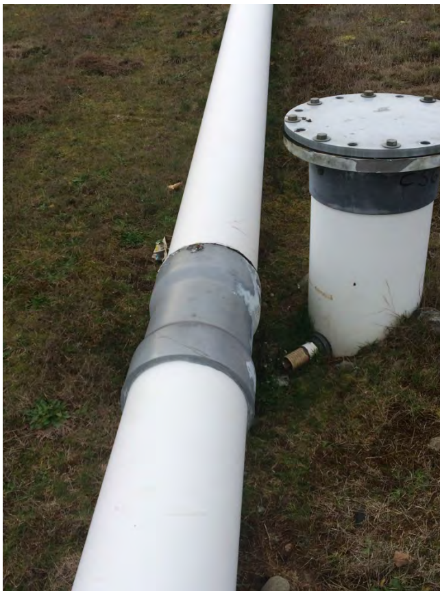
Repair of condensate sump CS-6
