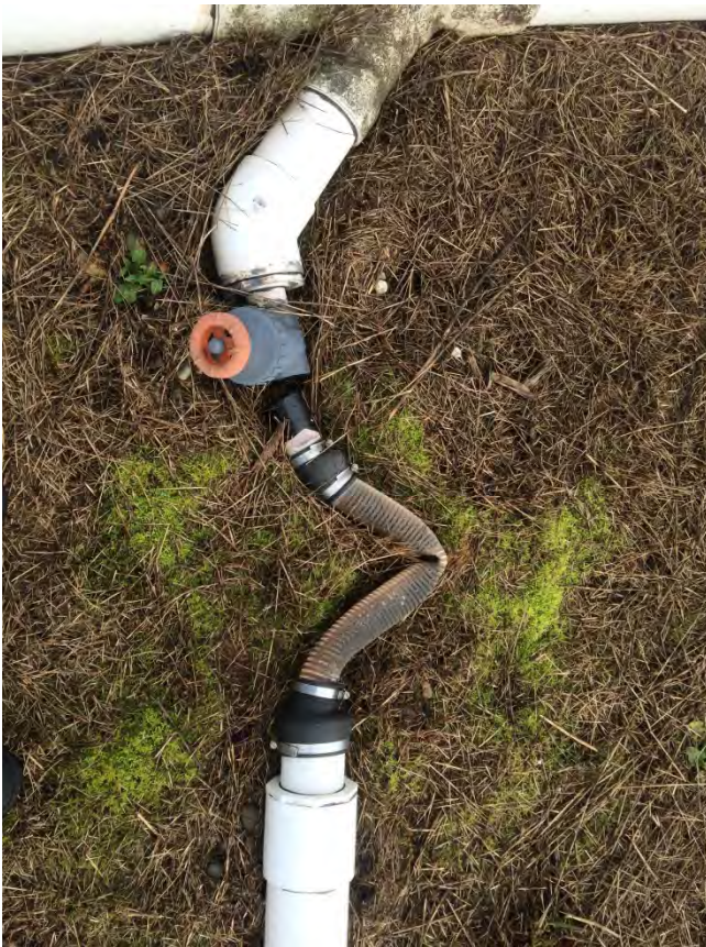
Repair of extraction well N-14
