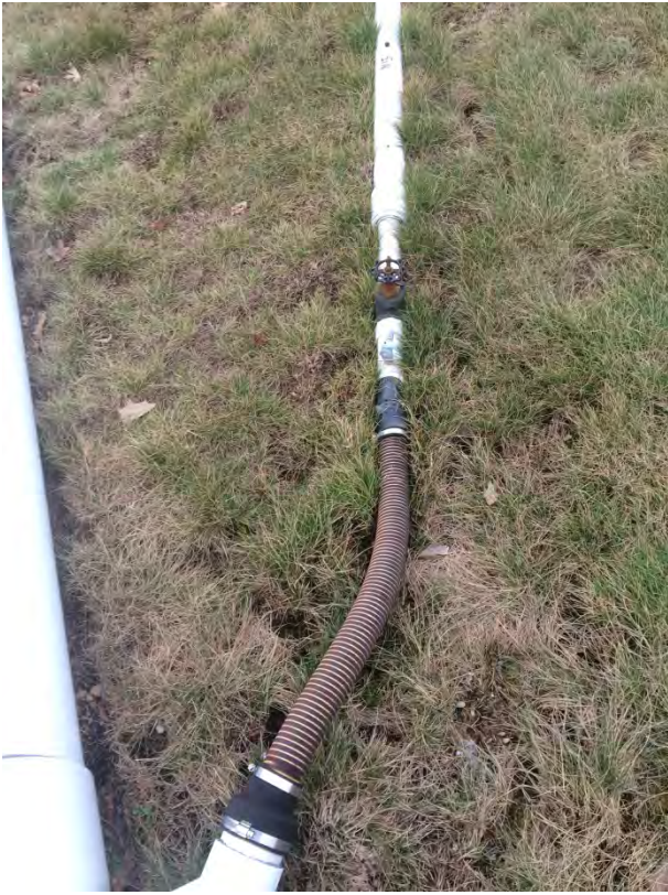
Repair of Extraction Well N-15
