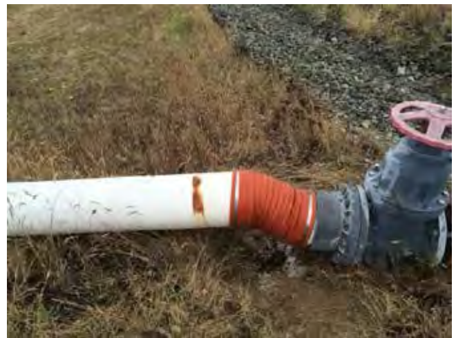
Flex-hose repair south of well E-12
