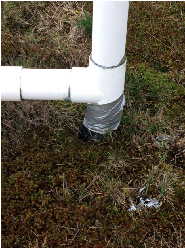
Repair of Extraction Well N-6
