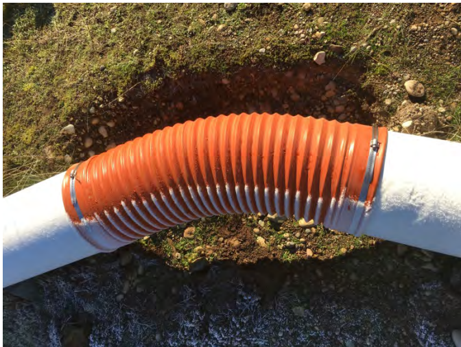
Replaced flex-hose at well E-2
