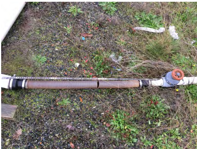
Flex-hose repair at well N-58
