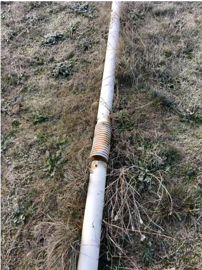
Repaired lateral at well N-44
