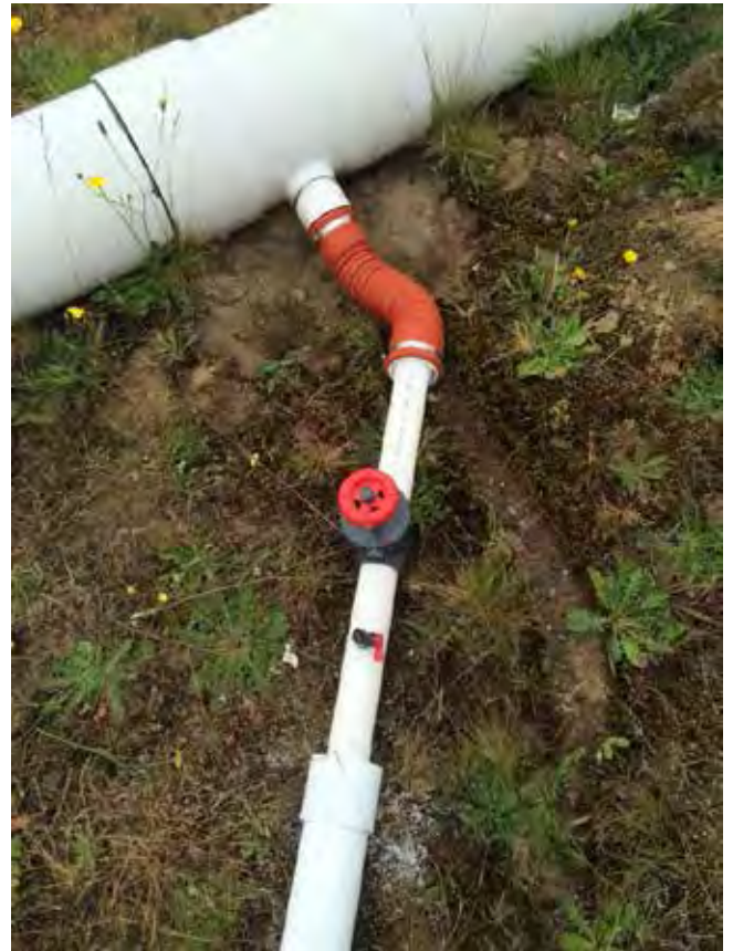
Flex-hose repair at N-17
