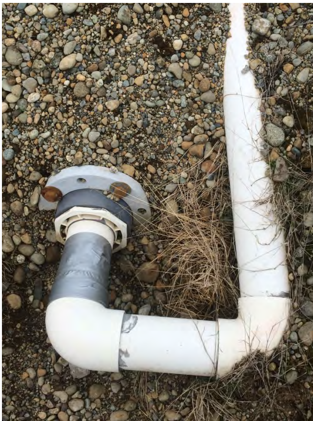
Repair of piping at condensate sump CS-2
