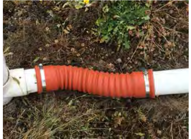
Flex-hose repair at N-29
