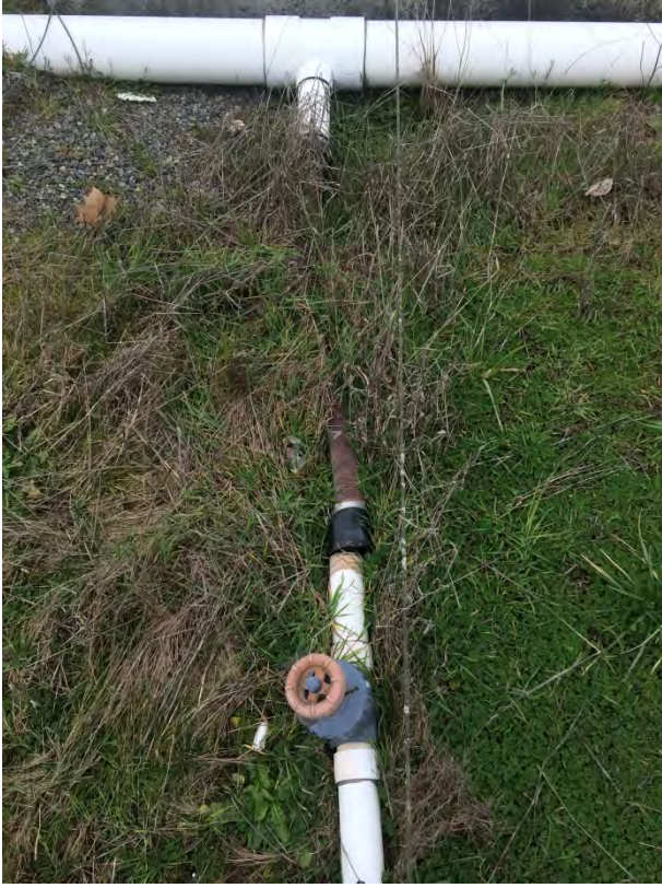
Repair of Extraction Well N-60
