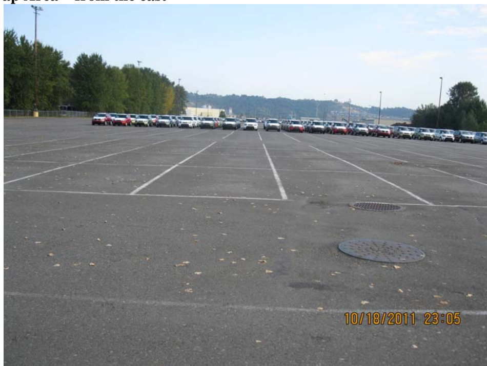
Photo 2: Cap Area – from the east
