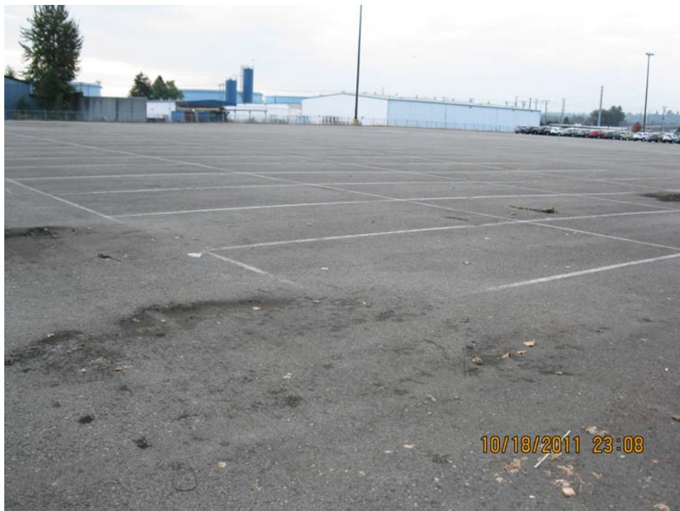
Photo 4: Minor Cap Damage
