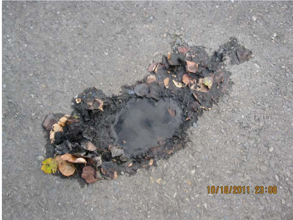
Photo 4: Minor Cap Damage
