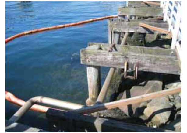
P7 PHOTO - DRAIN PIPE
