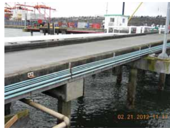
P6 PHOTO - UTILITIES & SUPPORTS Ⓧ NORTH EDGE OF DOCK WALKWAY
