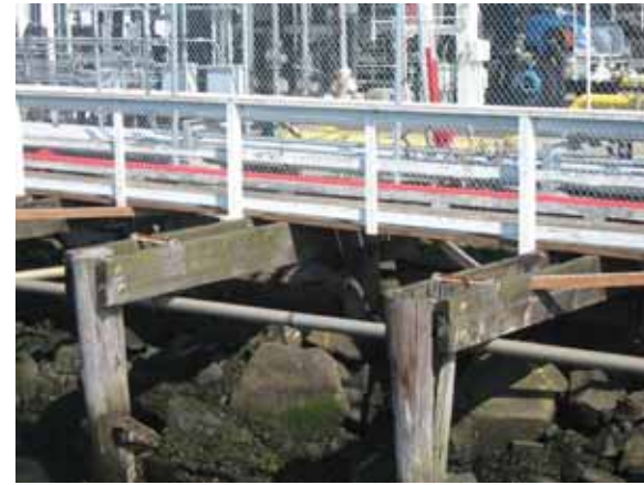
P5 PHOTO - (E) BULKHEAD & WALKWAY
