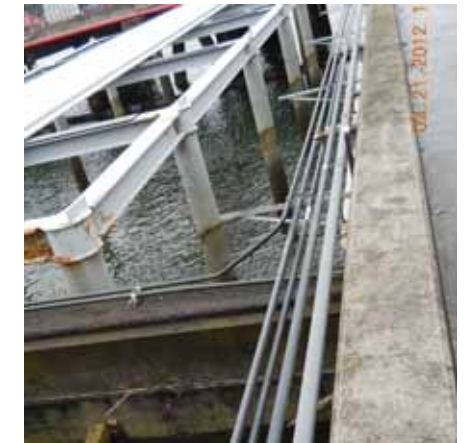
P8 PHOTO - UTILITIES & SUPPORTS Ⓧ SOUTH EDGE OF DOCK WALKWAY
