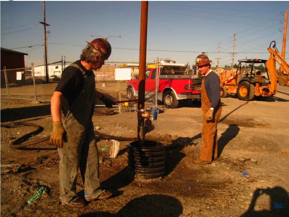
Figure B.2 – Current wellhead condition of AW-1
