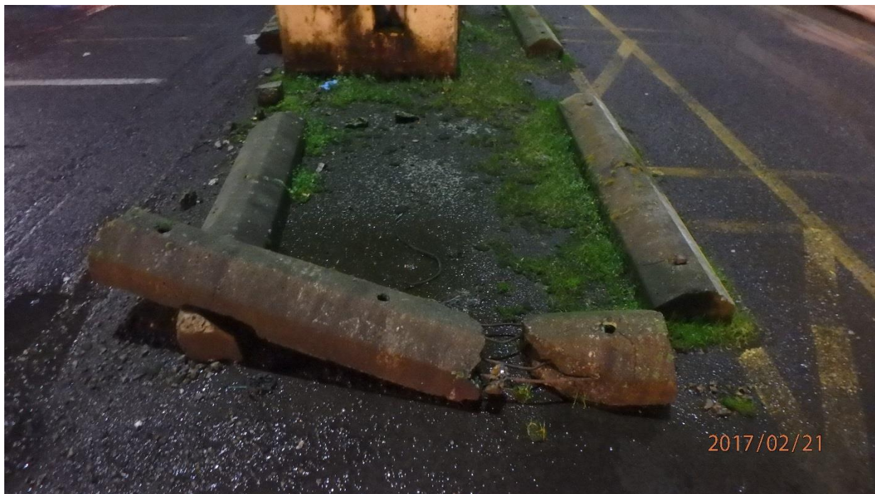
Figure 5. Example of deteriorated wheel stops
