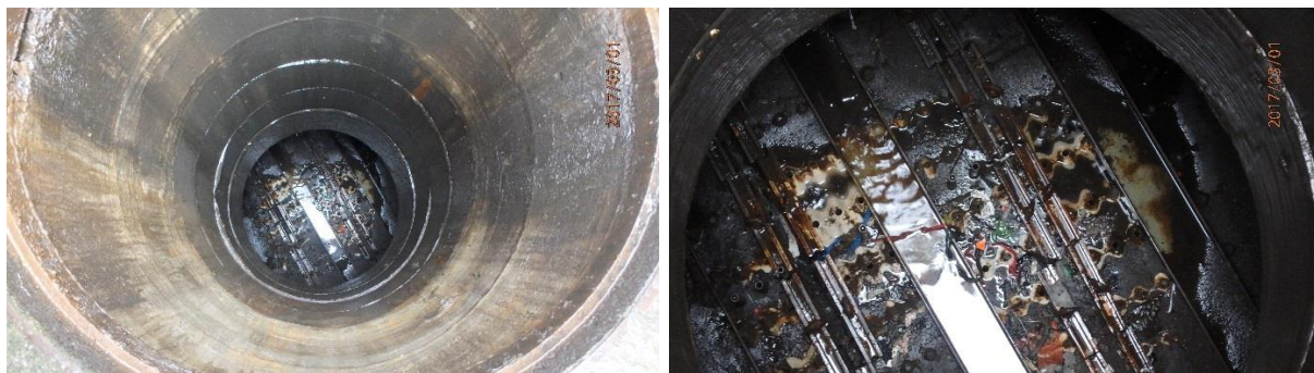
Figure 6. Representative views of sediment accumulation on the coalescing plate oil/water separators
