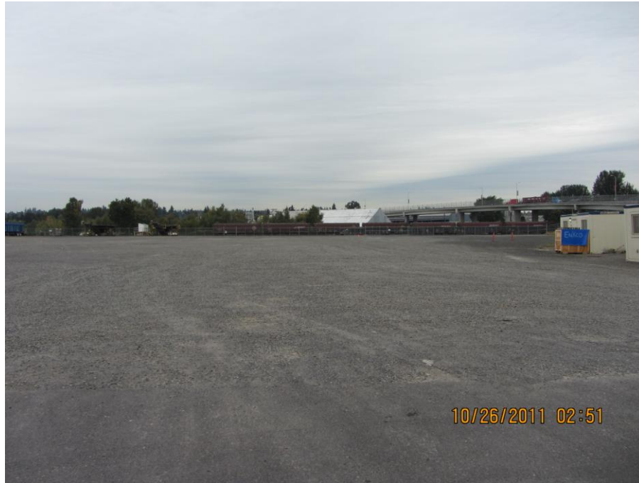
Photo 2: Former Pond Site Engineered Gravel Cap – Looking West
