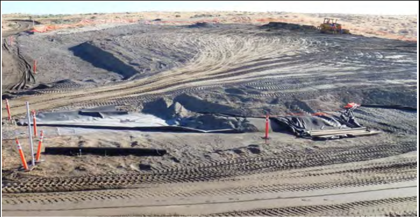
Photo 3: View of the western side of the CAP. Note the western and NW swales have not yet been graded out with the EOC. View looking north from SW corner of the site.
