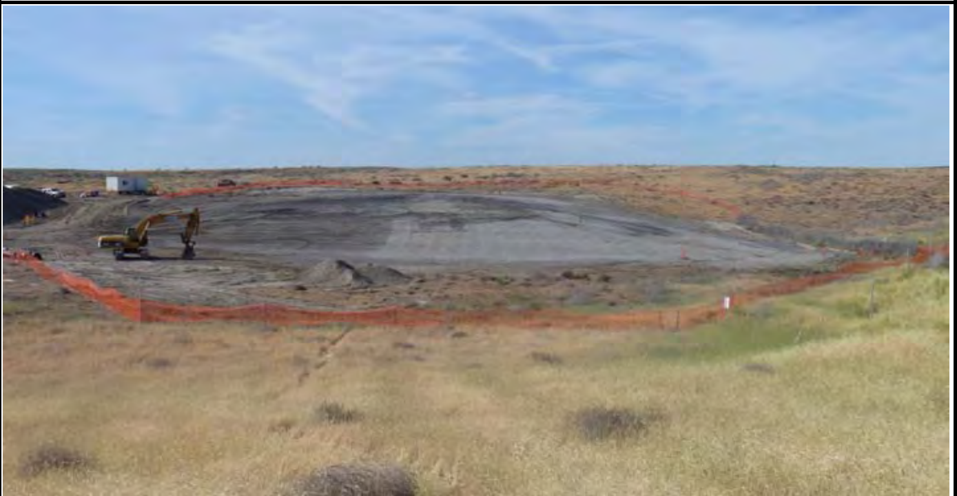
Photo 10: View of the site at the conclusion of work for the day. OCF has been installed along the south end of the new perimeter fencing posts. Note infiltration basin grading stockpile that will be installed in the G-layer along the eastern edge of the cap (along AE-4 western edge). View looking north from area beyond south end of site.
