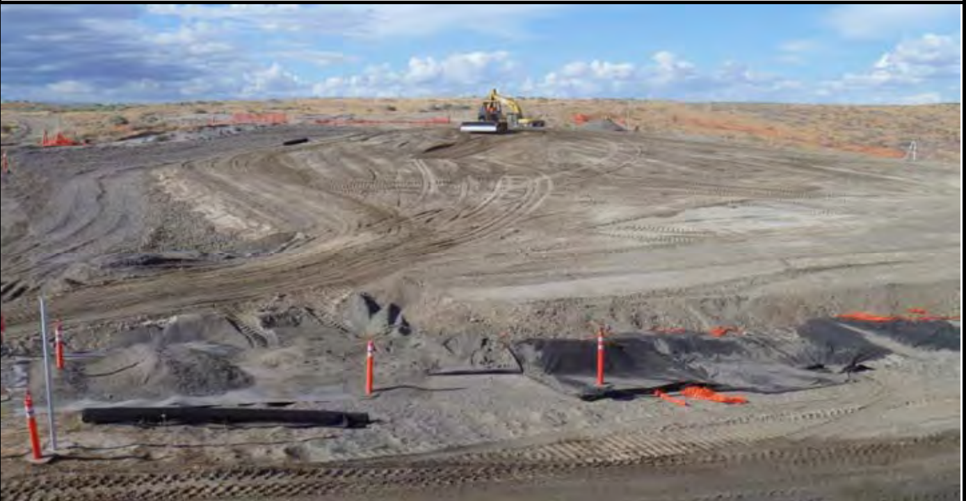
Photo 4: View of the western and northwestern swales (with perimeter rock installed) and top of the western side of the CAP after surface grading. View looking north from point just SW of the SW corner of the EOL.
