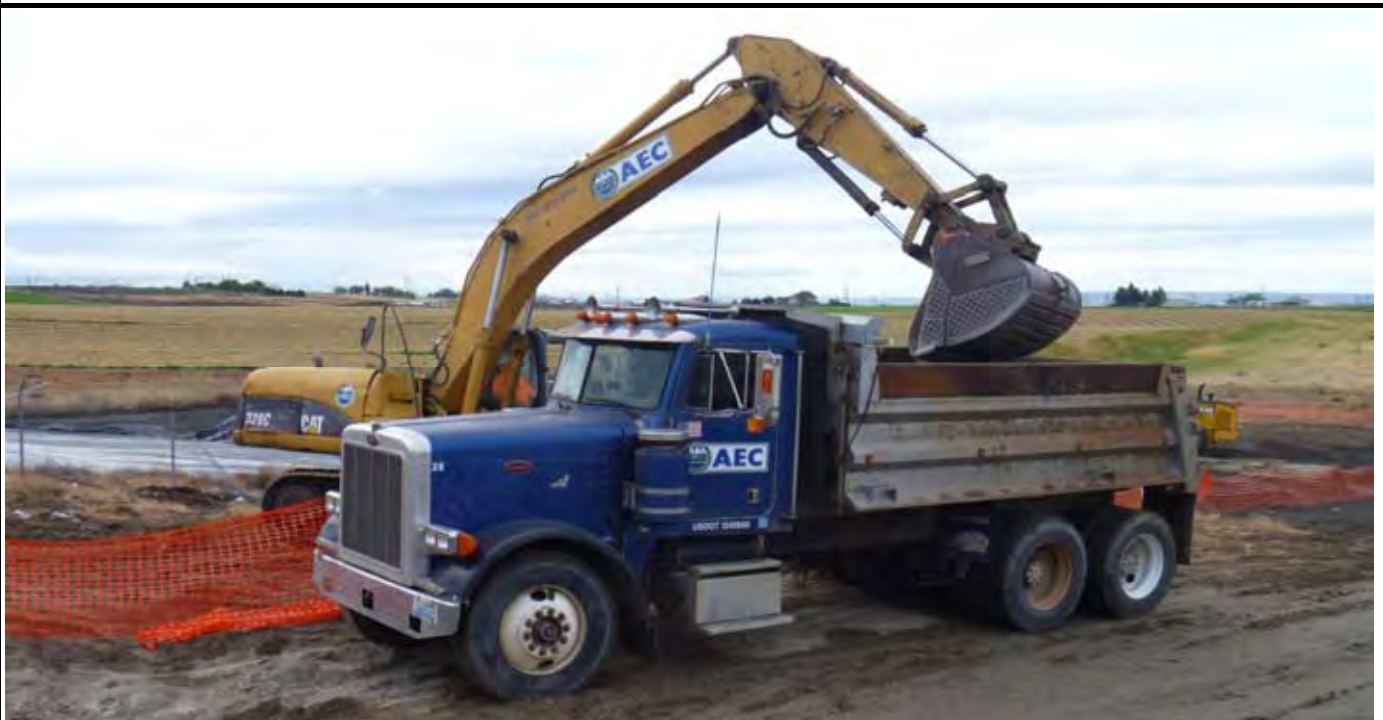
Photo 2: View of AEC loading cyclone fencing for scrap metal recycling.
