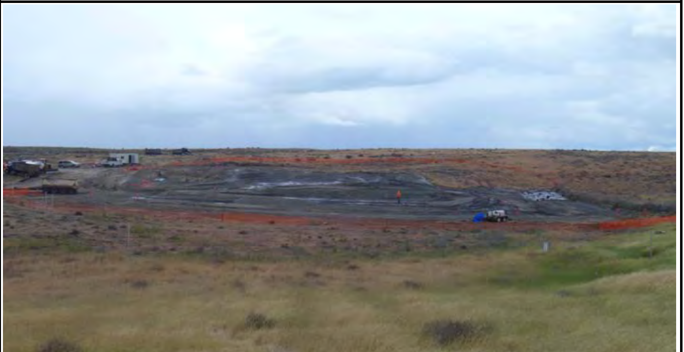
Photo 6: View of the site from the end of the day. Note that almost all of the original cap liner is cover (except for small area on NE corner) with G-layer gravel. View looking north from area beyond southern end of site.
