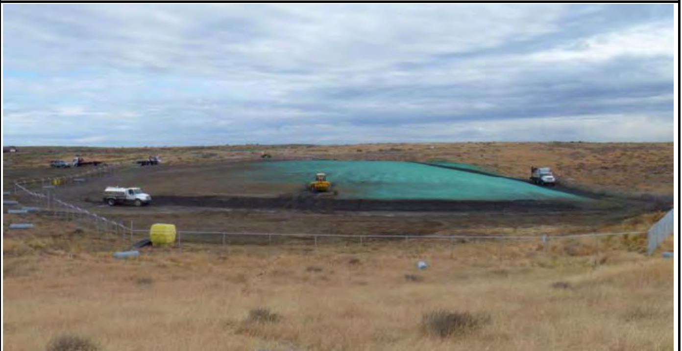
Photo 4: View of Wildlands hydroseeding the eastern half of the CAP surface from the eastern perimeter access road (erosion protection rock road). View of the entire CAP from area south of the site.
