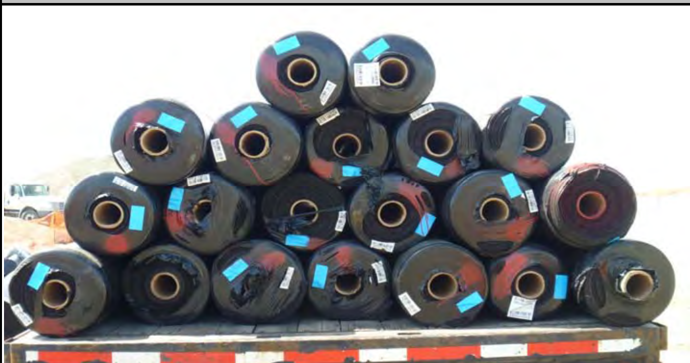
Photo 7: View of the ends of the 20 geosynthetic rolls (barrier between sand and topsoil layers) on delivery truck. View looking west from area near SW corner of the CAP.
