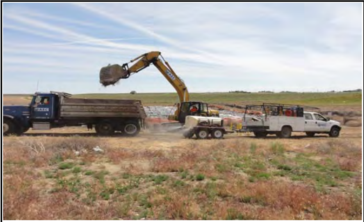
Photo 3: Water trailer spraying water on the site roadway. Loading grubbing debris (tumbleweeds) into dump truck for off-site disposal at adjacent transfer station. View looking east.
