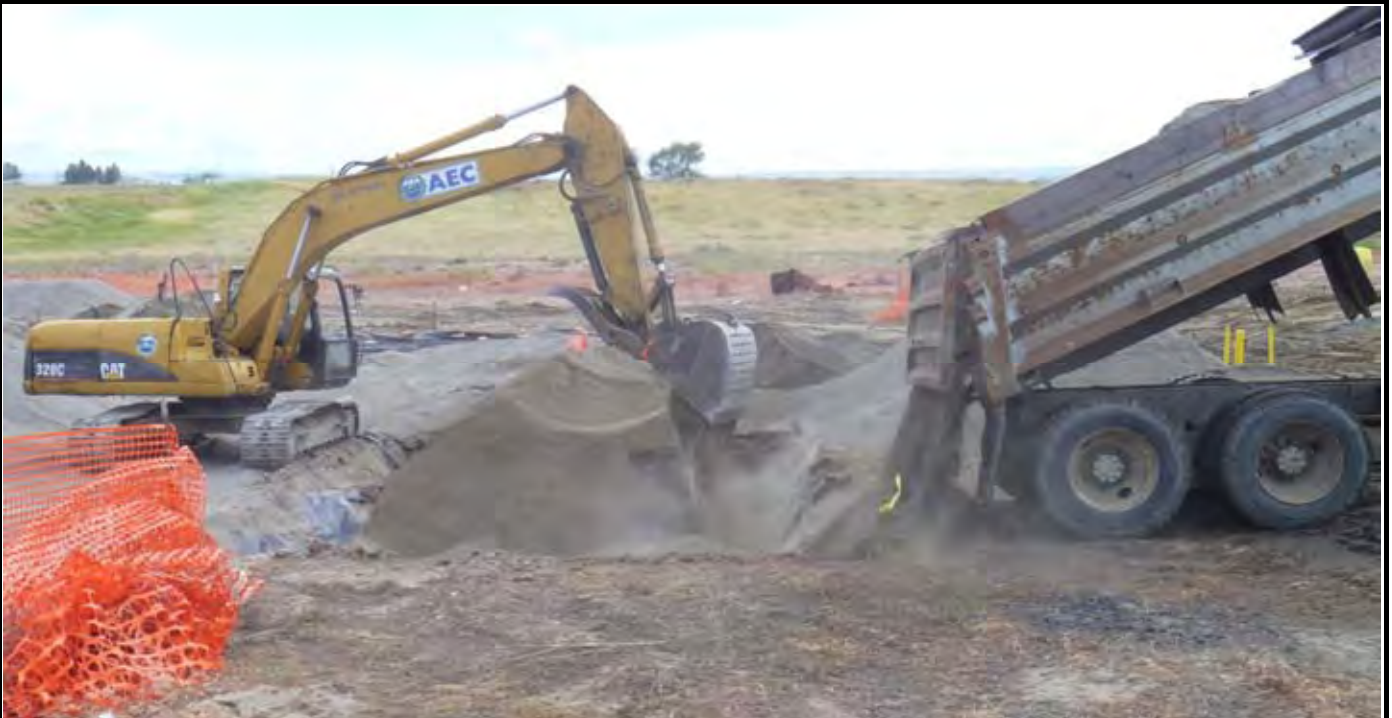
Photo 8: View of AE-2 getting backfilled with gravel with trackhoe and load from AEC dump truck. View looking south from the north side of AE-2.
