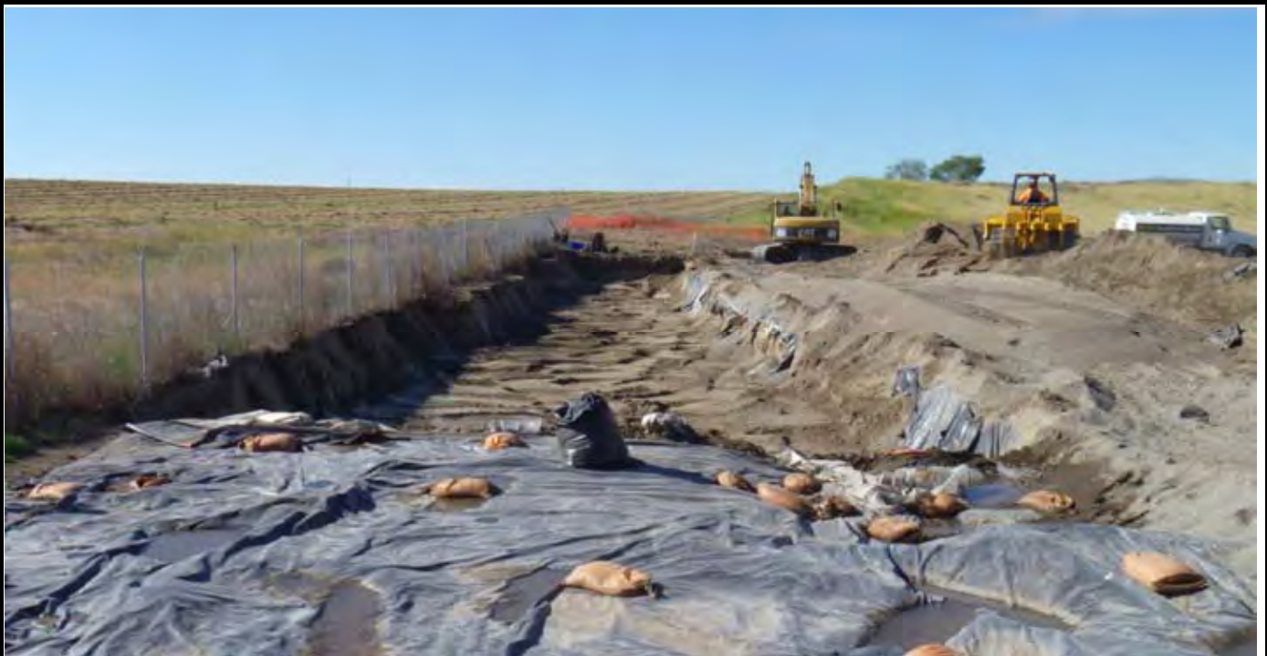
Photo 3: View of AE-4 after AEC completes excavating down to 4-ft bgs. View looking to the south across the excavation of AE-4.
