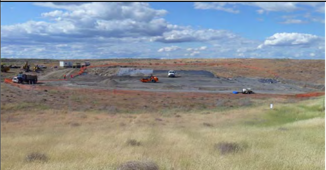
Photo 6: View of the site at the end of the work day. Note that the entire "hump" is covered with G layer gravel and parts of original cap liner and Old GCL is also covered. G layer gravel is stockpiled for the next morning. View looking to the north from the south side of the site.
