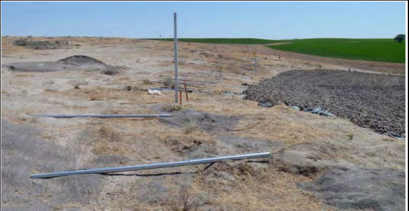
Photo 7: View of the fence posts staged along the northern side of the CAP zone perimeter. View looking east from the NW corner of the CAP perimeter.
