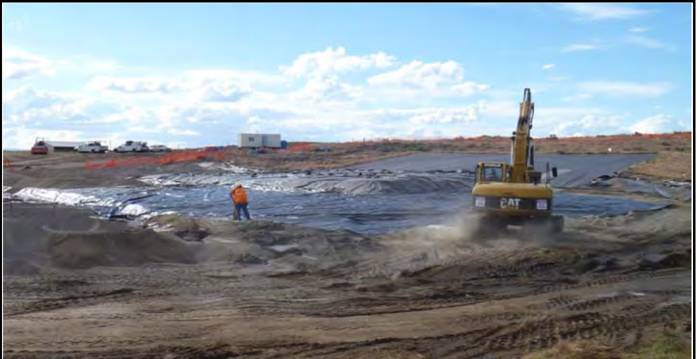
Photo 9: View of the area of soils from AE-4 and AE-5 under the 12-mil plastic liner. Note trackhoe spreading gravel over the cover liner. View looking to the north/northwest.
