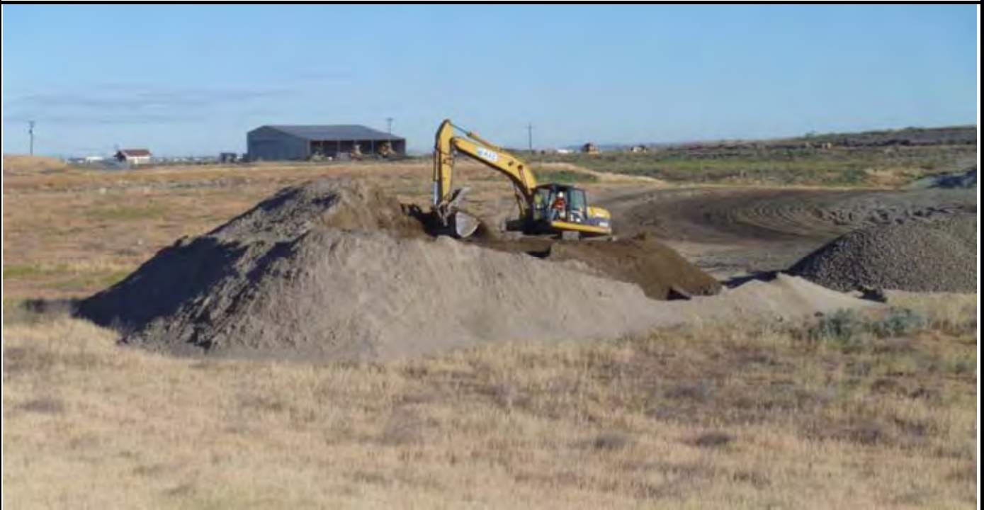
Photo 2: AEC managing the topsoil stockpile. Photo taken near beginning of the work day. View looking NW from area south of the site.
