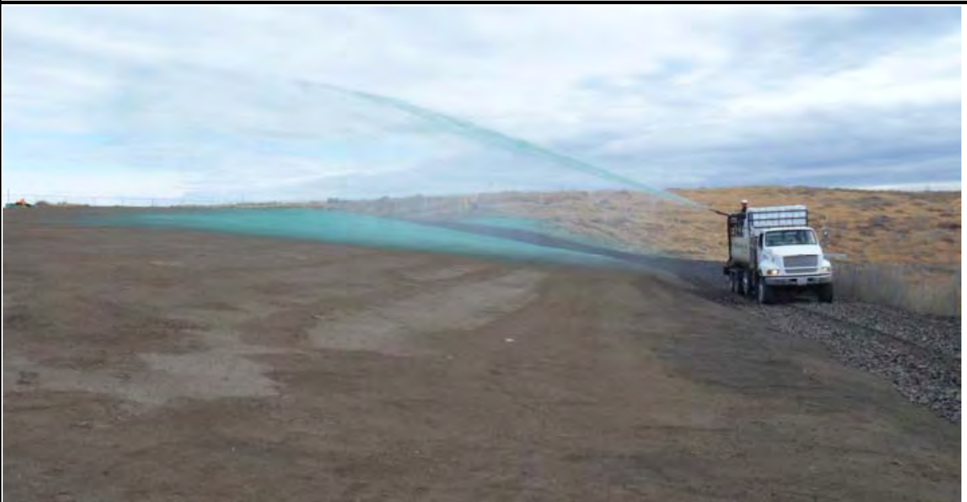
Photo 2: View of Wildlands hydroseeding the eastern half of the CAP surface from the eastern perimeter access road (erosion protection rock road). View of the eastern half of CAP from SE corner of the CAP.
