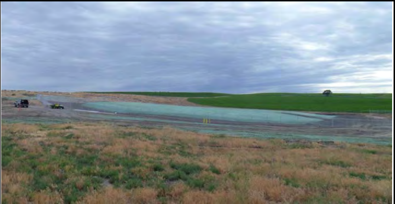
Photo 1: View of the site from the western edge of Zone B. Note the completed hydroseeding and perimeter fencing. View of the CAP from west of the CAP.
