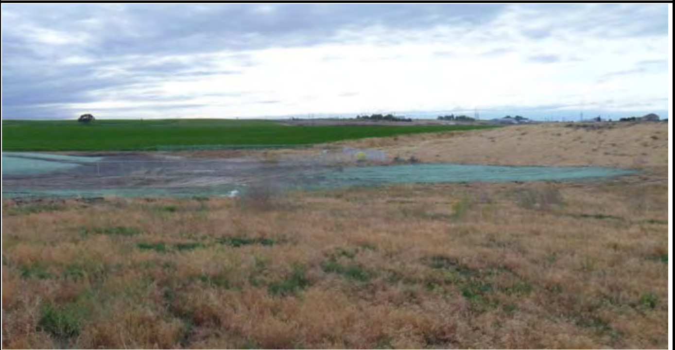
Photo 2: View of the southern portion of the CAP area and disturbed area SW of the perimeter fencing. Note that hydroseeding has been applied to the areas of disturbed soils. View looking east to southeast from west.
