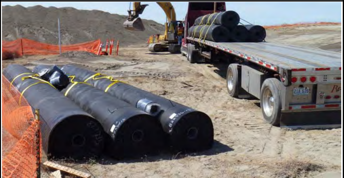
Photo 8: View of the three new rolls of geomembrane liner delivered and stockpiled beyond SW corner of the cap with five rolls of plastic welding cord. View looking NW from the SW corner of the site.
