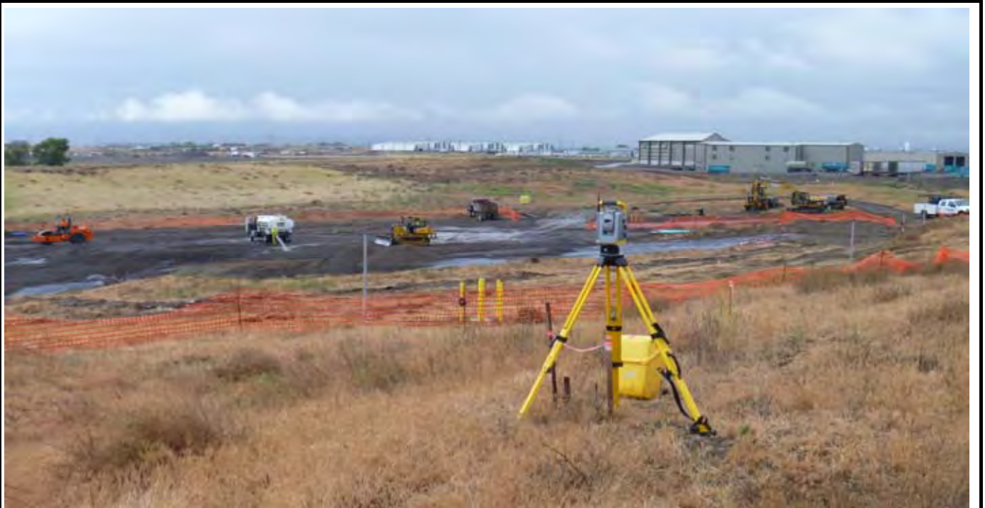
Photo 2: View of the site and AEC's surveyor setting up over northern control point to set out stakes for G-layer grade. View looking south from northern end of site.
