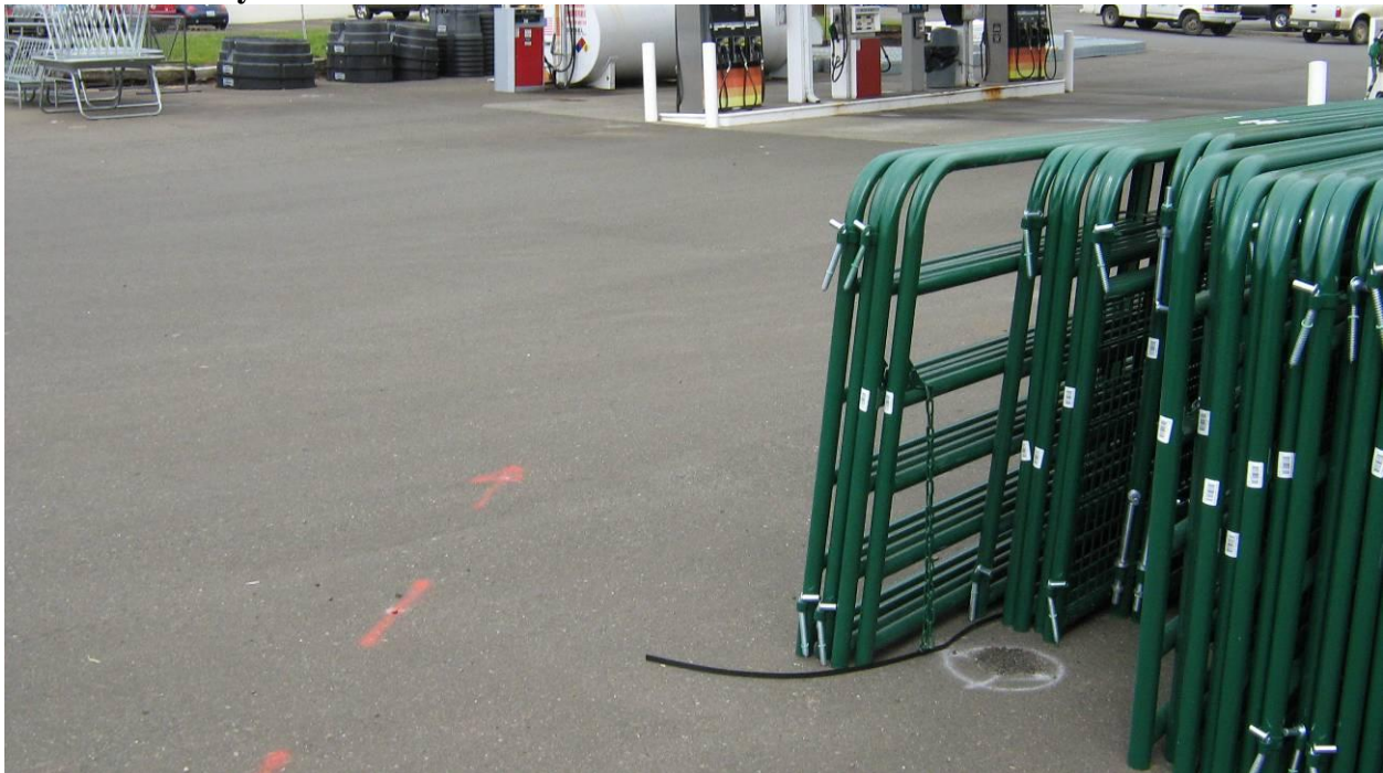
Photo 2: UST System East of Store – from the southwest
